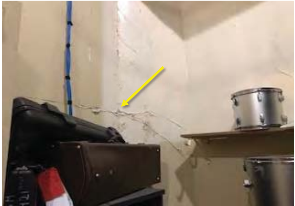
Photograph 5: Multipurpose Building: View of wall water damage in storage room.
