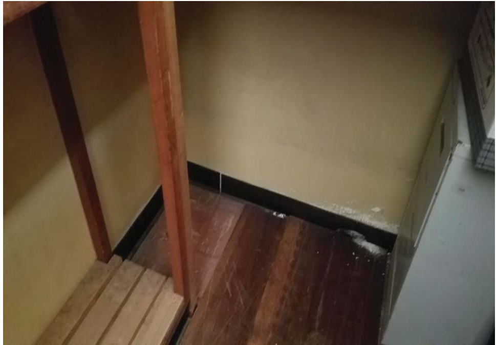
Photograph 11: Multipurpose Building: View of asbestos-containing black cove base in storage room 129.
