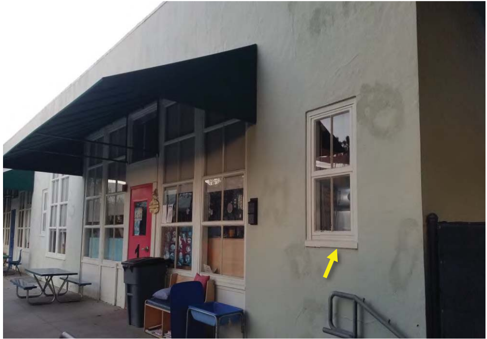
Photograph 5: Classroom Building: View of asbestos-containing window putty at exterior small windows throughout.
