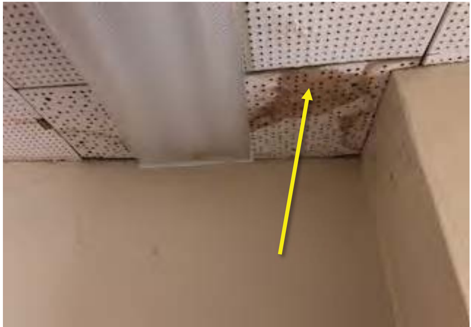
Photograph 4: Multipurpose Building: View of ceiling water damage in hallway areas.
