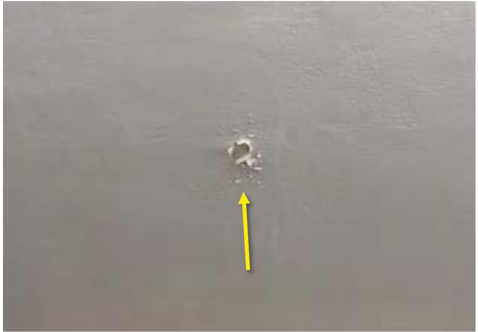
Photograph 1: Classroom Building: View of ceiling water damage in classroom 4.
