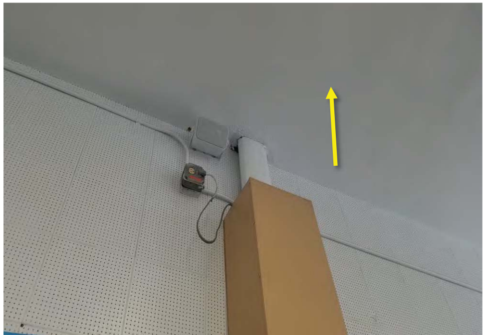
Photograph 2: Classroom Building: View of the asbestos-containing plaster ceilings throughout classrooms 1-4 and restroom.
