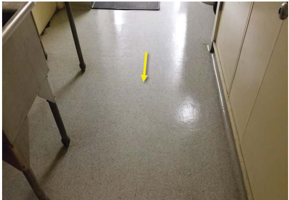
Photograph 10: Multipurpose Building: View of asbestos-containing 9"x9" grayish vinyl floor tile and mastic under vinyl floor sheeting in hallways and break room.
