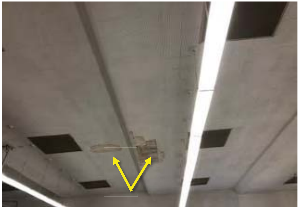
Photograph 2: Multipurpose Building: View of ceiling water damage in the MPR room.
