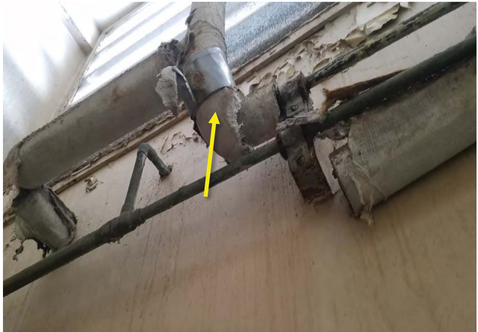
Photograph 6: Multipurpose Building: View of asbestos-containing TSI elbows in poor condition in storage room and throughout attic areas.
