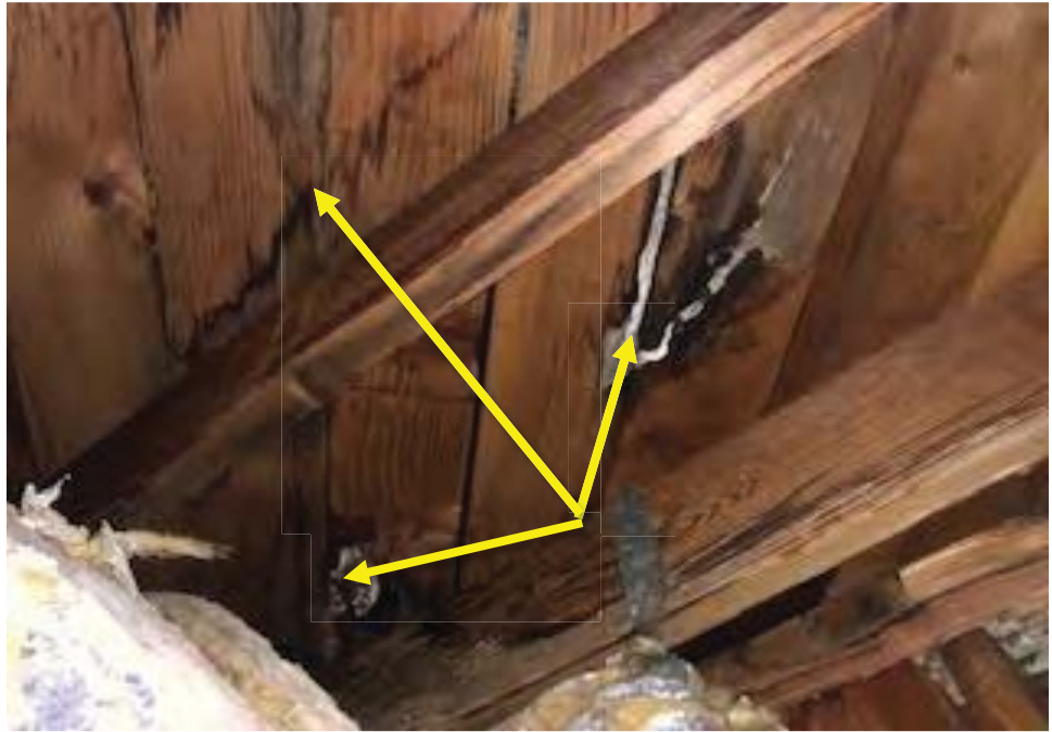
Photograph 3: Multipurpose Building: View of ceiling water damage in the hallway attic areas.
