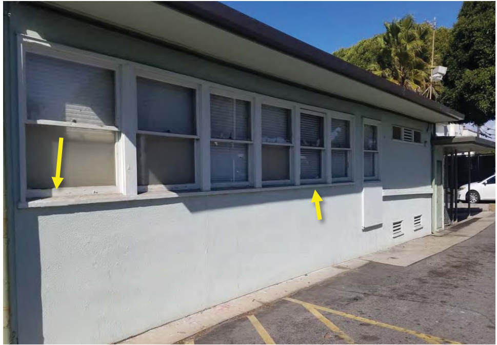
Photograph 15: Multipurpose Building: View of asbestos-containing exterior window putty and asbestos-containing window caulking.
