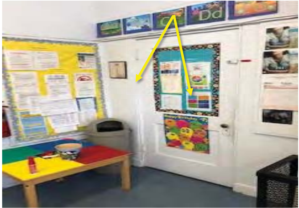
Photograph 3: Classroom Building: View of lead-containing door and door frames.
