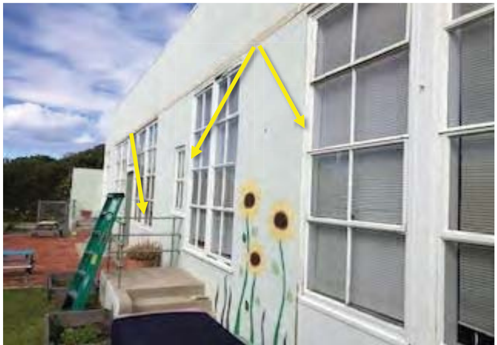
Photograph 2: Classroom Building: View of lead-containing exterior window frames and hand rails.
