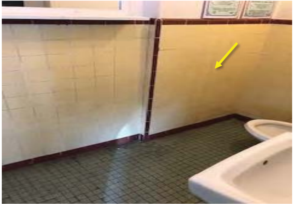
Photograph 17: Multipurpose Building: View of lead-containing ceramic wall tile.
