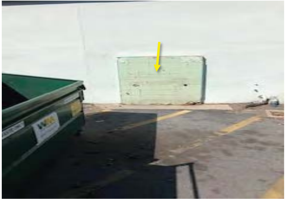
Photograph 13: Multipurpose Building: View lead-containing exterior ceramic wall tile.
