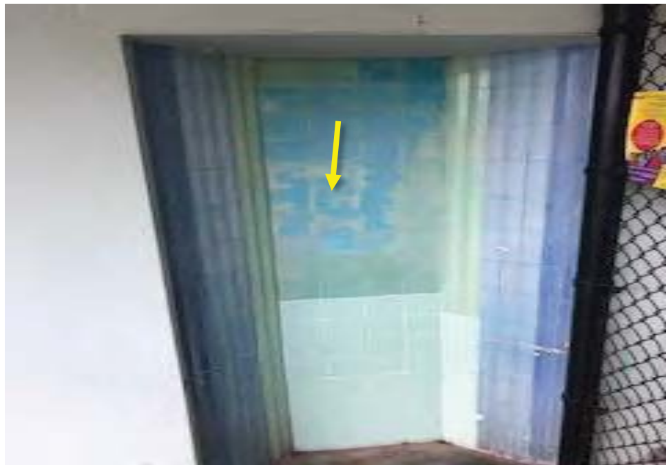
Photograph 10: Classroom Building: View of lead-containing exterior wall tile.
