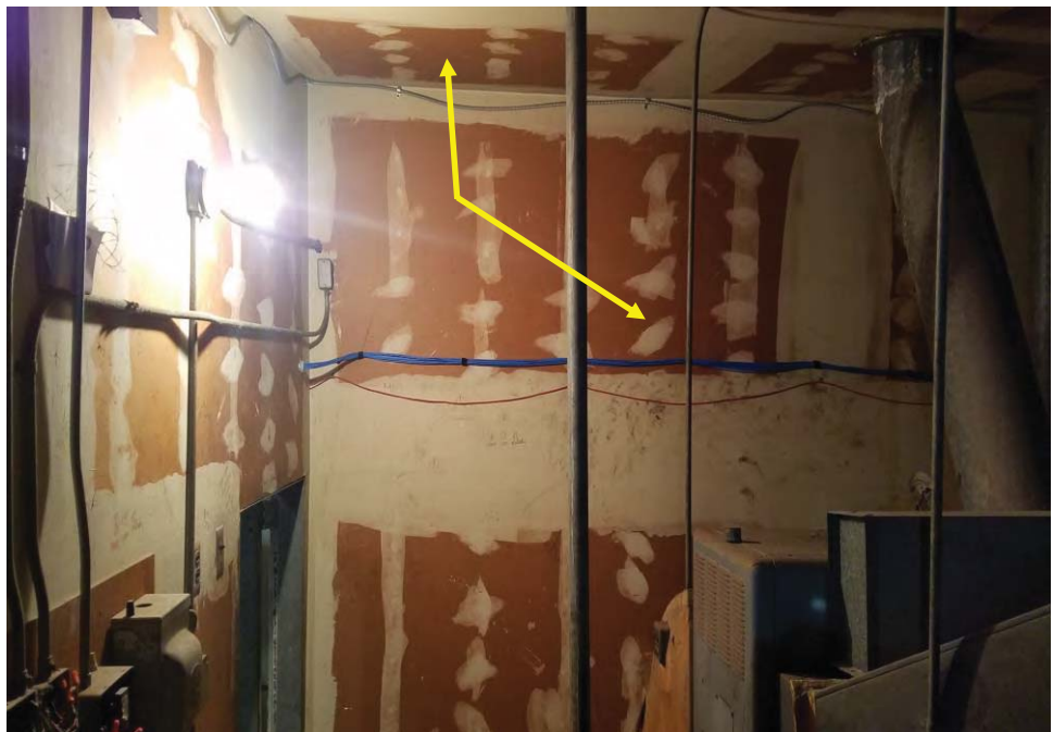
Photograph 14: Multipurpose Building: View of asbestos-containing drywall and joint compound in the mezzanine mechanical room.
