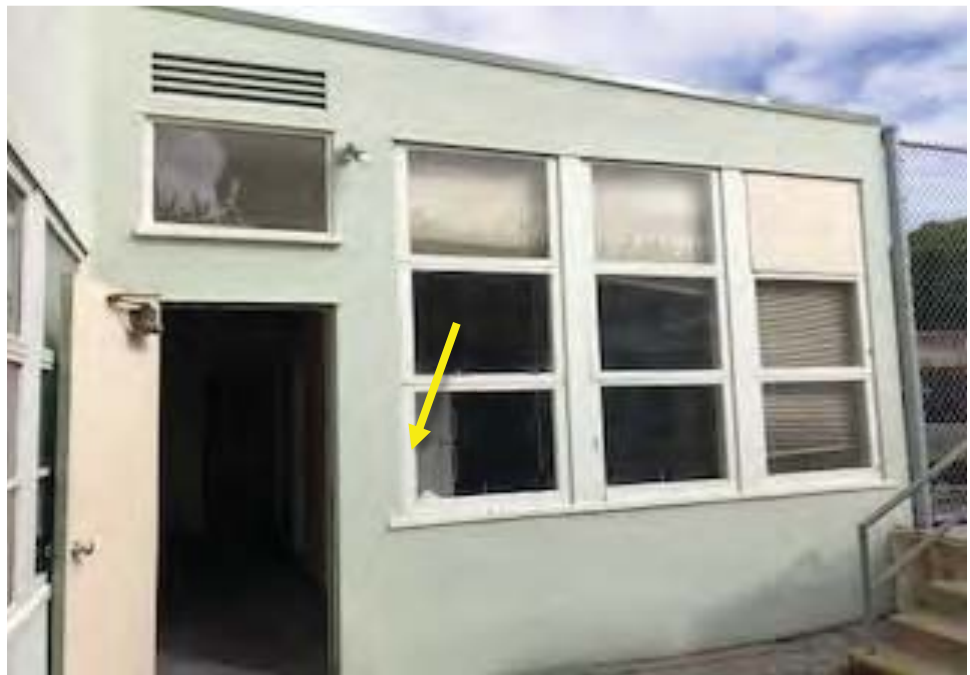
Photograph 12: Multipurpose Building: View of lead-containing exterior window frames.
