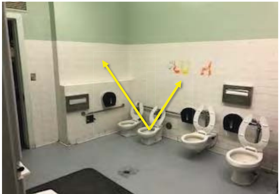
Photograph 4: Classroom Building: View of lead-containing ceramic wall tile.
