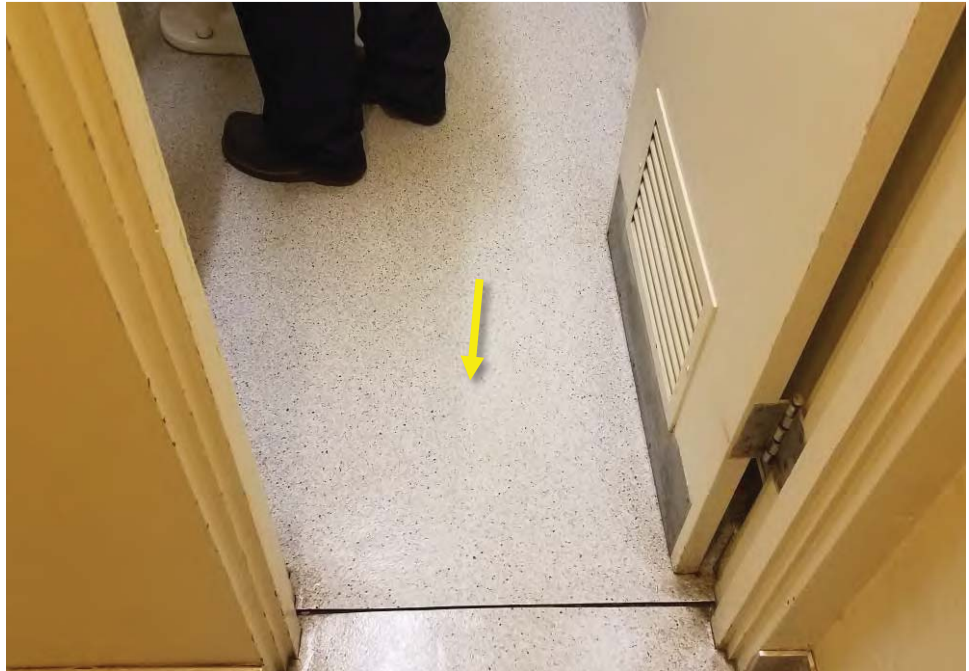
Photograph 13: Multipurpose Building: View of asbestos-containing 9"x9" green vinyl floor tile and mastic under vinyl floor sheeting in small restroom.
