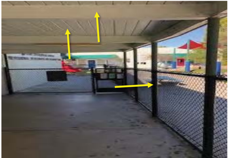
Photograph 14: Multipurpose Building: View of lead-containing beams, posts and decking.
