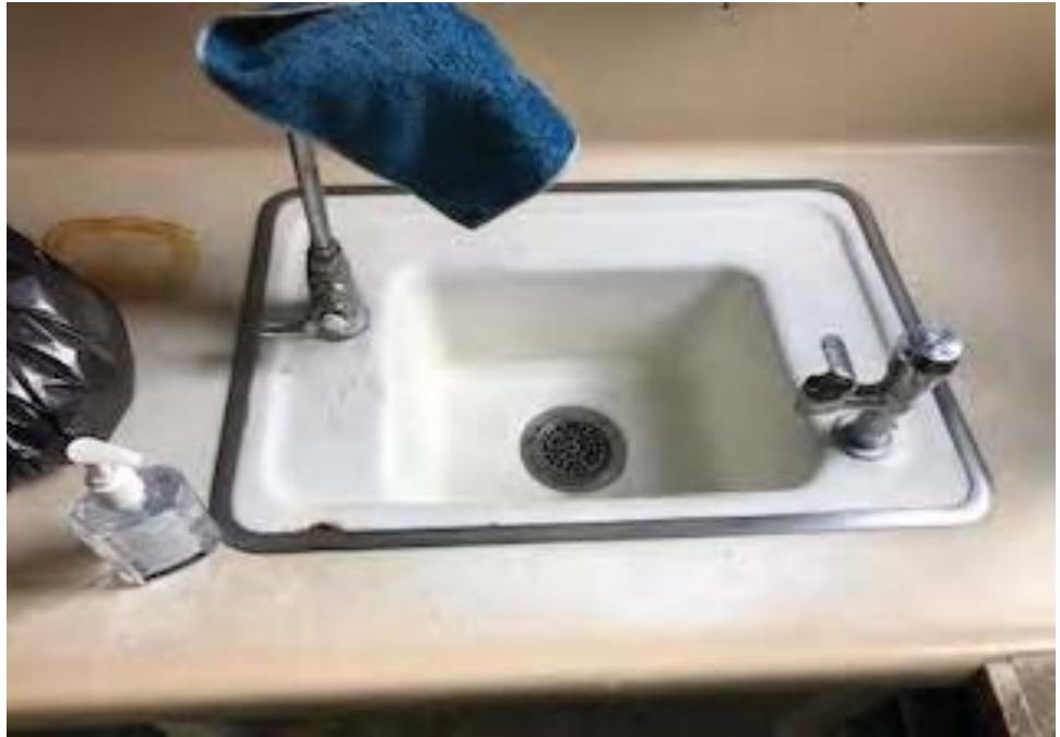
Photograph 1: Classroom Building: View of lead-containing sinks.
