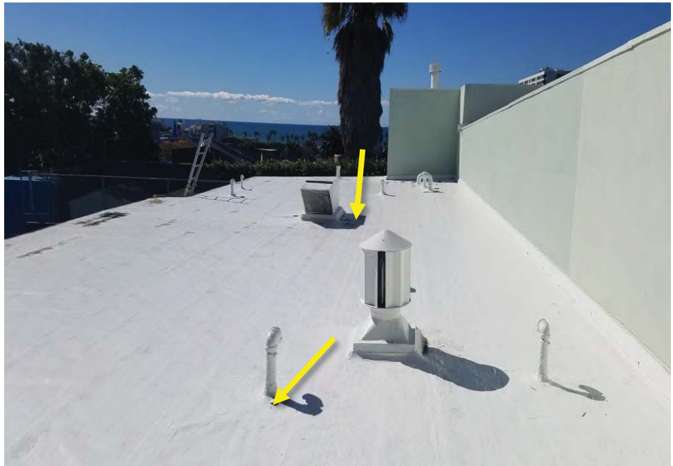
Photograph 16: Multipurpose Building: View of asbestos-containing vinyl rolled roof and roof penetration mastic at library roof areas only.
