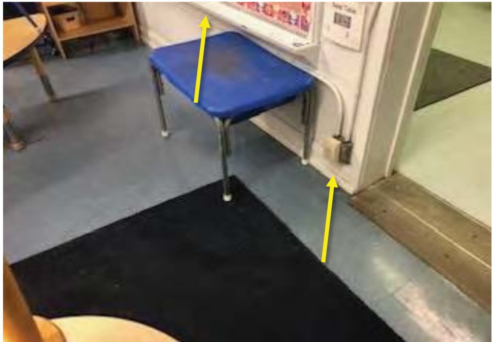
Photograph 6: Classroom Building: View lead-containing chalkboard and base board.
