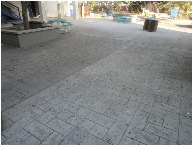
Photo 4: Expansion Joint Caulk, Gray (Exterior walkway)
