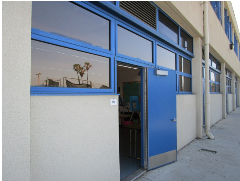
Photo 3: Door Paint, Blue Paint
