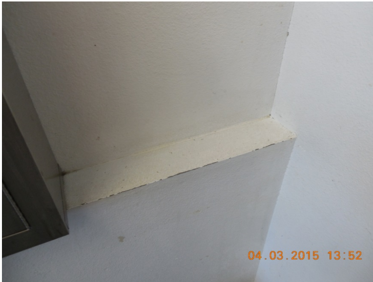
Photo 15: Wall Joint Caulk, White.
