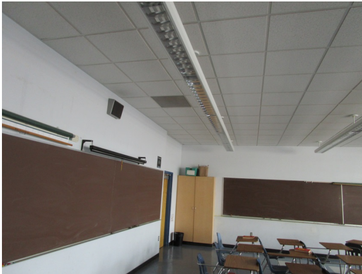
Photo 2: Ceiling Tile, 2'x4' White Painted (2 nd Floor).
