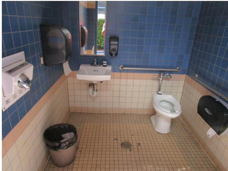
Photo 14: Sink and Toilet Caulk, White. (All Bathrooms)
