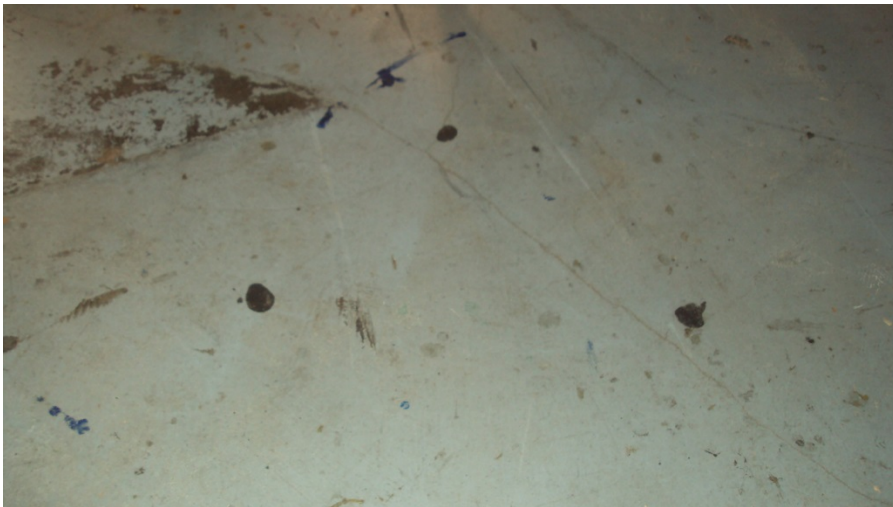
Photo 10: Floor Paint, Gray (Room 105).
