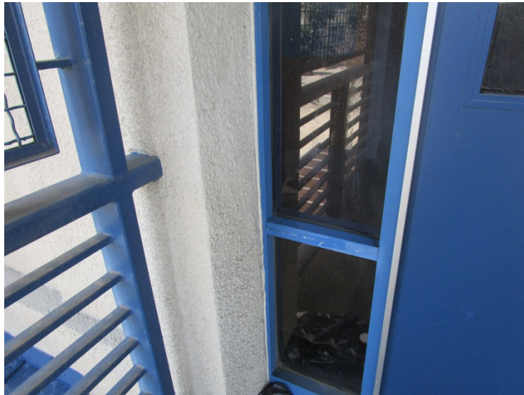
Photo 16: Stucco Painted, Cream abutting White Window Caulk and Black Window Glazing.
