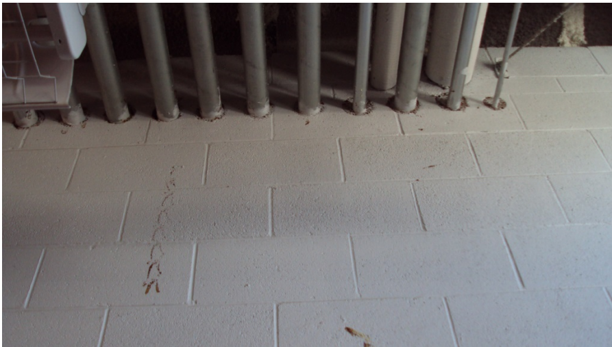
Photo 8: Fire Stop Caulk (Room 105).
