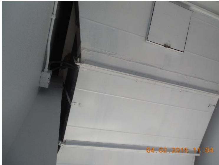
Photo 18: HVAC Caulk/Sealant (Mechanical Room).
