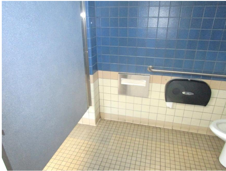
Photo 13: Wall Tile - Ceramic, 4"x4" Blue, Tan and White with Tan and Beige 2"x2" Ceramic Floor tiles. (1 st Floor Men & Women Bathrooms; 2 nd Floor both Women Bathrooms )
