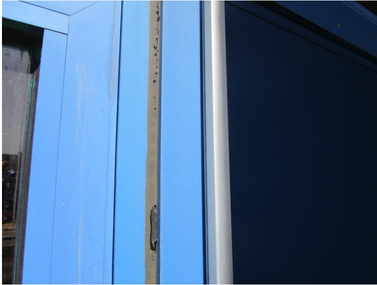
Photo 17: Window Caulk, Black inside Blue Window framed casing (Exterior Room T10).
