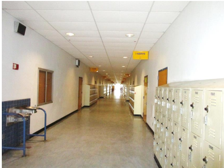
Photo 12: Floor Sheet Vinyl, Blue with Tan Marbled pattern (2 nd Floor only) abutting White Painted Walls and Black Vinyl Cove Base (All Floors).
