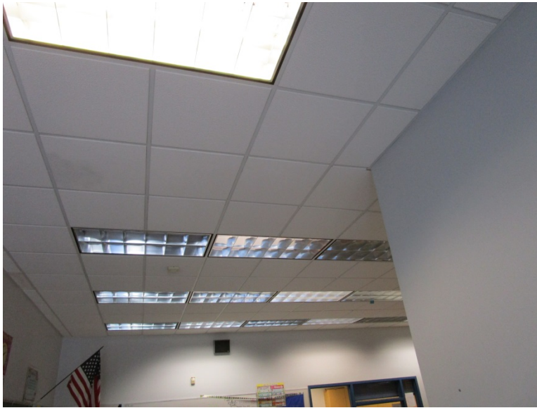
Photo 1: Ceiling Tile, 2'x2' White Painted (1 st Floor).
