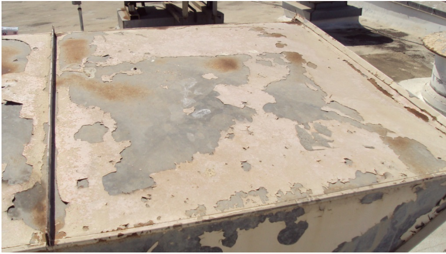
Photo 5: Roof Fan Hood Paint, Beige.
