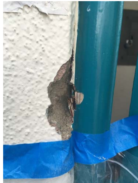
Door D708A-exterior (no visible caulking) Photo 3
