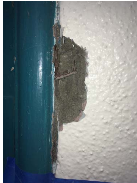
Exterior D708B-exterior (no visible caulking) -Photo 5
