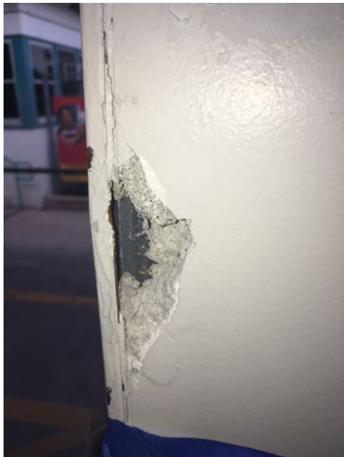
Door D708A-interior (no visible caulking)-Photo 2
