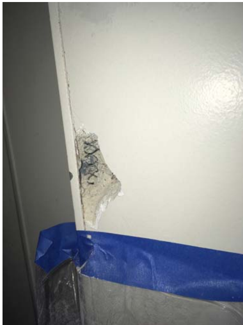
Interior D708B-interior (no visible caulking) -Photo 4
