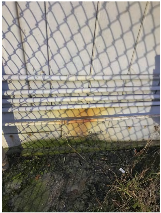
Photo #6: Moisture impact evidence of siding (skirt) under the AHU condensate line
