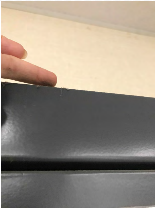
Photo #17: Heavy dust deposition on high horizontal surfaces
