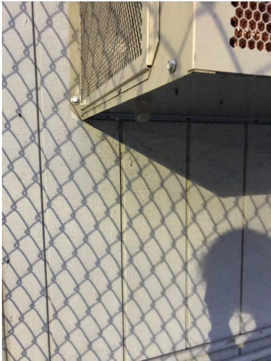
Photo #5: AHU – condensate drain line observed short
