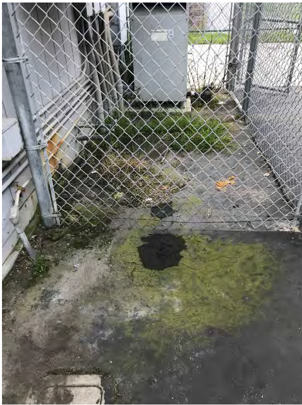
Photo #7: AHU – moss growth observed at the north elevation beneath the AHU
