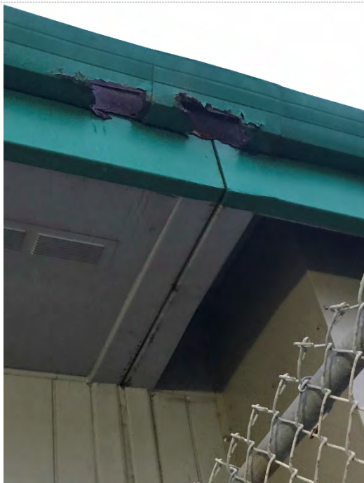
Photo #3: Exterior – rain gutter warped and damaged
