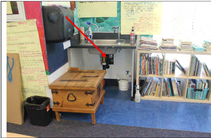
Photo 210: Interior finishes had been removed at two classrooms in building D prior to the DTR site assessment, in an effort to address a leak at this location.
