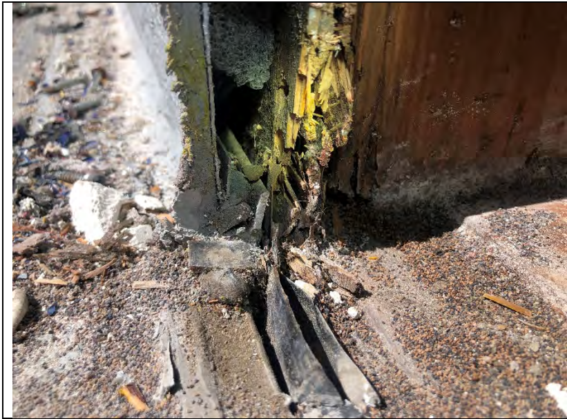
Photo 72: Dry rot and damp wood within the wall assembly.
