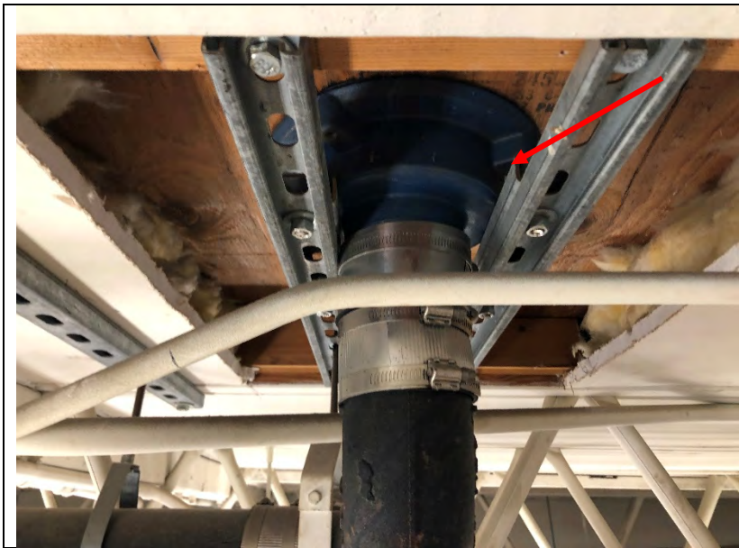
Photo 62: A drain assembly was attached to the bottom of the deck with uni-strut. No anchor bolts were holding the assembly to the deck.
