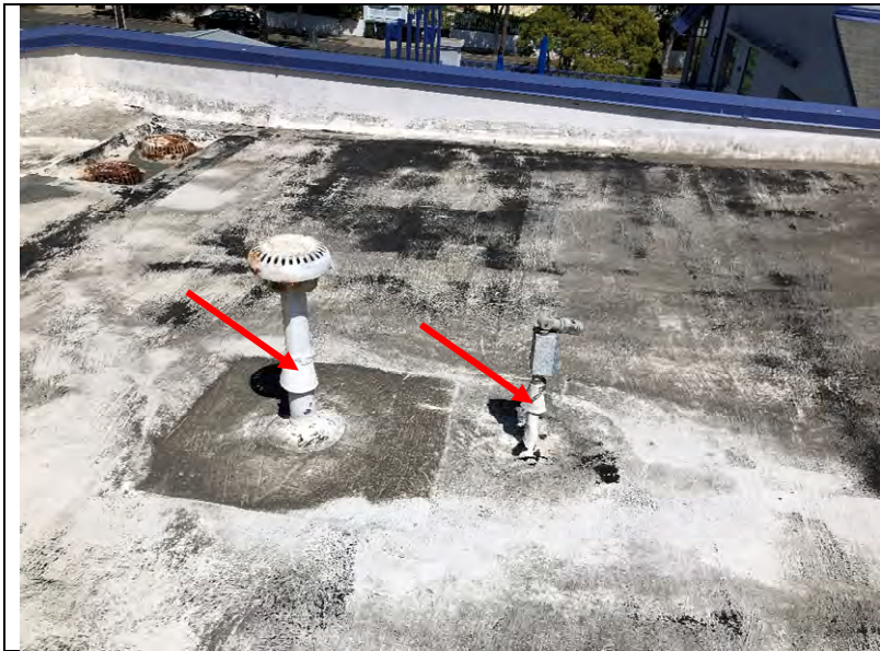
Photo 145: Penetrations with drip guards on the roof of the multipurpose room.
