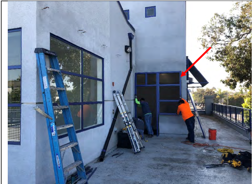
Photo 80: Hollow metal frame were being removed from the west side of building B.
