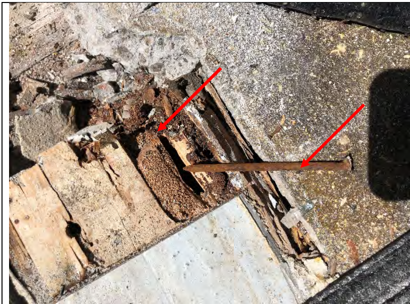
Photo 88: Dry rot, water damage, corroded fasteners, and suspected insect damage at the threshold
