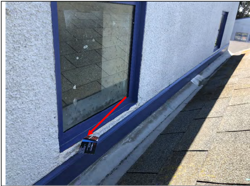
Photo 109: A sealant failure at the perimeter of an aluminum-framed window at roof level.
