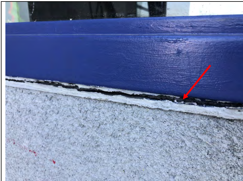
Photo 106: A sealant failure at the perimeter of a hollow metal frame.
