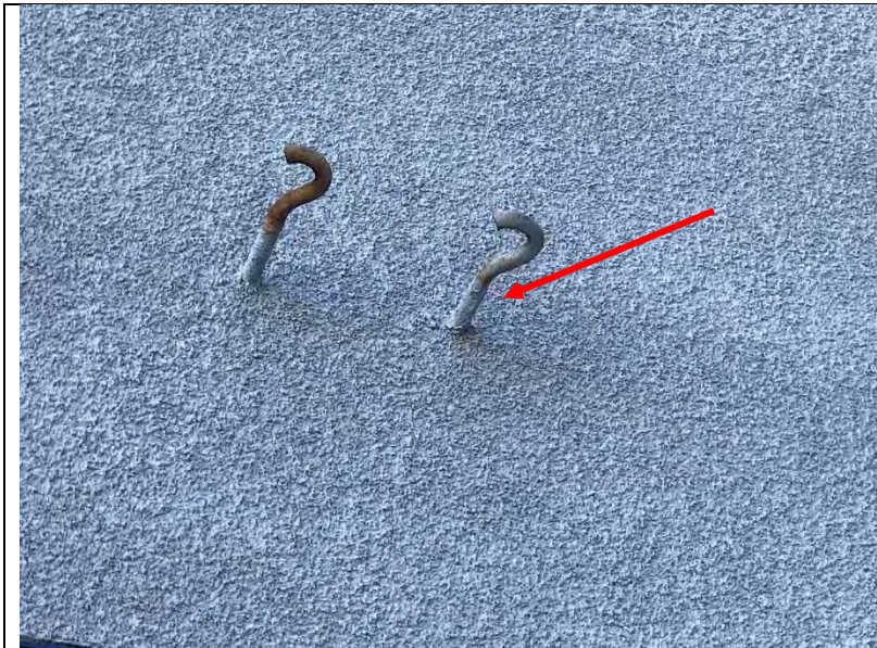
Photo 22: Hook anchor penetration in the cement plaster assembly
