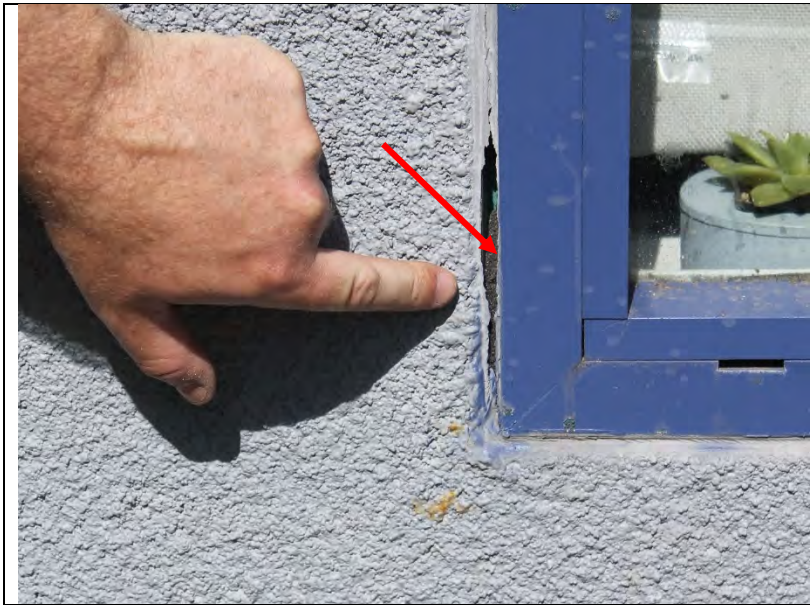
Photo 110: A sealant failure at the perimeter of an aluminum-framed window.
