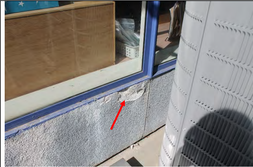
Photo 44: What appears to be salt corrosion of the cement plaster cladding under a window frame on the east side of building D.
