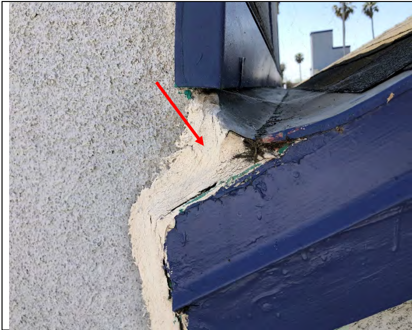
Photo 168: Sealant was observed at the ends of the sheet metal valley
