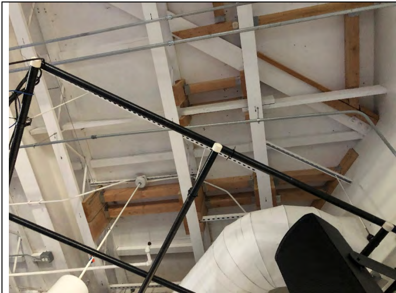
Photo 194: New blocking was installed in the ceiling of the multipurpose room during the HVAC project.
