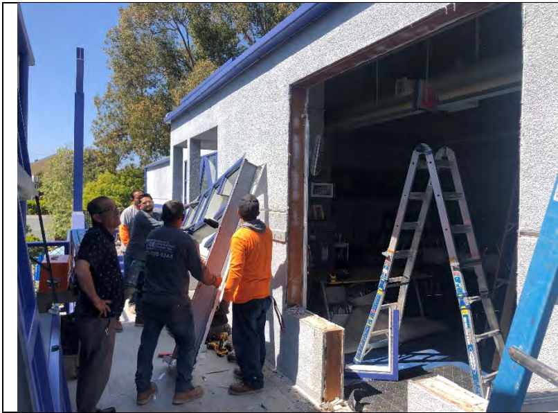
Photo 70: The hollow metal frame after it was fully removed at classroom 480.
