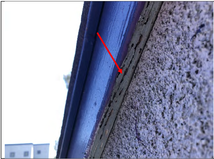
Photo 174: Dry rot and suspected insect damage at the wooden roof trim.
