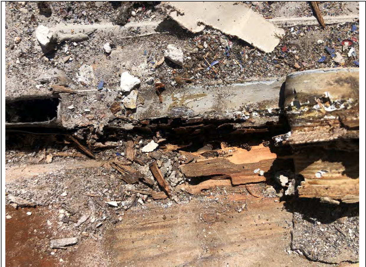
Photo 73: Dry rot, water damage, and suspected insect damage at the threshold of classroom 480
