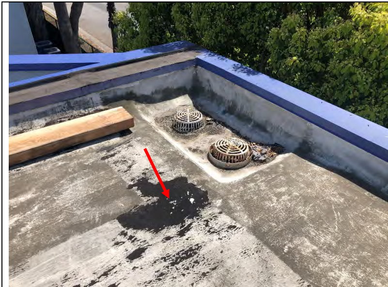
Photo 129: A coating failure at the BUR roof over the multipurpose room.
