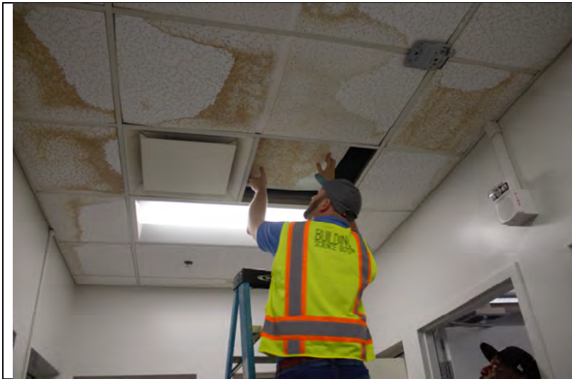
Photo 202: Stained ceiling tiles in room 205 Teacher's Prep.
