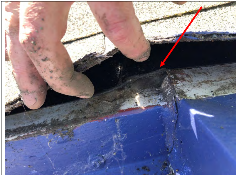
Photo 164: The black peel-and-stick underlayment was not fully adhered at some locations.
