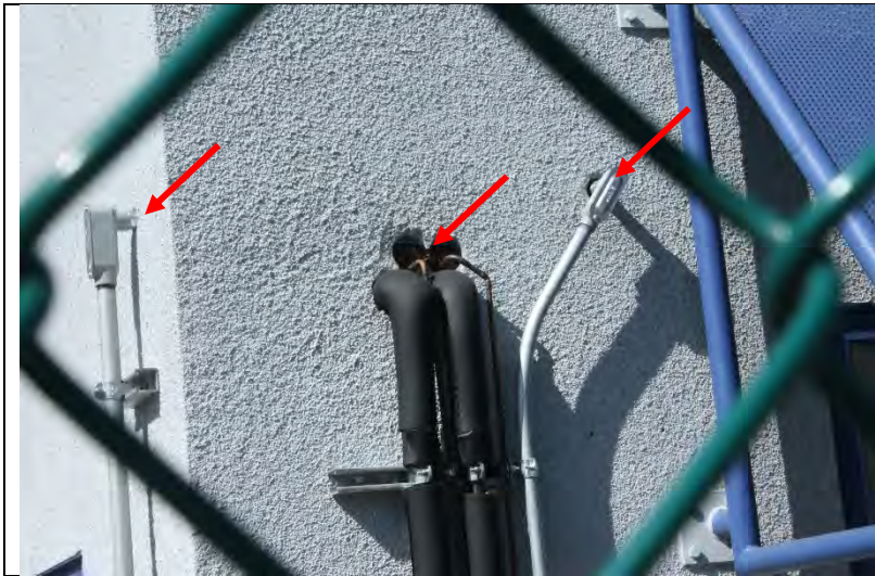
Photo 12: Penetrations in the cement plaster assembly with no visible sealant.
