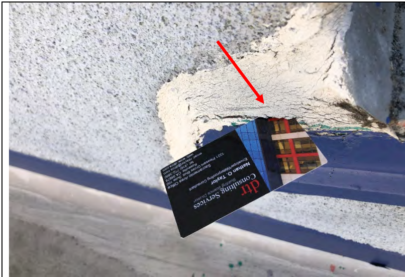
Photo 169: Sealant at the ends of the sheet metal valleys was cracked and had failed in many locations.
