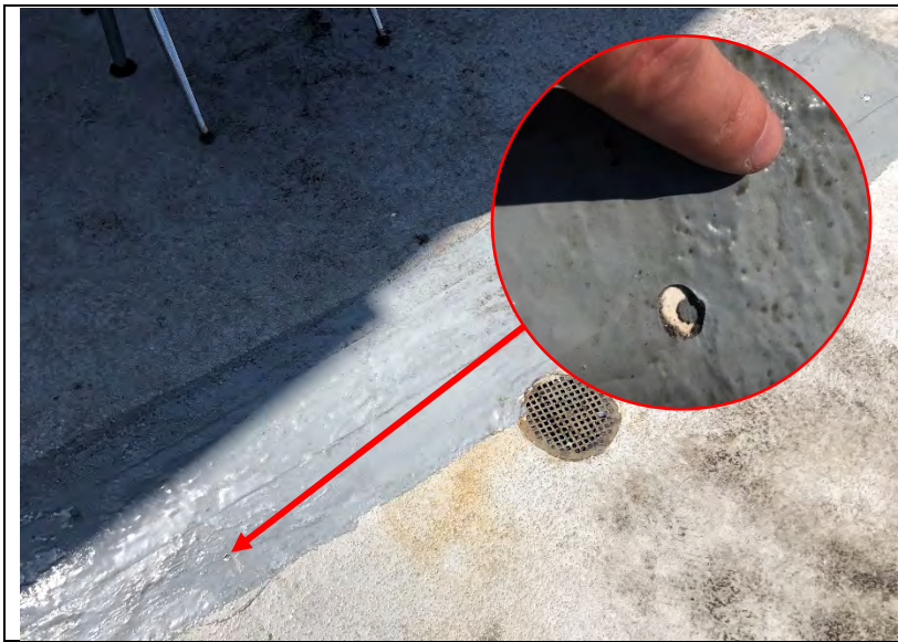
Photo 63: A failure in a traffic coating patch adjacent to a drain test.
