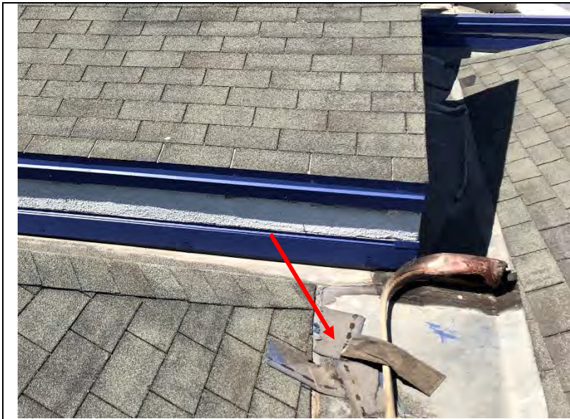
Photo 161: Shingle tabs were observed on the roof deck, at damaged areas on the roof, or were missing altogether.
