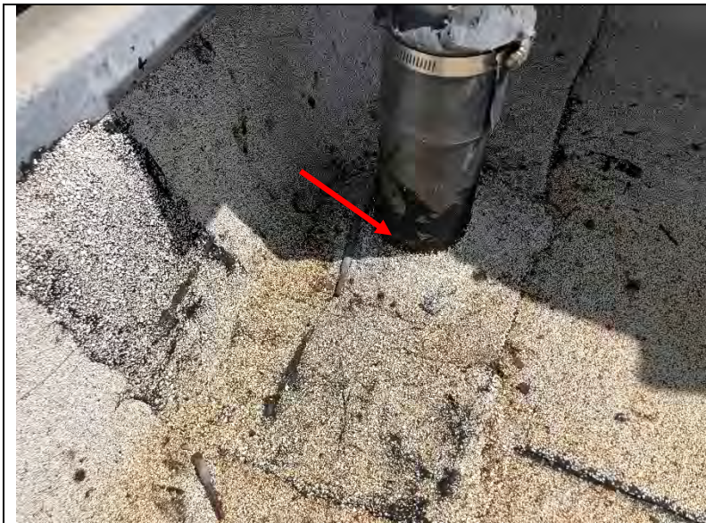
Photo 142: Lead flashings were installed in the newly installed granulated cap sheet on the roof of the multipurpose room.
