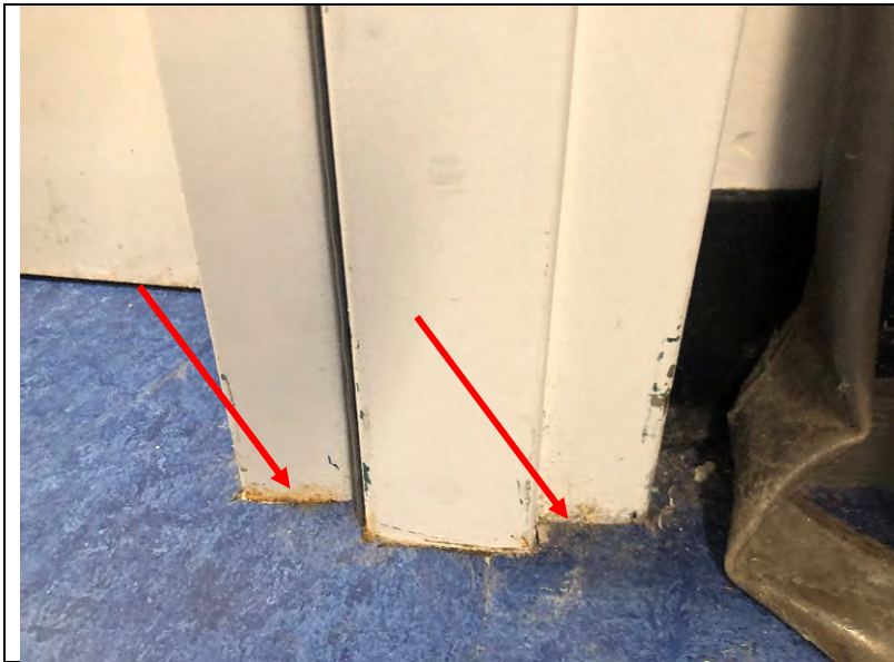
Photo 208: Corrosion at the bottom of the door jamb at Room 403 Teachers' Prep.
