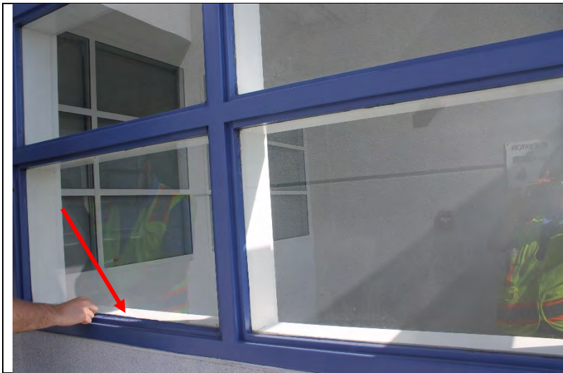
Photo 114: Silicone sealant was applied at the glazing of this hollow-metal framed window.
