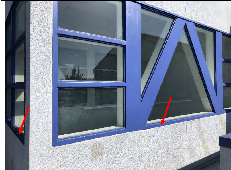
Photo 99: Hollow metal frame assemblies.
