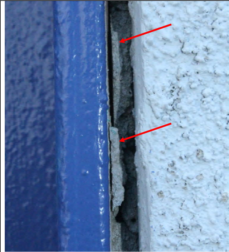
Photo 43: An un-sealed opening in the cladding system where the cement plaster assembly intersects a structural beam.
