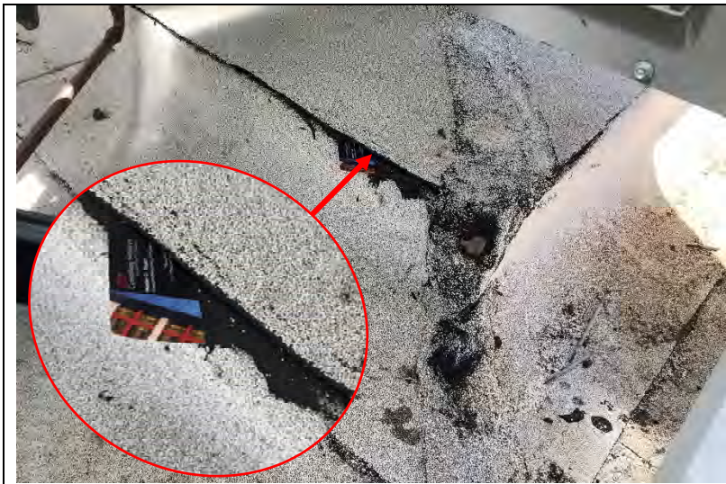
Photo 135: An open seam at the newly installed granulated cap sheet at a mechanical curb.
