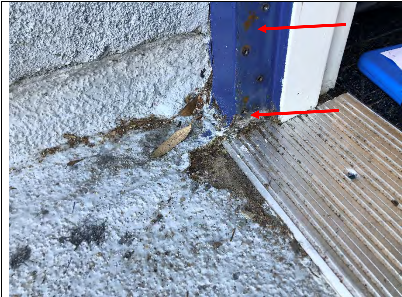
Photo 121: Corrosion damage at the bottom of a door jamb.
