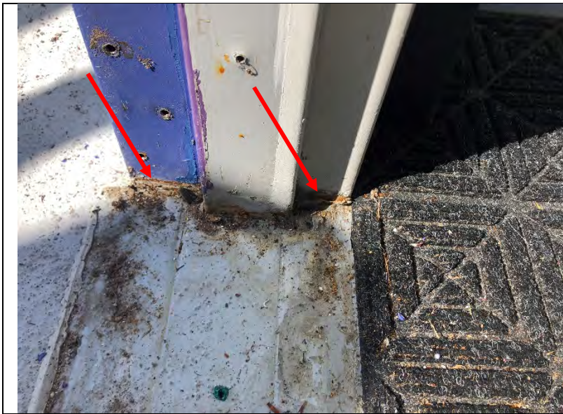
Photo 122: Corrosion damage at the bottom of a door jamb.
