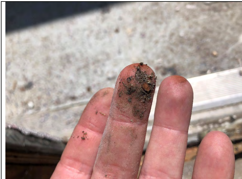
Photo 75: Wood surfaces at the threshold were damp to the touch.
