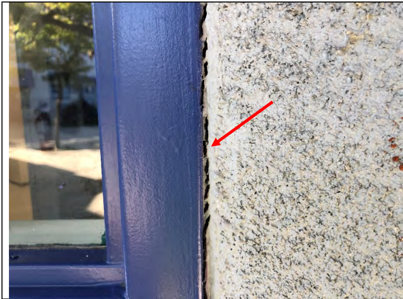
Photo 105: A sealant failure at the perimeter of a hollow metal frame.
