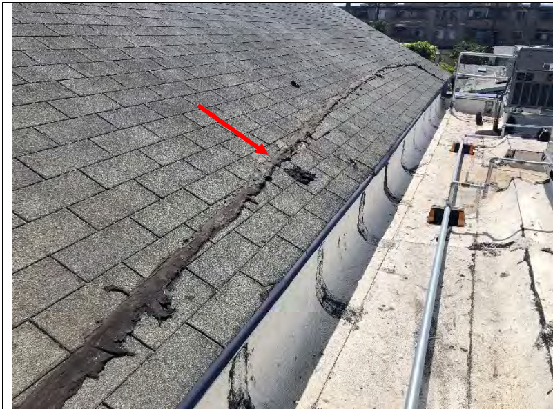
Photo 149: A swath of mastic was observed at the asphalt shingle roofs.
