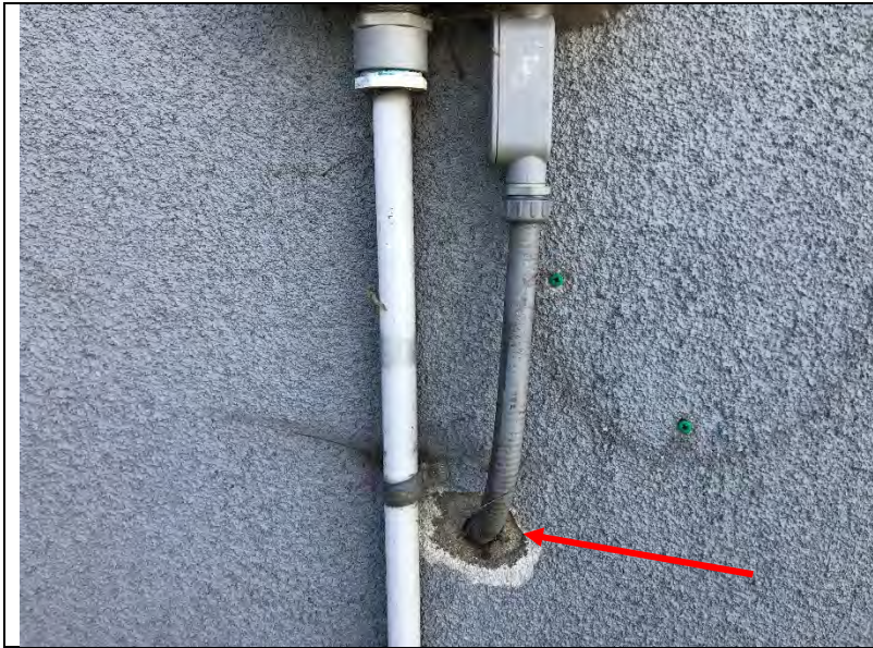
Photo 08: Penetrations in the cement plaster assembly with no visible sealant.
