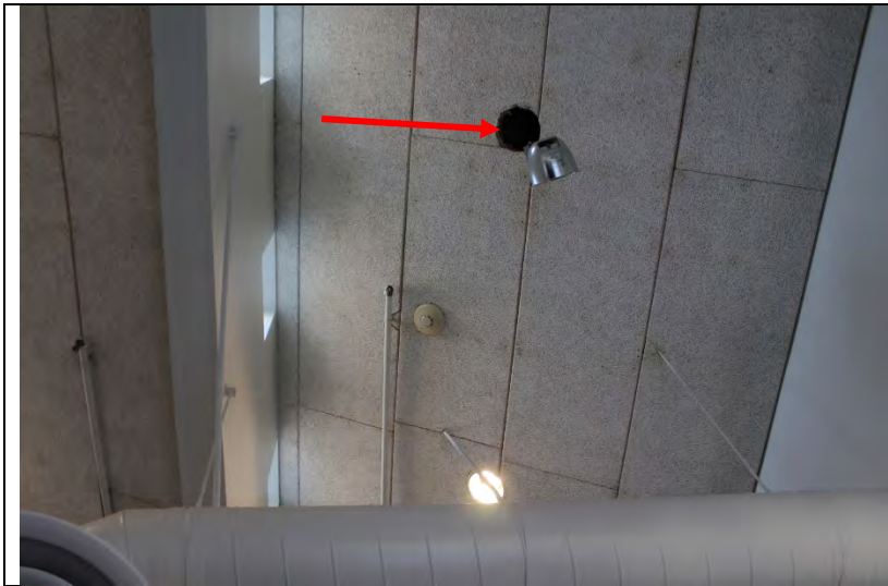
Photo 217: A loose light fixture in the acoustical panels on the ceiling of the classrooms in building D.
