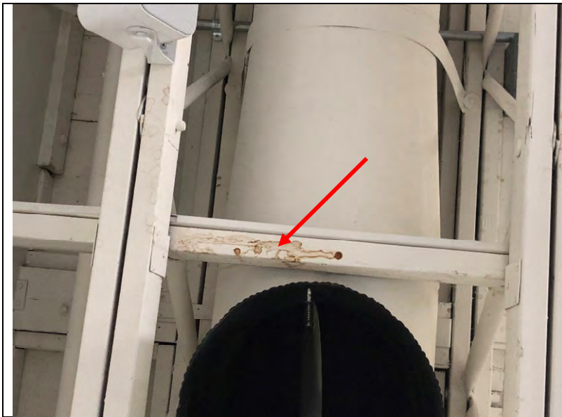
Photo 190: Water stains on the ceiling along the south wall of classroom 415.
