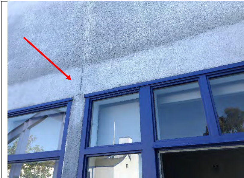
Photo 34: New paint had been applied to the cement plaster above two hollow metal frame assemblies.
