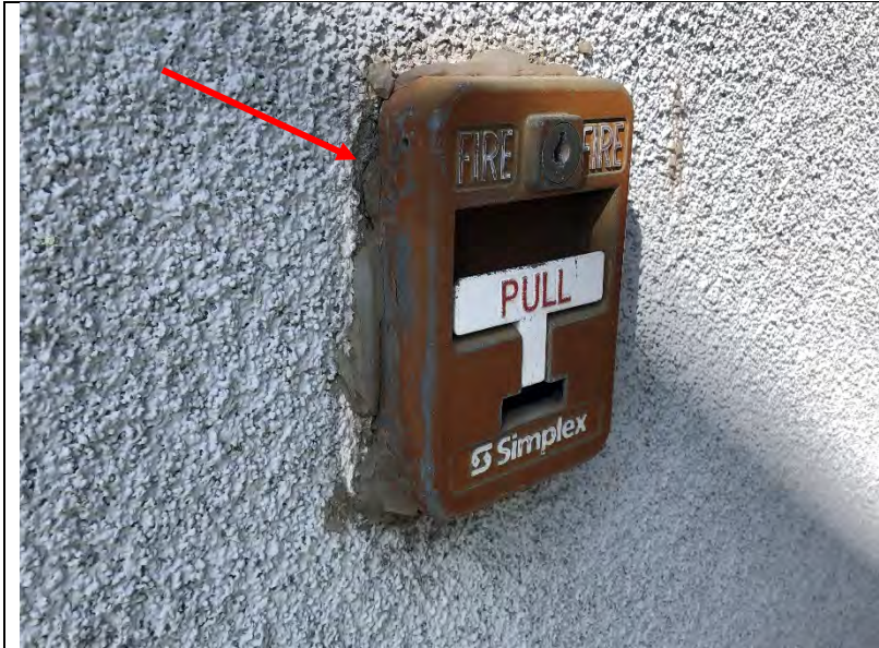
Photo 13: A fire alarm pull penetration in the cement plaster assembly with a failed sealant application.
