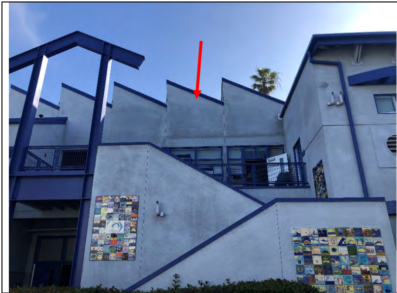
Photo 125: The saw-tooth roof over building D.
