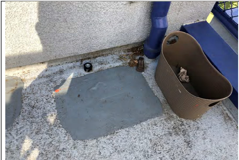
Photo 50: A patch in the traffic coating.
