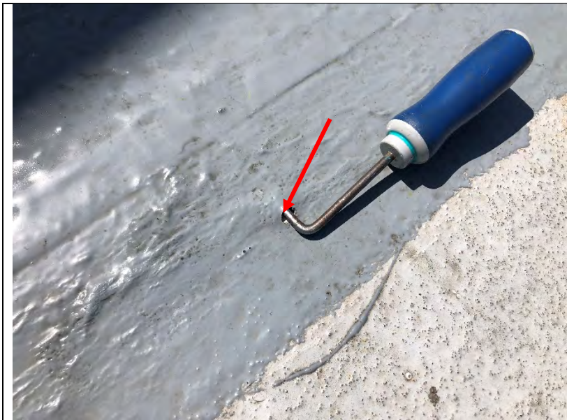
Photo 64: A failure in a traffic coating patch adjacent to a drain test.
