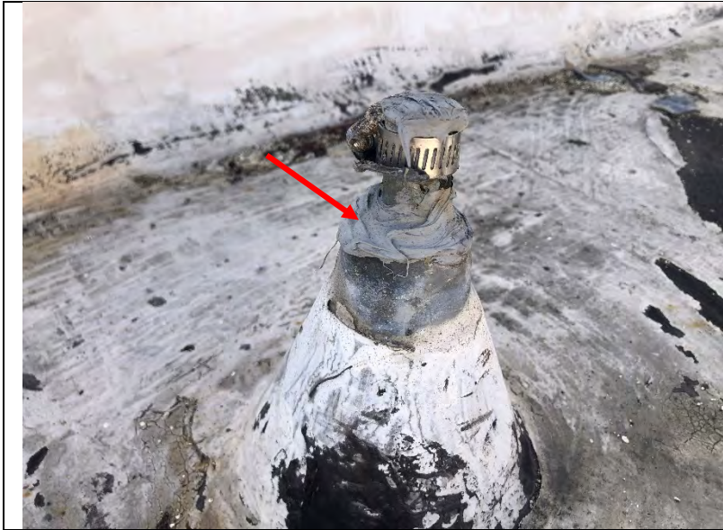
Photo 146: An abandoned conical penetration flashing on the roof of the multipurpose room.
