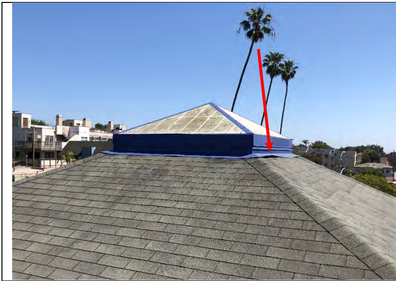
Photo 170: Sheet metal skirt flashing at the skylights was not flat and flush to the roof.
