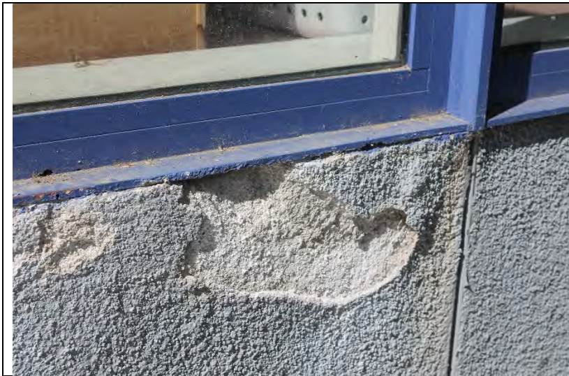
Photo 45: What appears to be salt corrosion of the cement plaster cladding under a window frame on the east side of building D.
