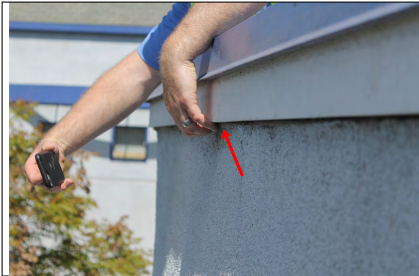
Photo 37: An opening between metal flashing and the top of the cement plaster assembly.
