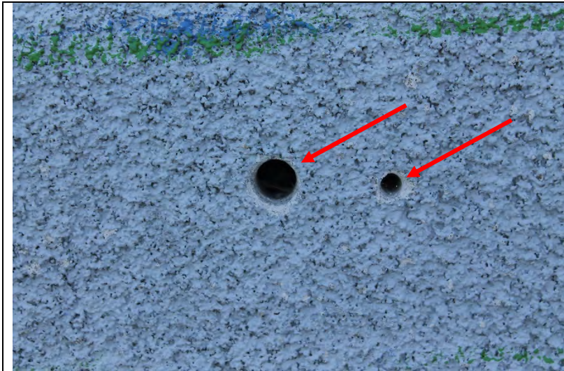
Photo 17: Abandoned penetrations in the cement plaster assembly
