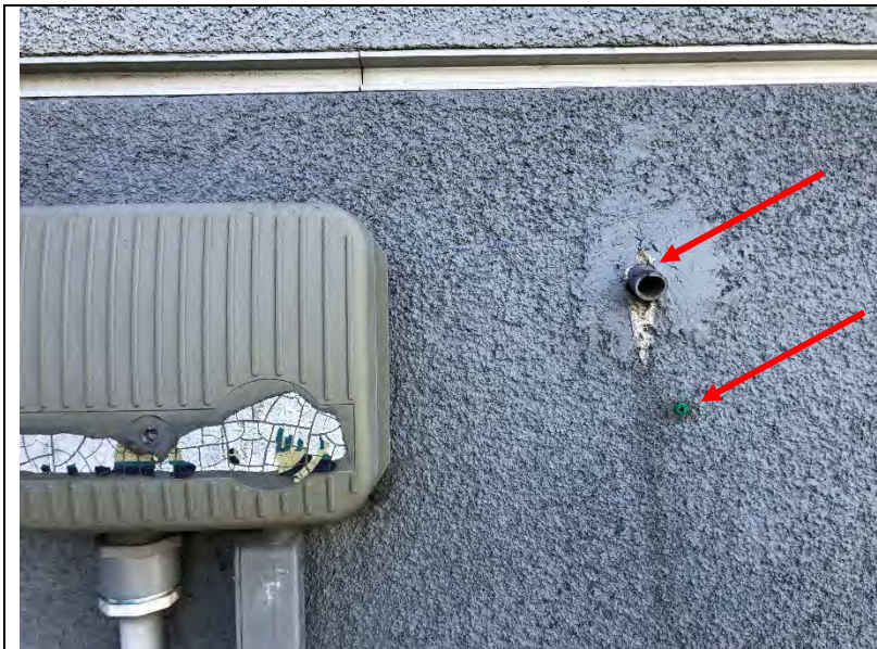
Photo 18: An abandoned penetration in the cement plaster assembly
