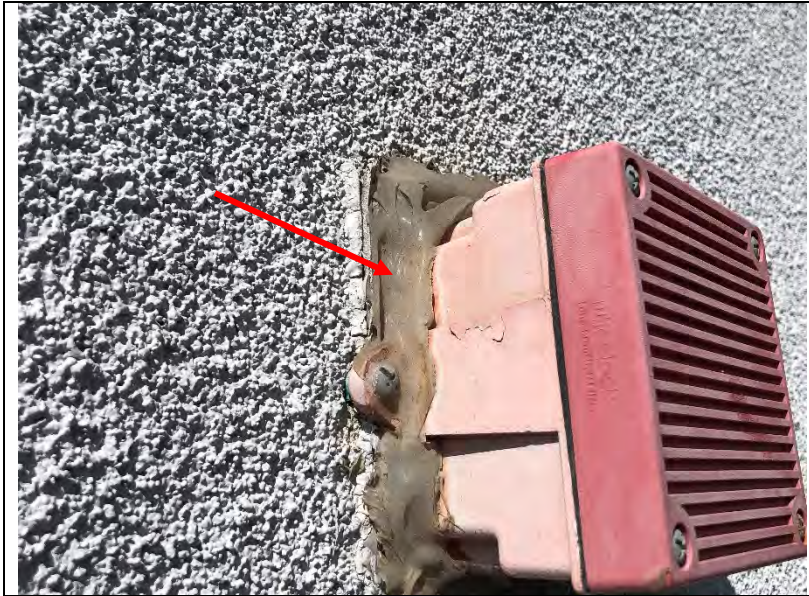
Photo 15: A penetration in the cement plaster assembly with a failed sealant application.
