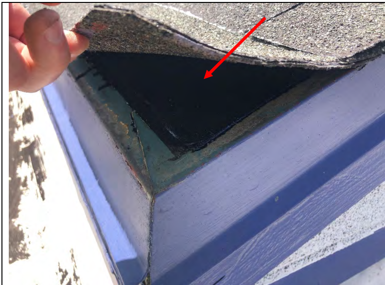
Photo 163: A black peel-and-stick underlayment was present under the asphalt shingle.
