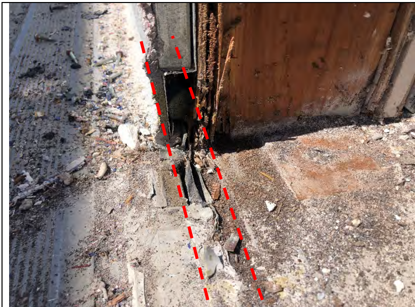
Photo 71: The neoprene water stop at the expansion joint drainage was level with the interior of the cement plaster assembly. This does not conform to the 2001 drawing set (see fig 02)
