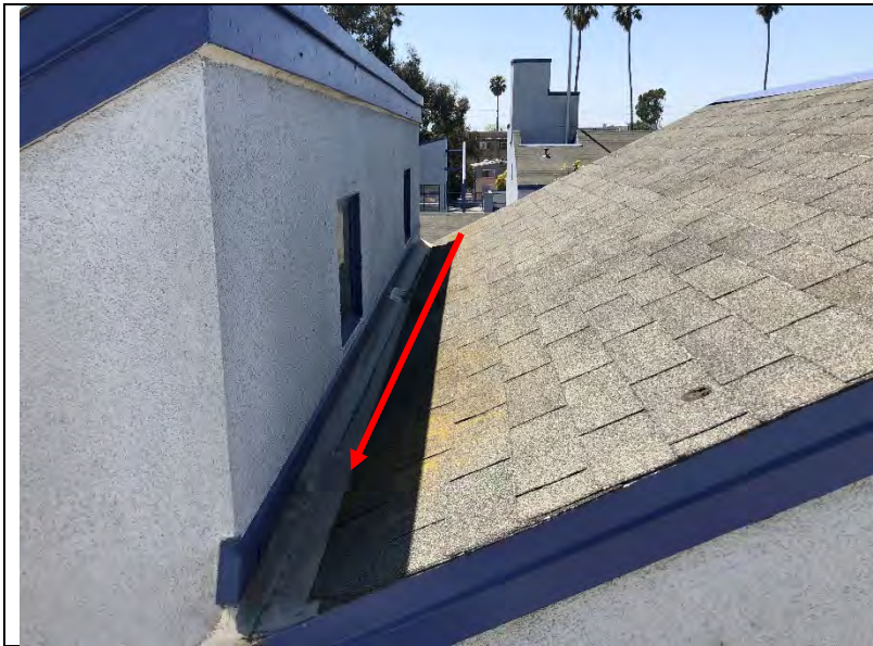
Photo 165: Sheet metal flashing on the asphalt shingle roofs showed various signs of age degradation.
