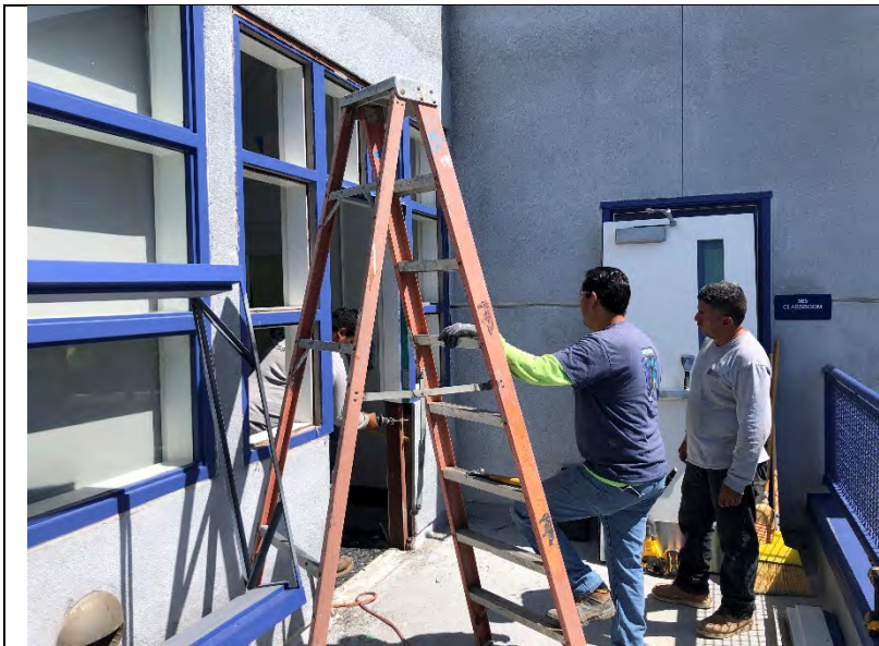
Photo 89: A hollow metal frame being removed at building D.
