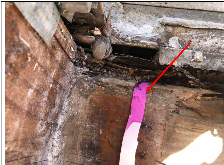
Photo 73: Dry rot, water damage, and suspected insect damage at the threshold of classroom 480
