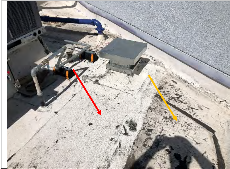
Photo 134: The existing BUR with a coating (yellow arrow) and the new granulated cap sheet (red) were installed at the new mechanical curbs.
