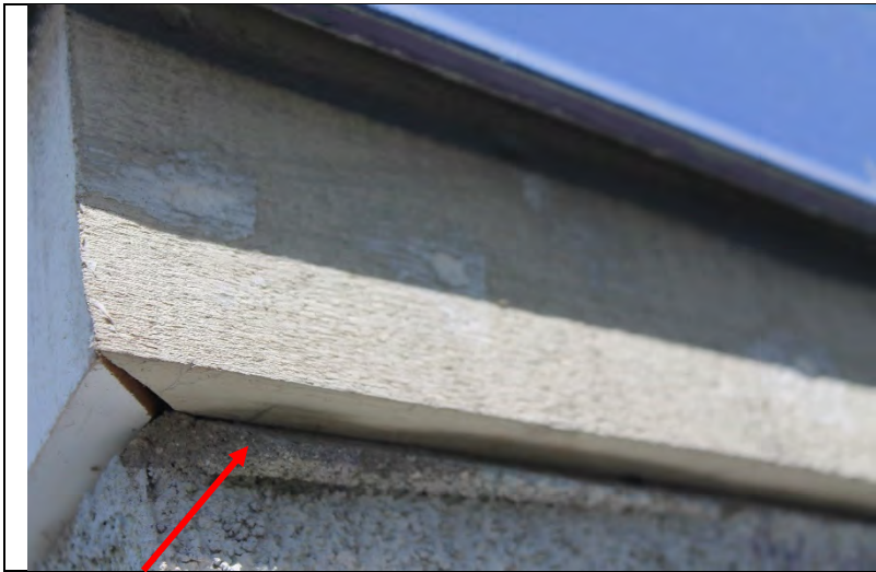
Photo 38: An opening at the top of the cement plaster assembly.
