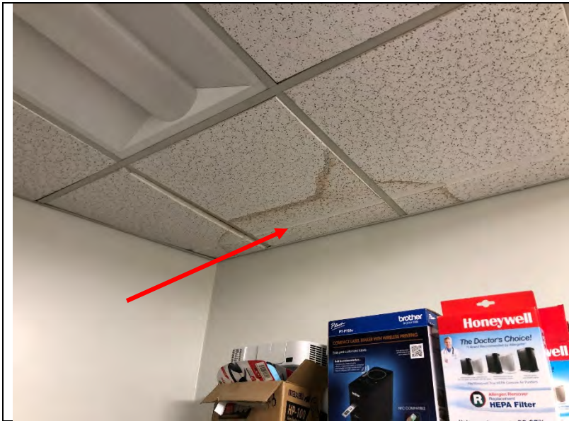
Photo 180: Staining was visible on the ceiling tiles in room 210B Media Equipment
