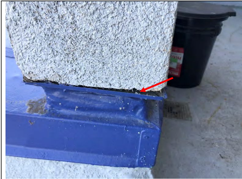
Photo 05: Abrasion and impact damage at the bottom of a plastered column.
