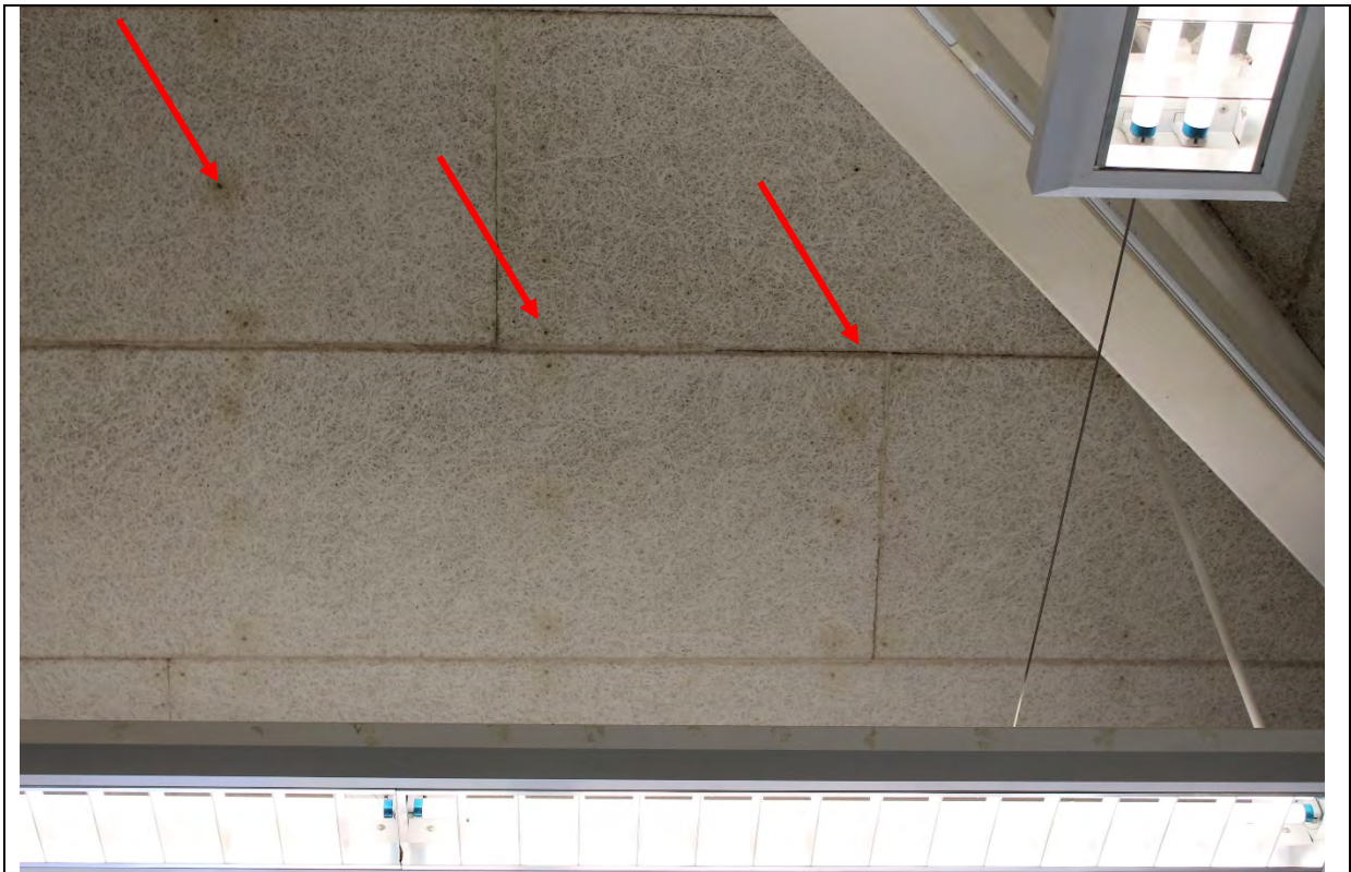
Photo 219: Water marks and staining at the acoustical panels on the ceiling of the classrooms in building D.
