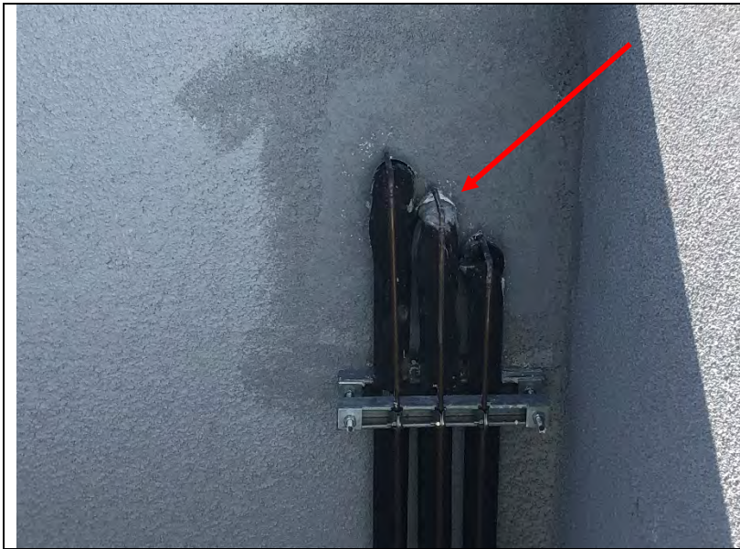
Photo 11: Penetrations in the cement plaster assembly.
