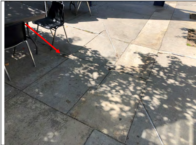
Photo 225: Drains in the hardscape were often not at the lowest points.
