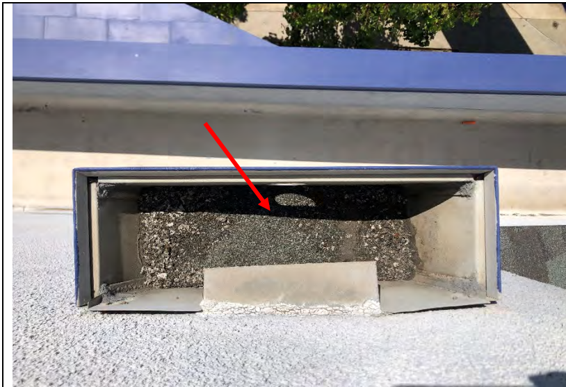
Photo 153: Granules had filled and blocked a scupper downspout.
