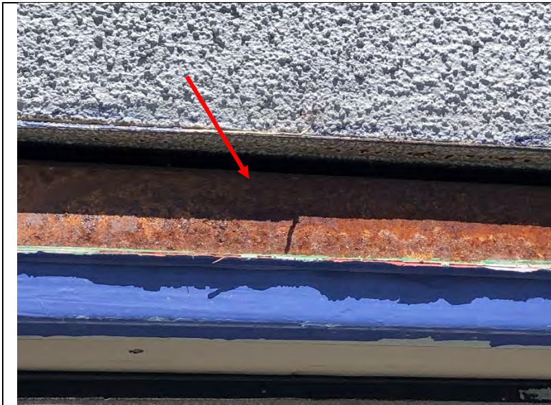
Photo 96: Corrosion was observed behind a head flashing at one of the hollow metal framed doors.
