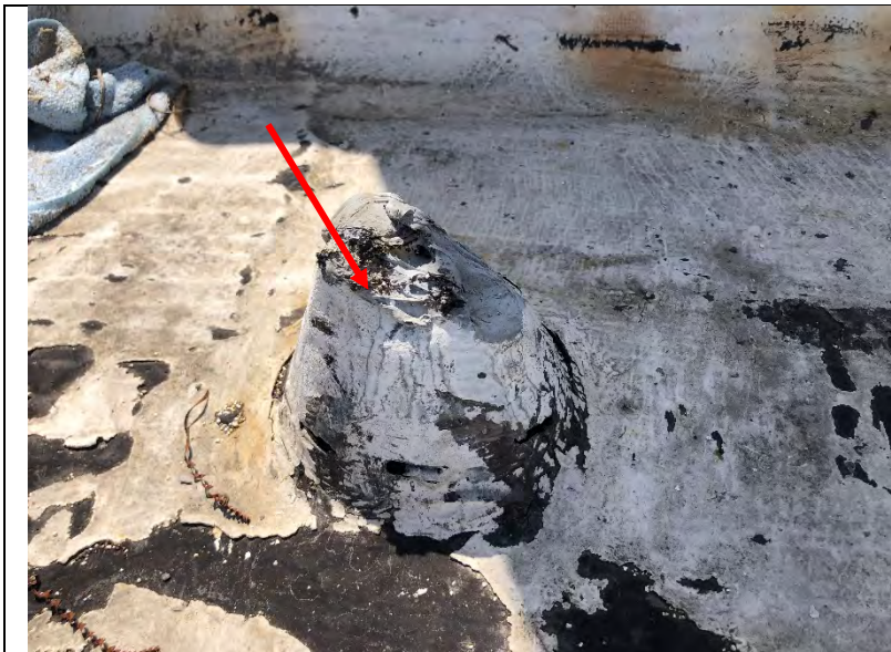
Photo 138: An abandoned cone-flashing on the roof of the multipurpose room.
