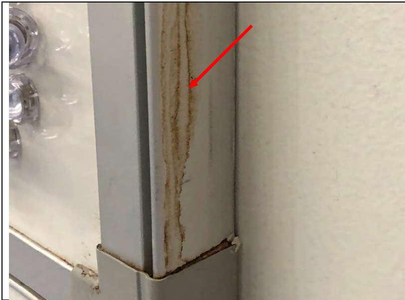
Photo 189: Water stains on the whiteboard in classroom 415.
