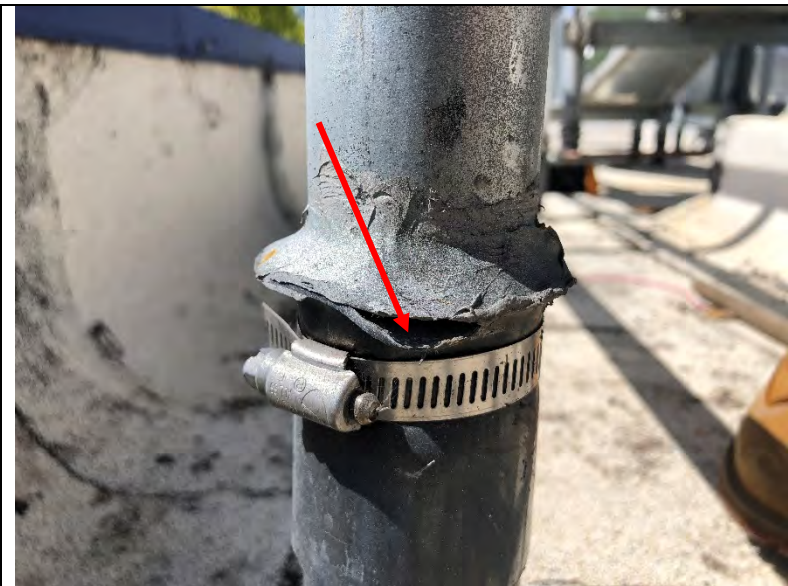
Photo 143: An opening at a lead flashing was installed in the newly installed granulated cap sheet on the roof of the multipurpose room.
