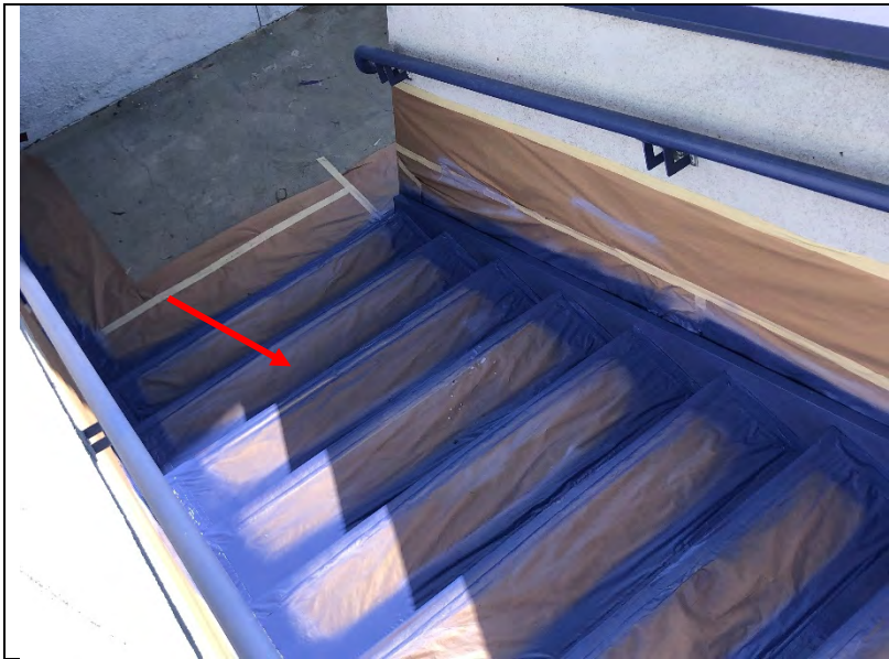
Photo 67: The stairs were masked off during painting.
