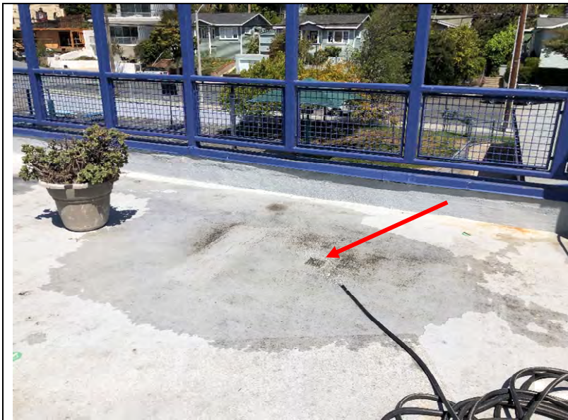
Photo 55: Flood testing of a square traffic coating drain over Communications room 205.
