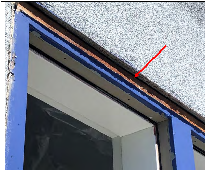
Photo 95: Corrosion was observed behind a head flashing at one of the hollow-metal framed doors indicating moisture behind the flashing.
