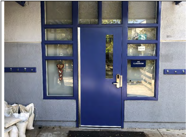
Photo 97: A hollow metal frame door/window assembly.
