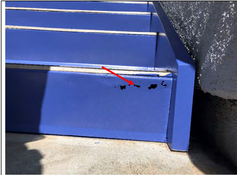
Photo 68: Corrosion was observed on the stairs after repainting.
