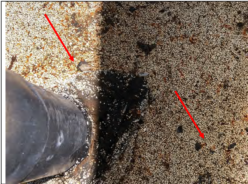
Photo 137: Pock-marks and welding damage on the newly installed granulated cap sheet on the roof of the multipurpose room.
