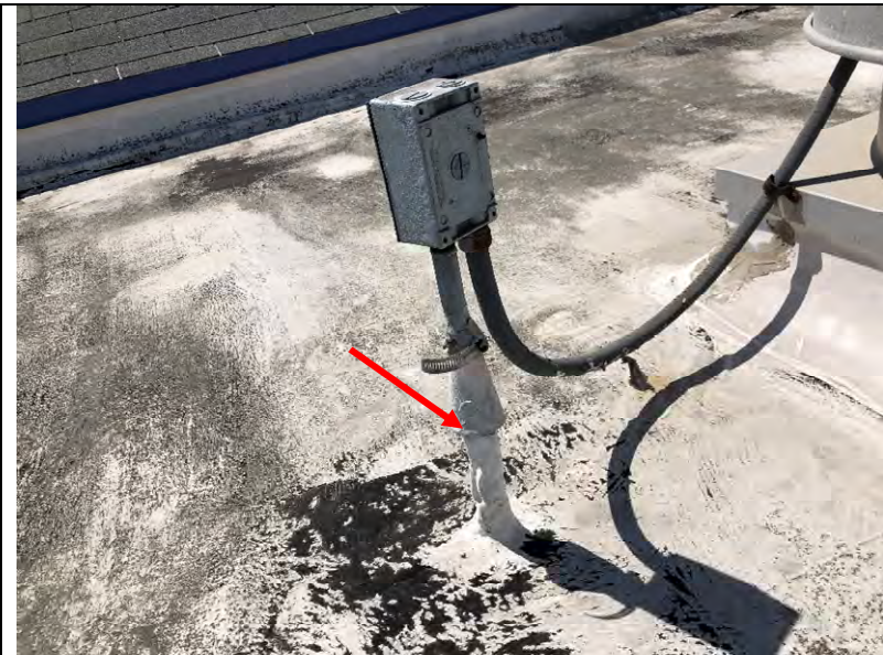
Photo 144: An electrical conduit flashing with a drip guard on the roof of the multipurpose room.
