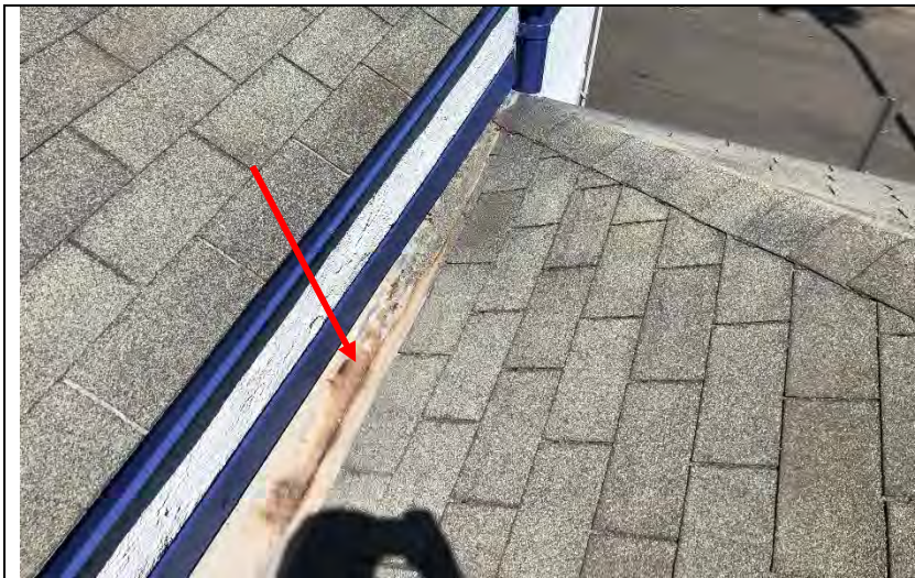
Photo 167: Sheet metal flashing on the asphalt shingle roofs showed various signs of age degradation.
