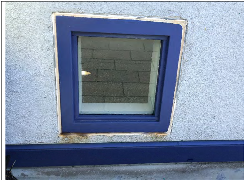
Photo 100: A hollow metal frame window at the saw-tooth roof.
