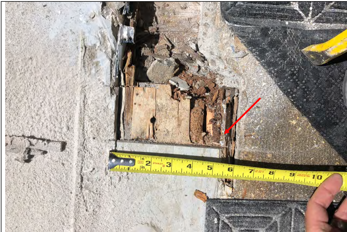
Photo 87: Water damage at the jamb to sill juncture at the threshold. DTR requested that this area be cut and opened for further visual observation.
