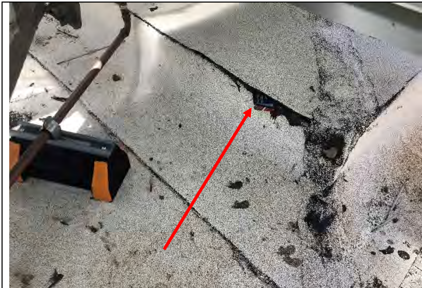
Photo 133: A business card was inserted into a gap in the new granulated cap sheet installed at the new mechanical curbs.
