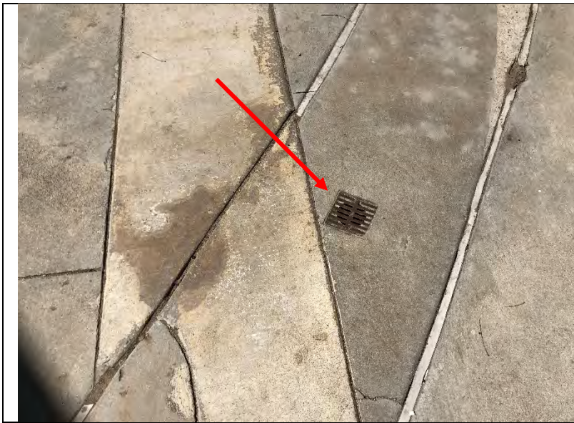
Photo 226: Drains in the hardscape were often not at the lowest points.
