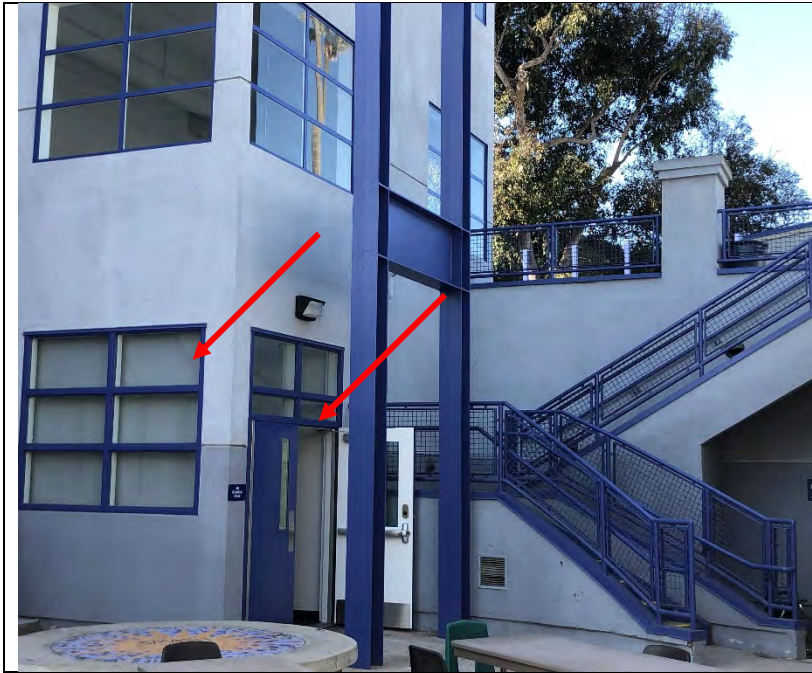
Photo 98: Hollow metal frame assemblies.
