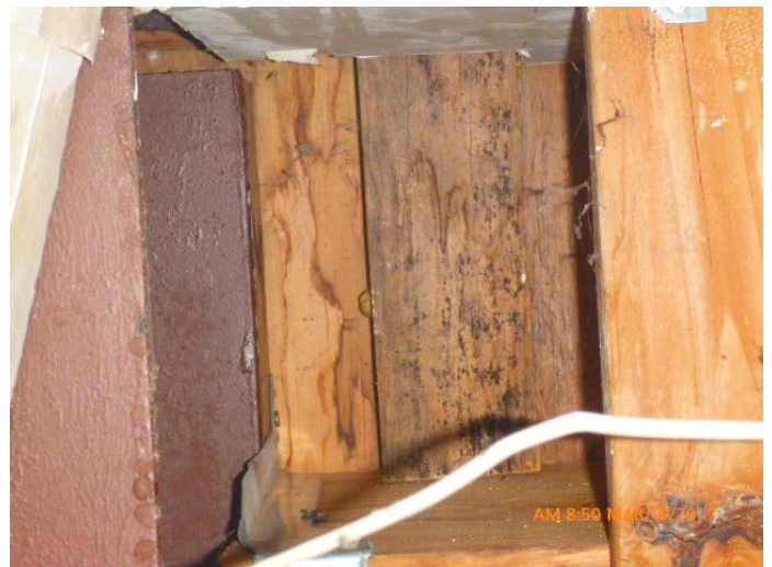
Photo 38: Close-up of staining on wooden beams
