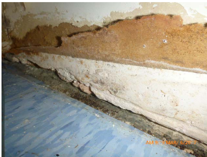
Photo 55: Mold growth and strong musty odors observed along base of west and south walls (both sides of ext. door)
