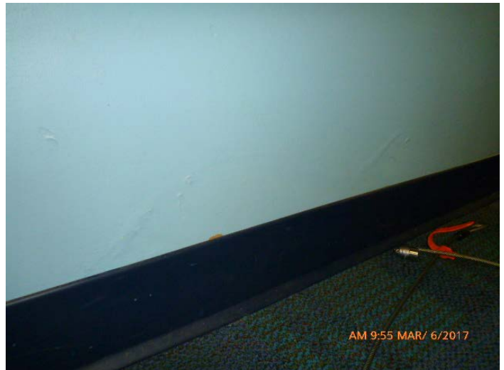
Photo 46: Moisture impact (e.g. bubbling) observed along base of south wall
