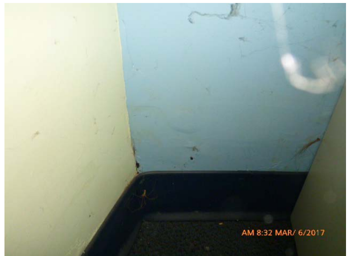
Photo #30: Overview of moisture damage along base of walls in NW corner
