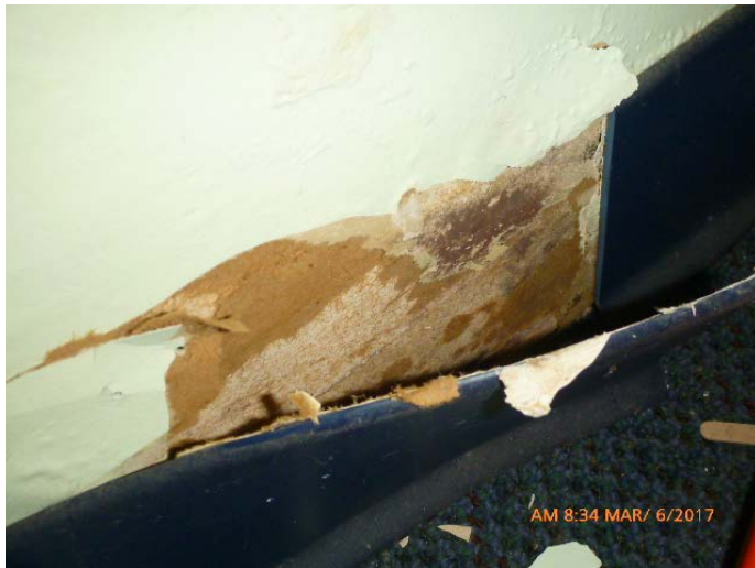
Photo #31: Mold growth observed behind base-cove on west wall
