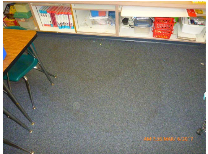
Photo #20: Stained carpeting along north perimeter
