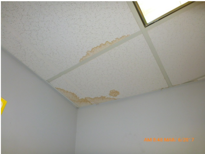
Photo 35: Stained ceiling tiles observed in SW corner
