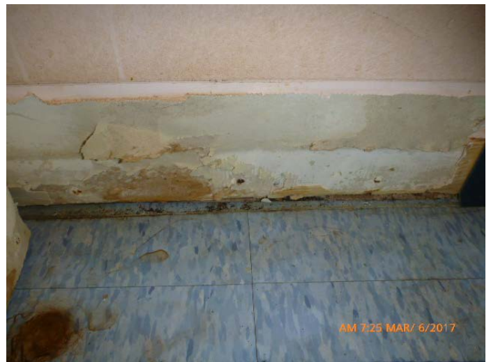
Photo #8: Close-up of base of wall and moisture impact. Staining observed on vinyl floor tile
