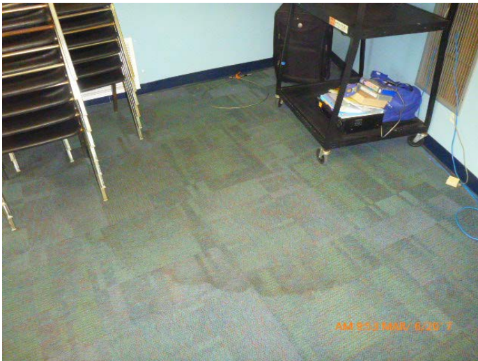
Photo 45: Large area of stained carpeting observed in SE corner
