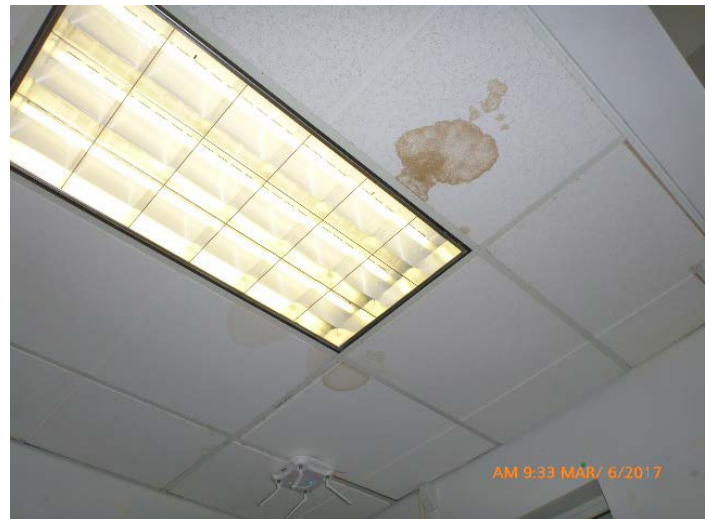
Photo 56: Stained ceiling tiles observed along north perimeter
