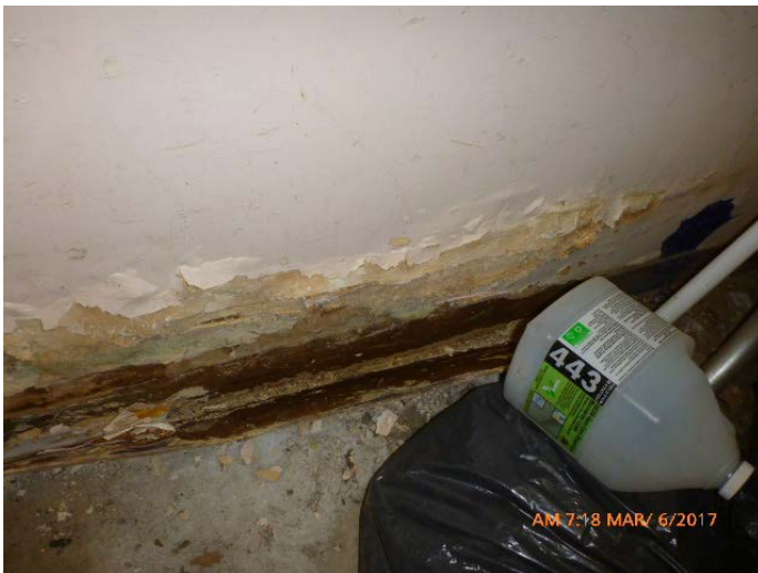
Photo #11: Heavy moisture damage, visible mold growth and elevated moisture along base of east wall
