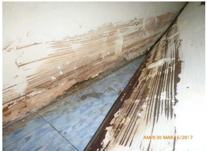
Photo 60: Moisture impact and mold growth observed along base of south and west walls
