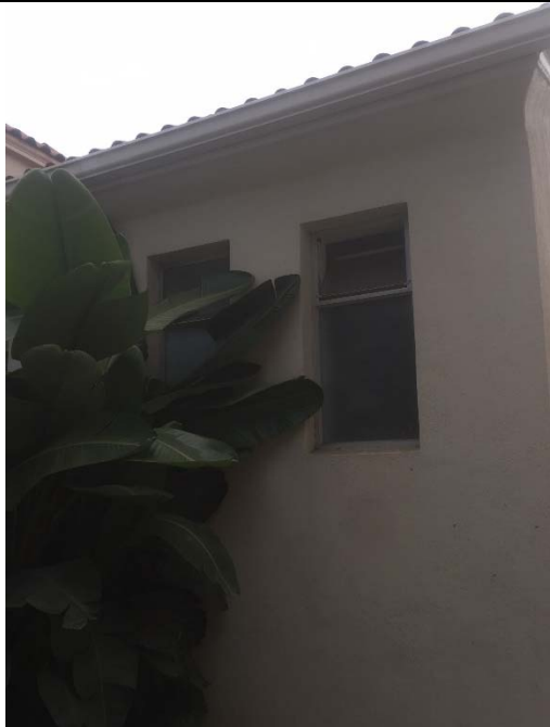
Photo 1: Example Window Type – Building C Northwest Adult Restroom
