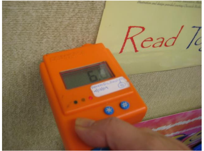
Photo #10: Moisture level readings measured at elevated levels in at N wall (pin board)
