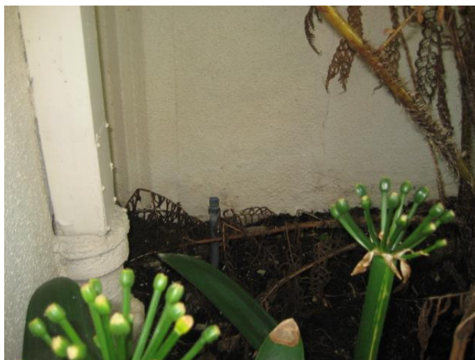
Photo #4: Exterior – rain gutter draining into planter (N wall)
