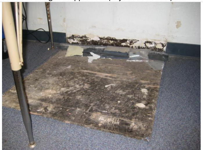
Photo #18: Annex – overview of SW lower wall – vinyl cove base and section of carpet flooring removed (note: black discoloration is mastic, not mold growth)
