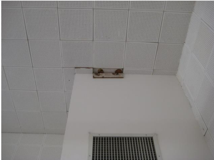
Photo #11: Library – damage/missing ceiling tile at SE corner (above the furnace closet)
