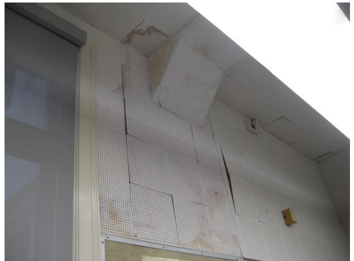
Photo #8: Library – overview of N wall – evidence of heavy moisture impacted building materials
