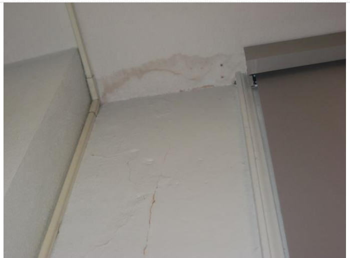
Photo #16: Annex – overview of SW upper wall – evidence of moisture impacted building materials at ceiling and upper wall (adjacent window)
