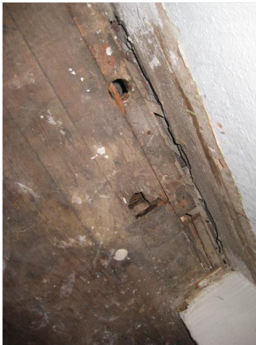
Photo #20: Annex – closeup of wood subfloor at NW wall – damage and warping of wood member observed
