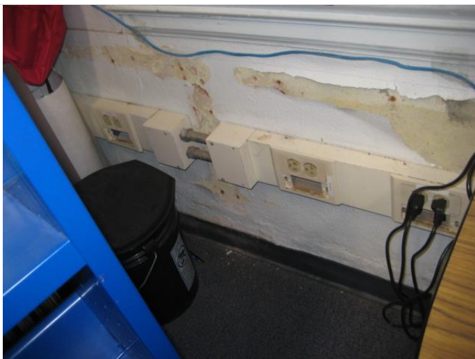
Photo #17: Annex – overview of SW lower wall – evidence of moisture impacted building materials (blistering paint, damage) below the window
