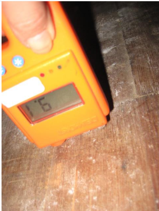
Photo #21: Moisture level readings measured at acceptable levels at the wood subfloor at NW wall
