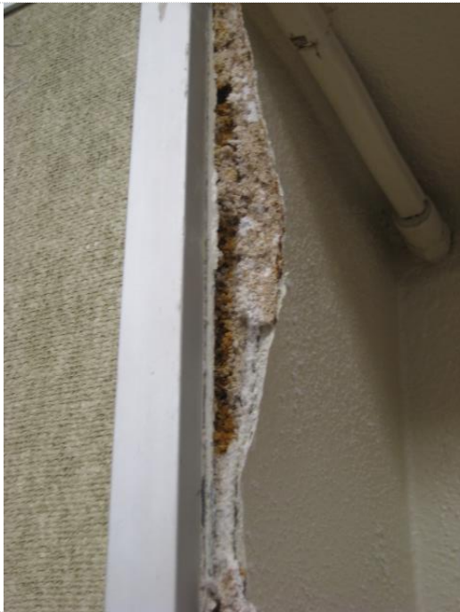
Photo #9: Library – N wall – close up of damage to building material
