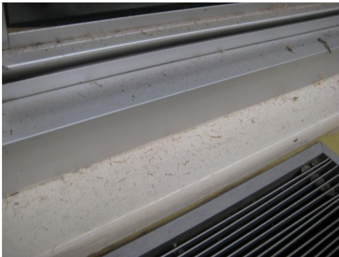
Photo #13: Library – heavy dust/debris deposition observed at N windowsill (adjacent N planter)
