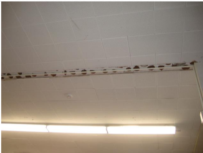
Photo #15: Annex – missing/damage ceiling tiles observed
