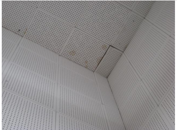
Photo #12: Library – moisture impacted ceiling tile at NE
