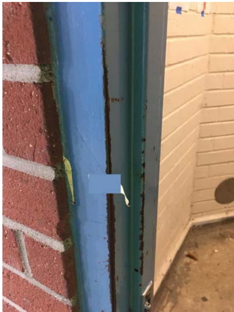
Sample #11-Exterior door caulking Photo #11
