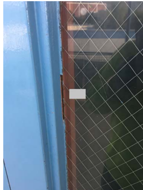
Sample #8-Exterior window caulking Photo #8
