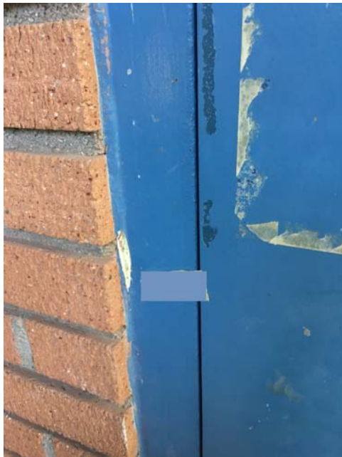
Sample #5-Exterior door caulking Photo #5
