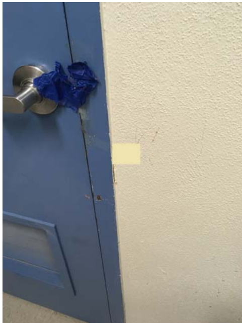
Sample #1-Interior door caulking Photo #1
