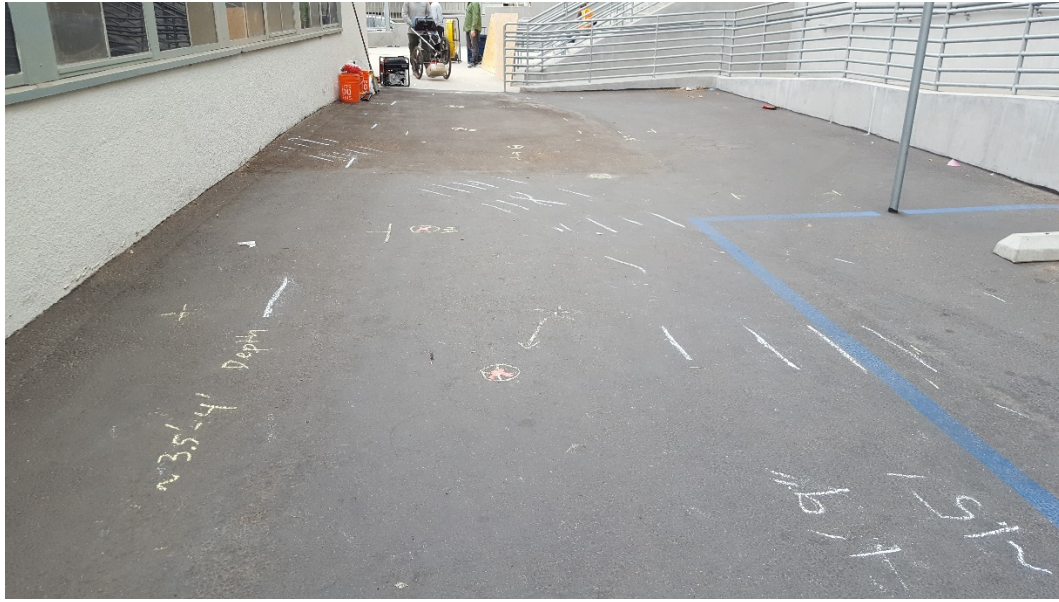
Photo 3 – Geophysical Survey to locate Underground Utilities
