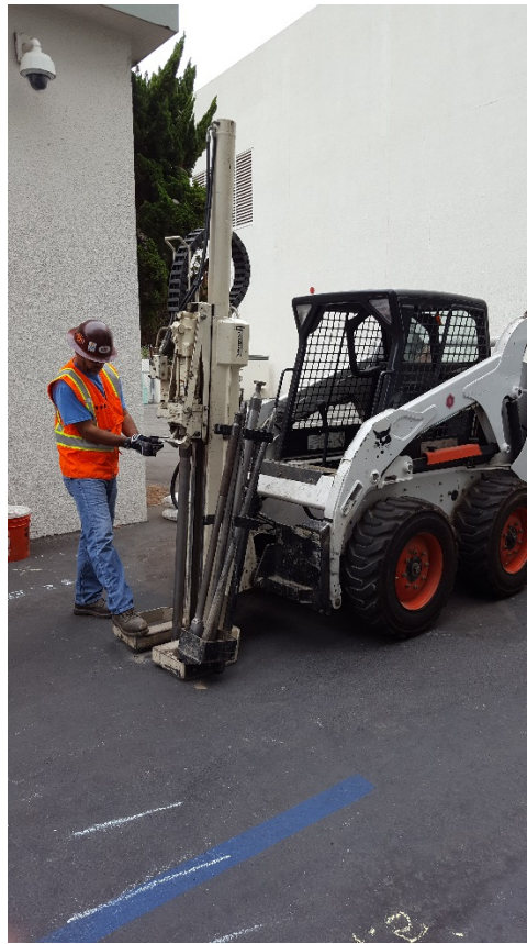
Photo 4 – Drilling and Sample Collection
