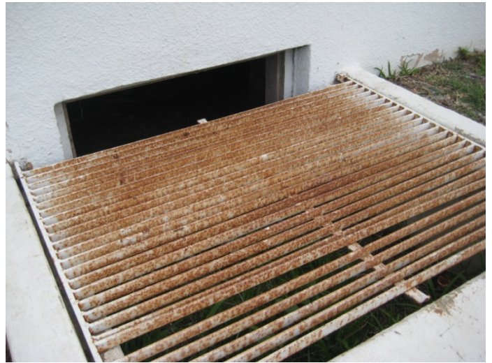
Photo #18: Open crawl space vent – south elevation
