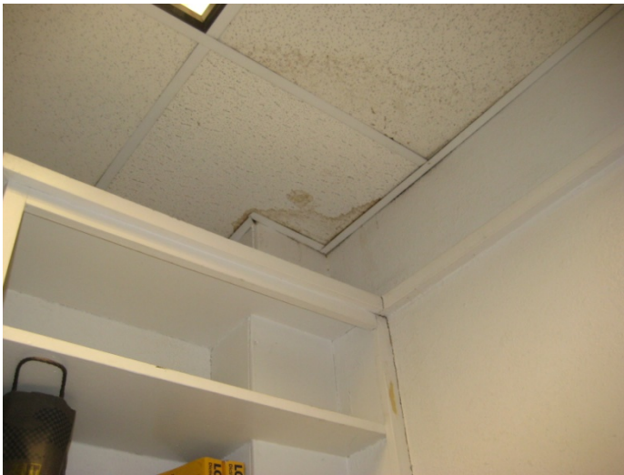
Photo #9: Discoloration/staining observed on the ceiling tile at the southwest corner – teacher's work area
