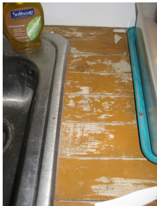
Photo #12: Wood counter top adjacent sink—measured moisture level not elevated – 9.7% - 10.1%
