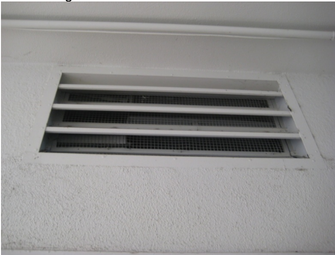
Photo #19: Fresh air supply – unobstructed – wire mesh in place
