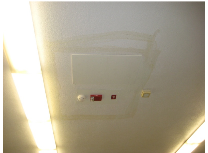
Photo #8 Light discoloration/staining observed on the center of ceiling
