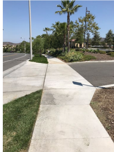
Left: Level walking path provides a continuous walkway across a driveway.
