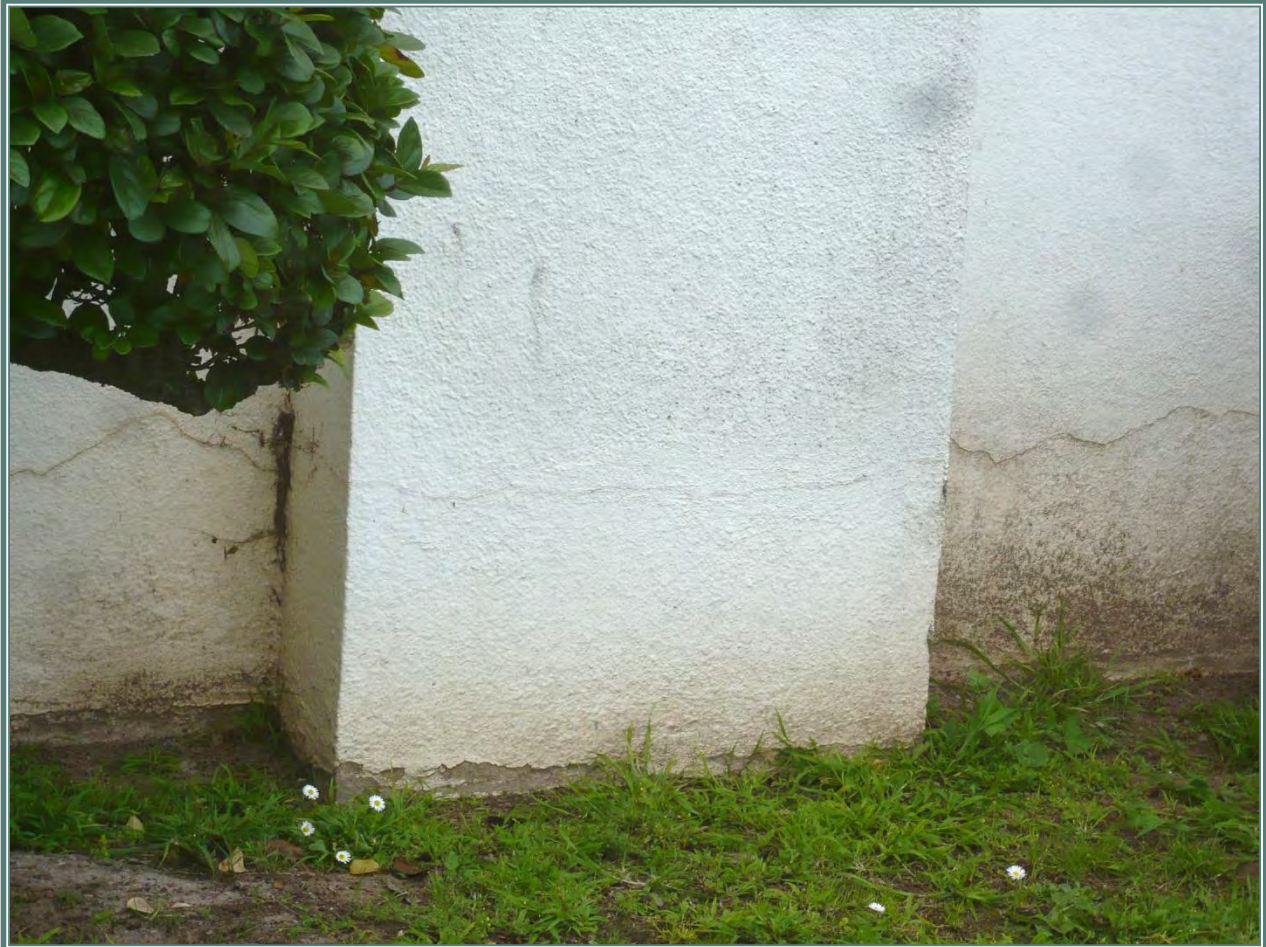
TYPICAL STRESS CRACKING AT SUPPORT COLUMN LOCATIONS ON THE EAST AND WEST WALLS OF THE AUDITORIUM
