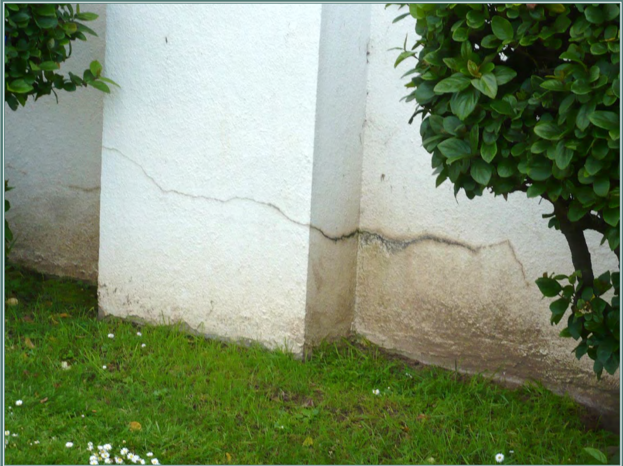
STRUCTURAL STRESS CRACKING ALONG FOUNDATION LINE OF PERIMETER WALLS IS TYPICAL AT THE EAST AND WEST WALLS OF THE AUDITORIUM
