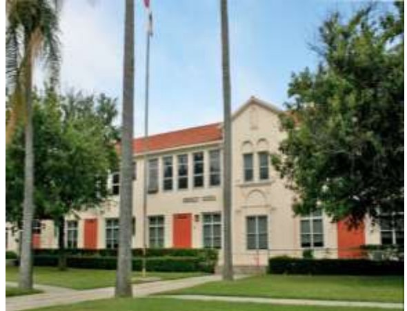
McKinley Elementary School
