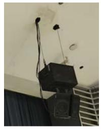
There is a provision for the suspension of a center cluster above the boxing ring location, but no speaker system is currently installed in that location. There is also a cable reel for a microphone to be lowered to the boxing ring, but no microphone is installed.
