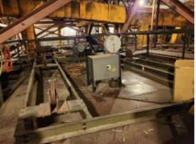
There are accommodations for suspending a central speaker cluster above a boxing ring, along with a cable hoist for a microphone.
