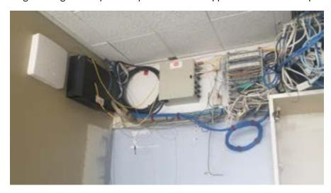
There are three locations where POE switches are installed for the data, voice, and WIFI systems through fiber cables from the MPOE. These switches are mounted on wall-mounted racks.
