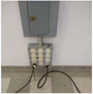
Figure 4.3.5 – Twistlock Receptacle Block
