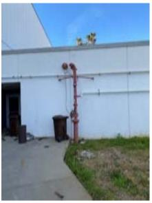
Figure 4.5.4 - East Wing Fire Riser Assembly
