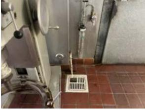
Figure 4.4.4 – Floor Sink for Fire Sprinkler Aux. Drain
