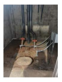
Figure 4.4.3 - Sewage Ejector in Basement
