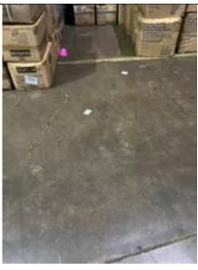
The concrete fill of the tilt floor appeared to have multiple cracks over its floor area that have been repaired with some kind of epoxy product that filled the cracks. A large portion of the floor was covered with boxes and other storage items that prevented a complete observation of the entire floor area. The type of epoxy repair used is unknown and effective strengthening capacity may be uncertain.
