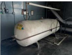
Figure 4.4.1 - Gas-Fired Domestic Boiler
