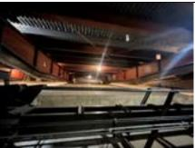
The steel members appeared to be in good condition. The main girders appeared to have been strengthen by an added steel section below the bottom flange.
