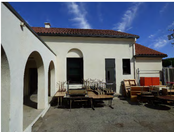
Building C. South view.
