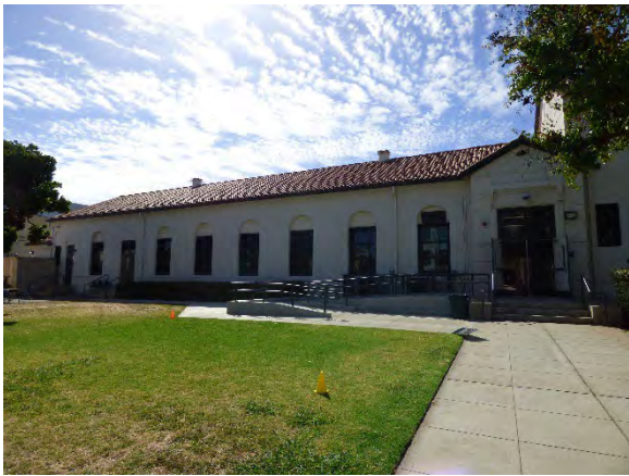
Building C. West view.
