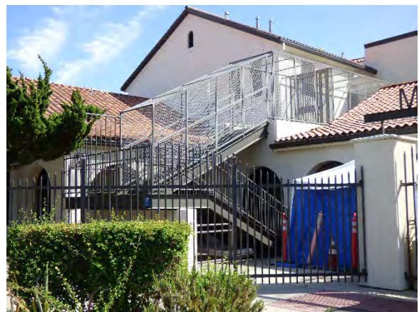
Detail, staircase. Building C. South view.
