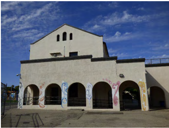
Building B. East view.
