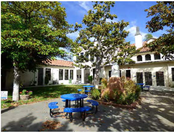
Building C. Southeast view.
