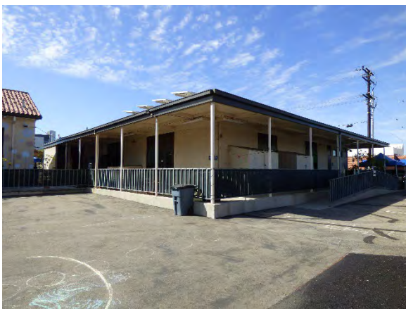
Building D. North view.
