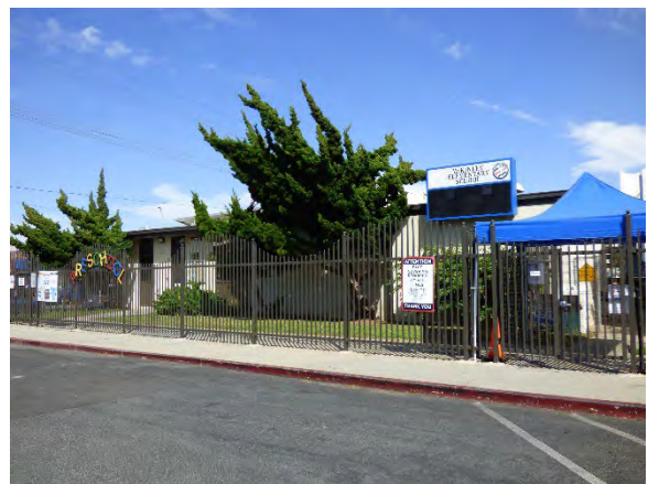
Building D Southeast view.
