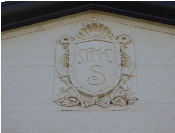
Detail, Building C. Northwest view.
