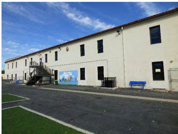
Building B. Southwest view.
