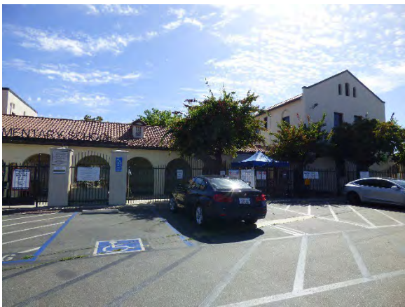
Building C. West view.
