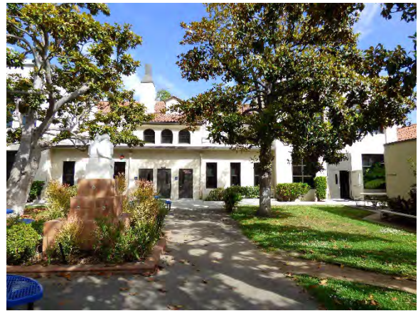
Building C. Southwest view.
