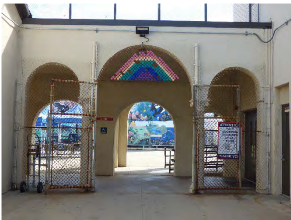
Arcade, Building C. East view.
