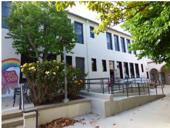
Building B. North view.
