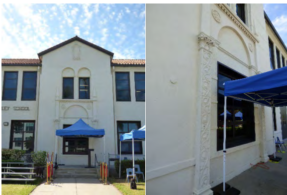
Entrance, Building C. Northwest and North view.
