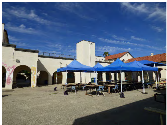
Building C. East view.
