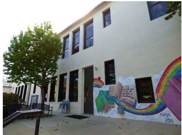
Building B. Northwest view.
