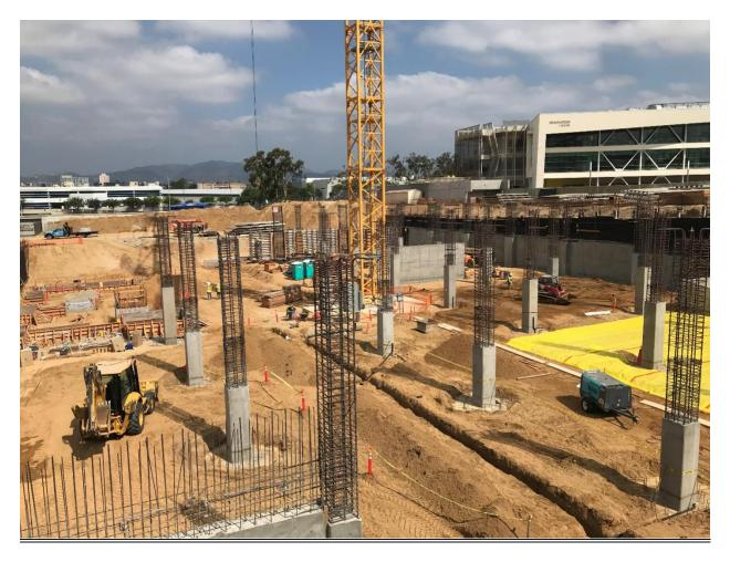
Bases are complete for three of four quadrants. The wall and columns for the second level of parking are now 50% complete and waterproofing for the floor slab is installed.
