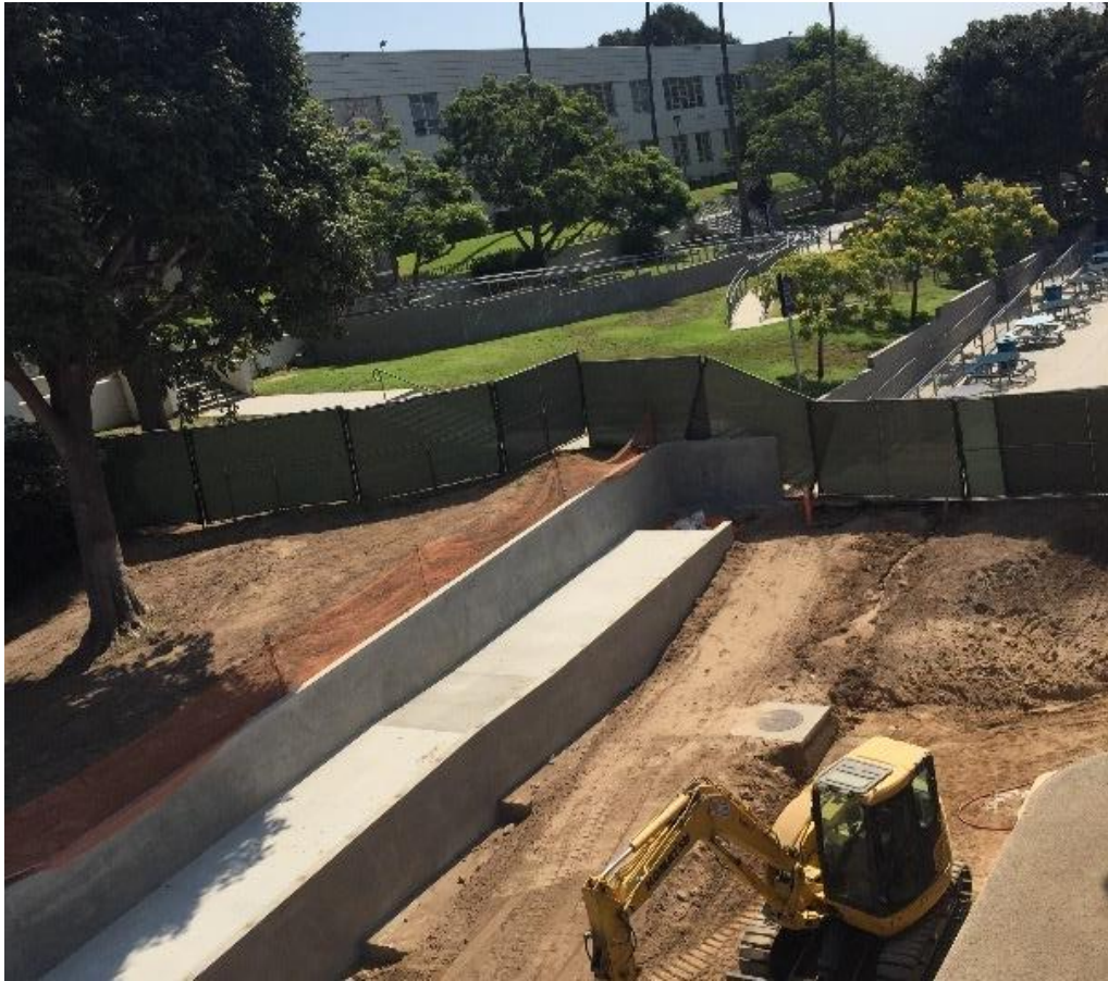
This view of Viking Way between Barnum Hall and the Business Building shows the removal of the stairs at that location to make way for a revised configuration with one flight of steps instead of two. That eliminates the need for a second ramp.
