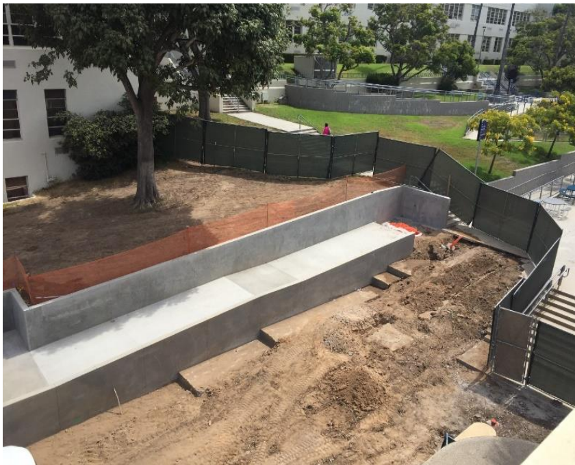
This view of Viking Way between Barnum and Admin, shows the removal of the stairs at that location to make way for a revised configuration, with one flight of steps instead of two, which will eliminate the need for the second ramp.
