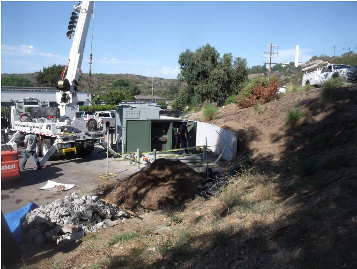
Preparations for the new transformer in the upper parking lot.
