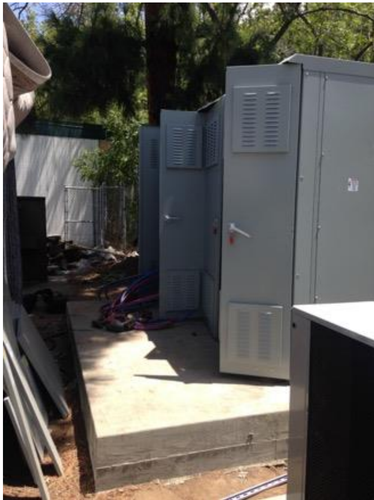
New electrical switchgear awaits power-up.
