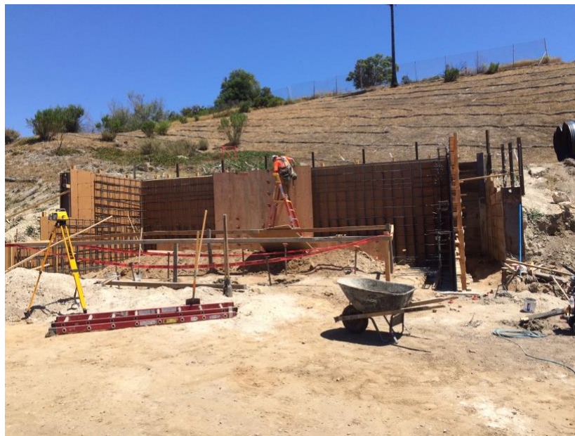
Rebar and forms being placed for a retaining wall at the location of the new chiller plant.
