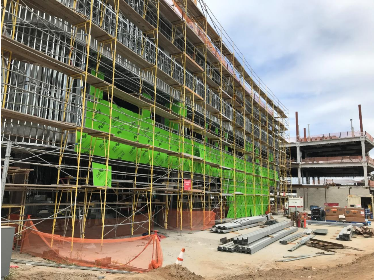
Most of the framing is complete on the south building, allowing workers to start closing up the building with sheathing.
