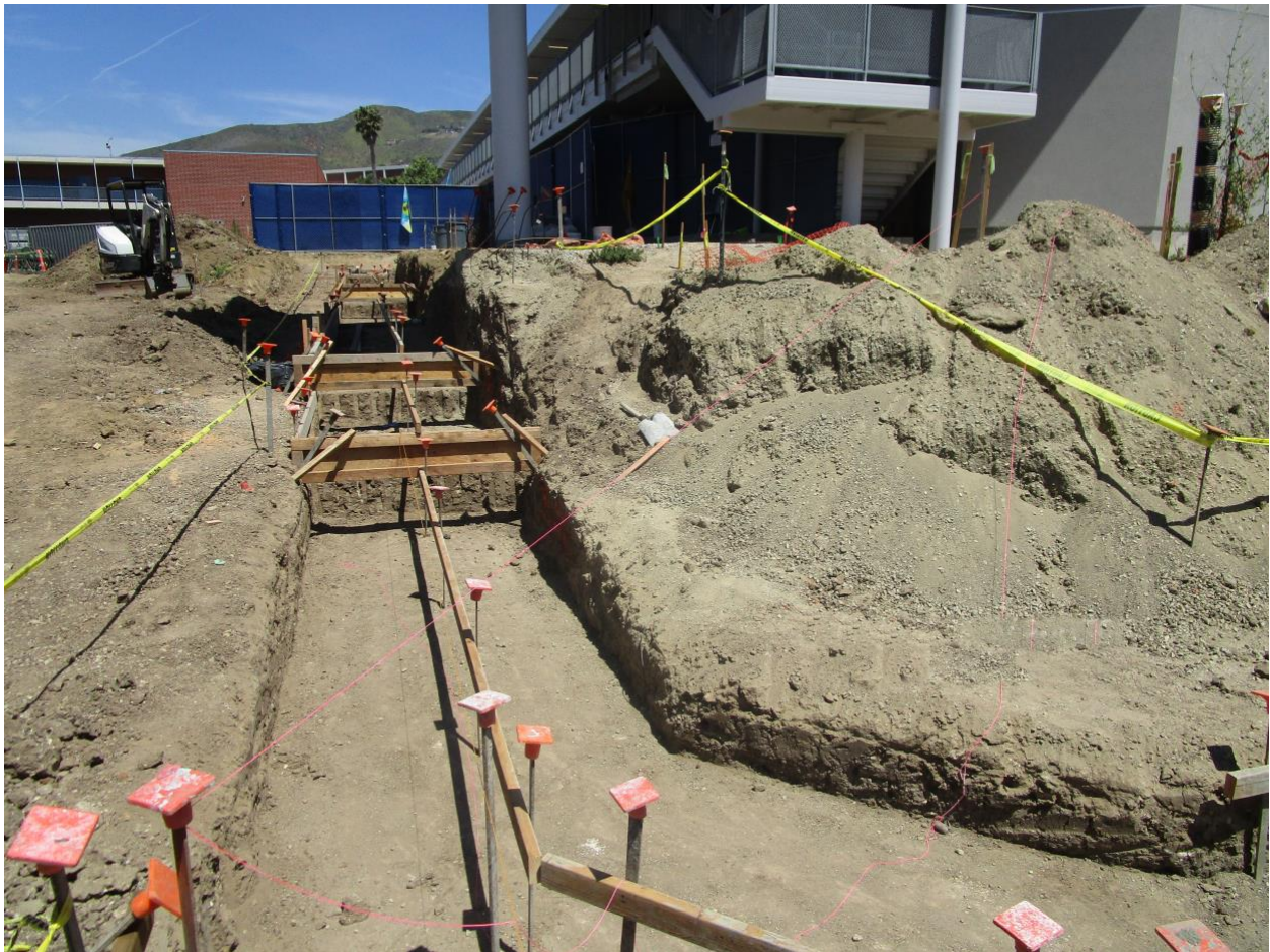
Preparation being made for the pouring of a ramp footing.
