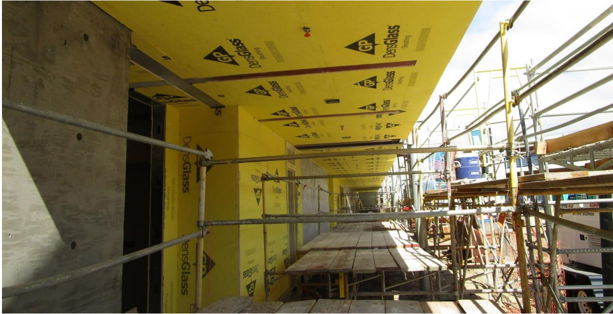
Exterior sheathing seen on the north side of the new administration and library building.
