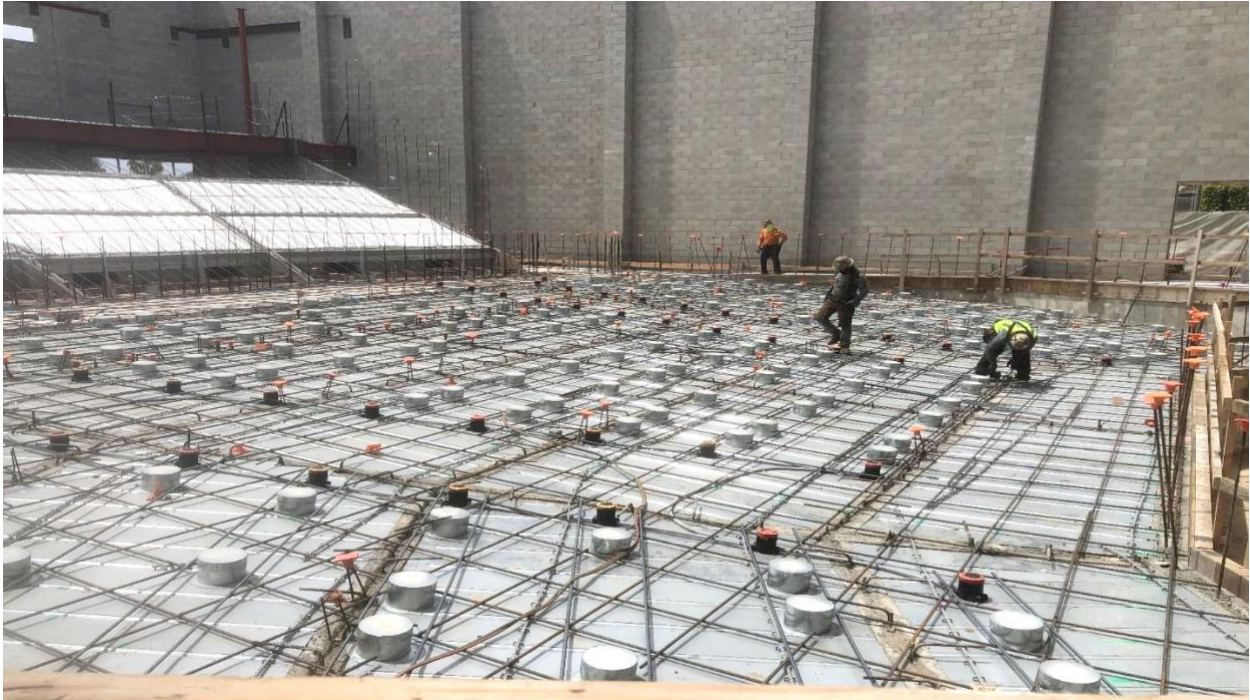
Workers finish installing rebar for the lower seating area in the theater.
