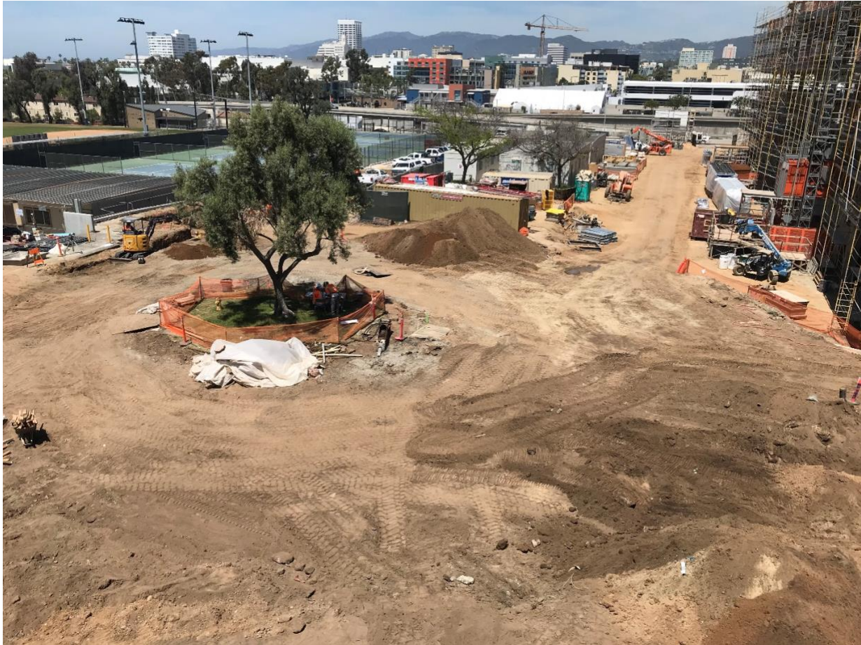
The old traffic circle and half of Viking Way have been prepared for the installation of utilities and the construction of retaining walls
