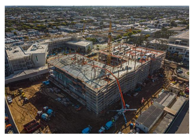
McCarthy completed the final deck pour of the building on April 7 (almost a year after construction began) with the completion of the concrete roof deck on the north building.
