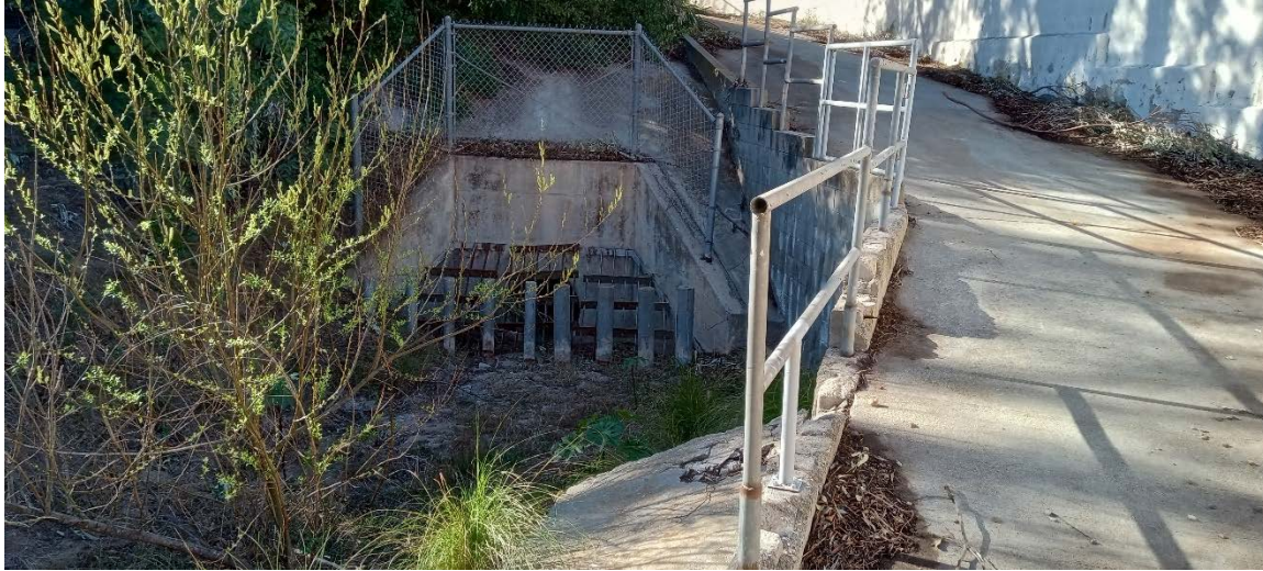
Headwall with debris rack at downstream terminus of earthen channel; vehicle access way on right
