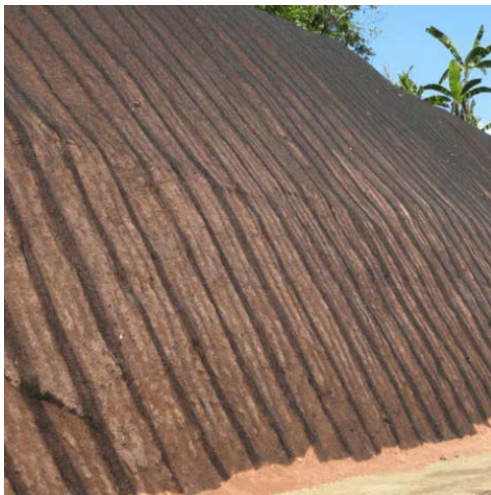
Example of geotextile erosion control mats installed on a steep slope
