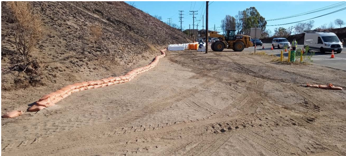
Sand bag barrier and concrete barriers along toe of slope north of School
