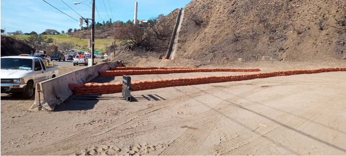
Sand bag barriers and concrete barriers at culvert inlet north of School, concrete terrace drain also visible
