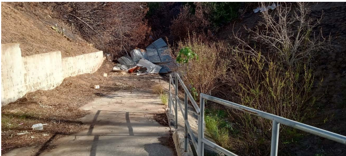
Looking upstream in earthen channel from top of vehicular access way, note debris accumulation
