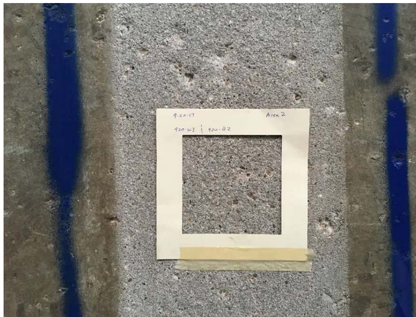
Representative close-up photo of Pilot Study Area 1, Strip 2 after bead blasting
