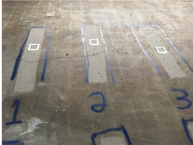
Representative photo of Pilot Study Area 1, showing Strips 1, 2 and 3 after bead blasting
