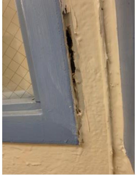
Photo 9. Room 401 - Interior window gap in encapsulant.
