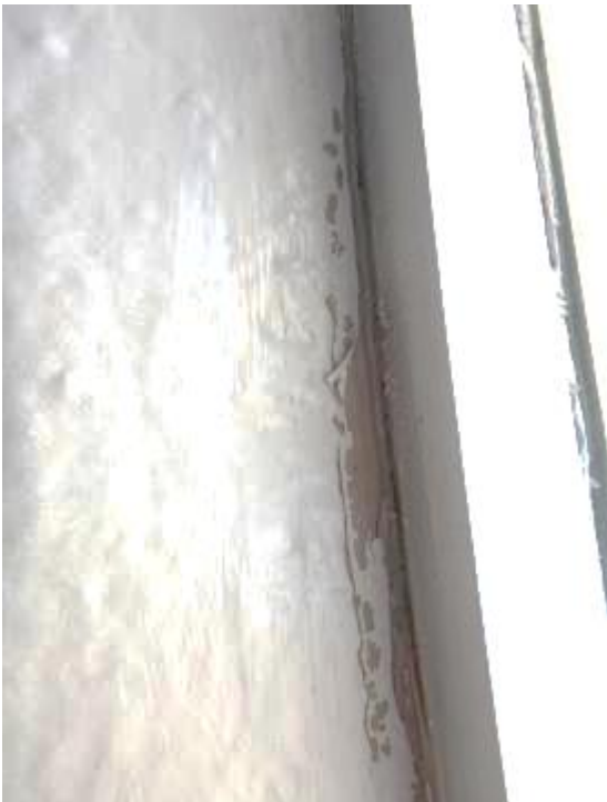
Photo 27. Room 22 - Additional interior window gap in encapsulant.
