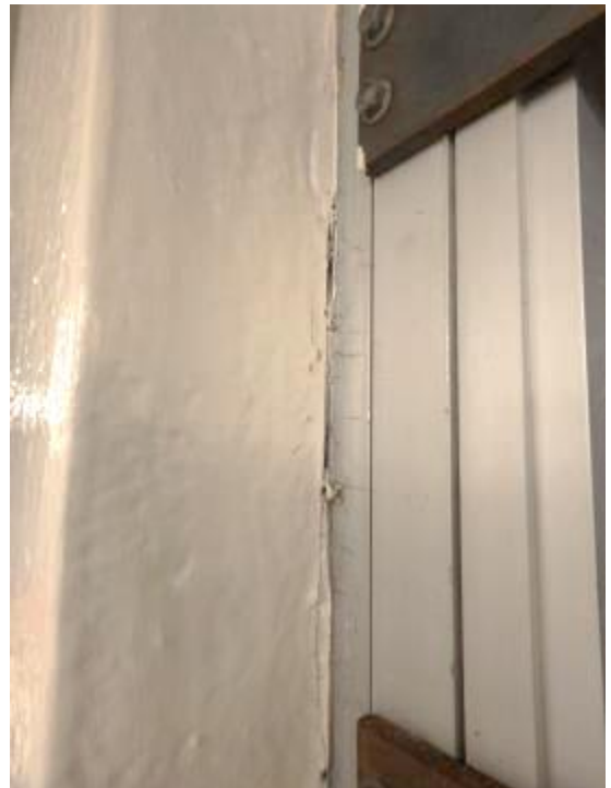
Photo 4. Room 801 - Additional interior window gap in encapsulant.
