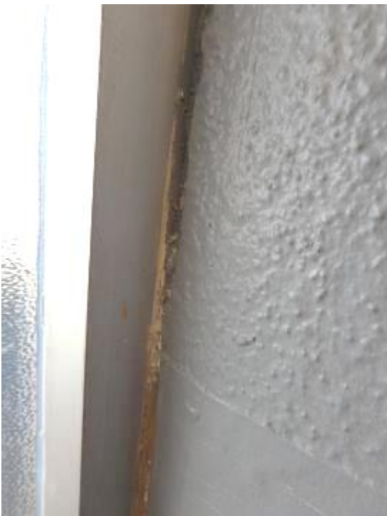
Photo 16. Room 18 - Interior window gap in encapsulant.
