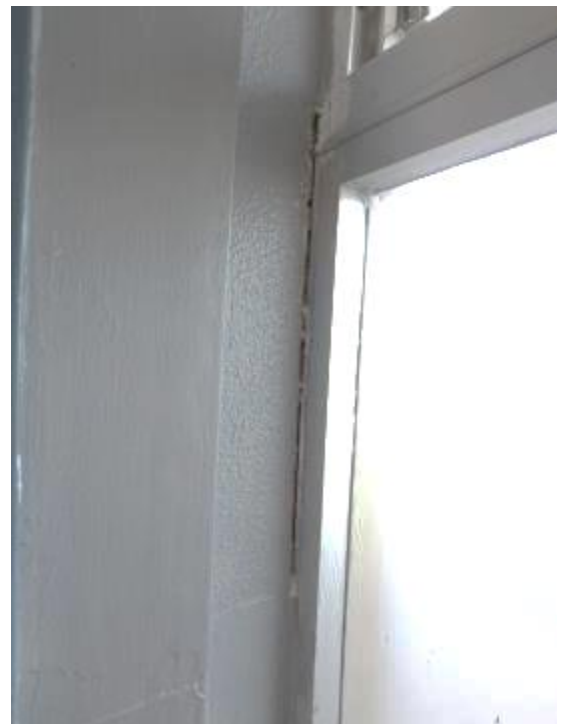
Photo 17. Room 18 - Additional interior window gap in encapsulant.
