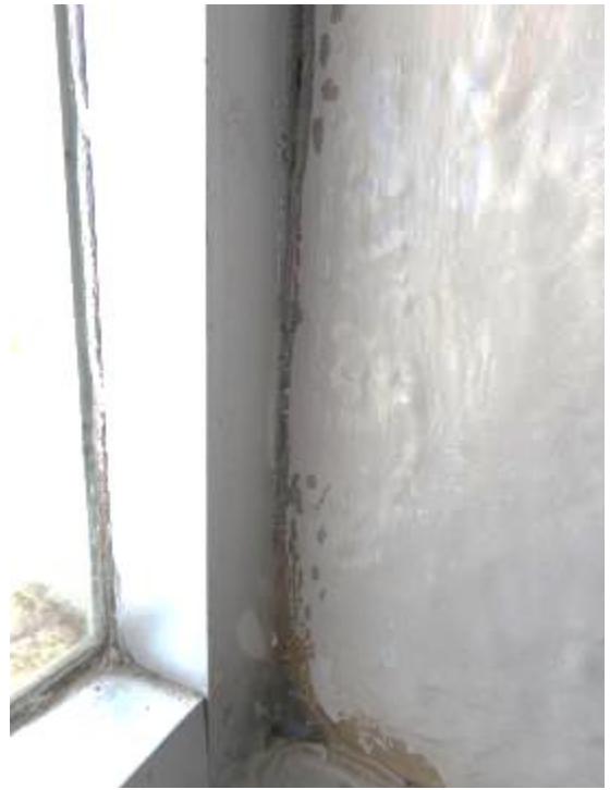
Photo 26. Room 22 - Additional interior window gap in encapsulant.
