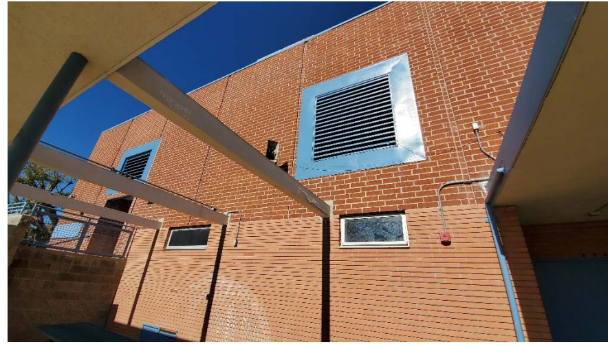
Photograph 1 – View of metal cladding in in the Mechanical Closets above Rooms 662/666.
