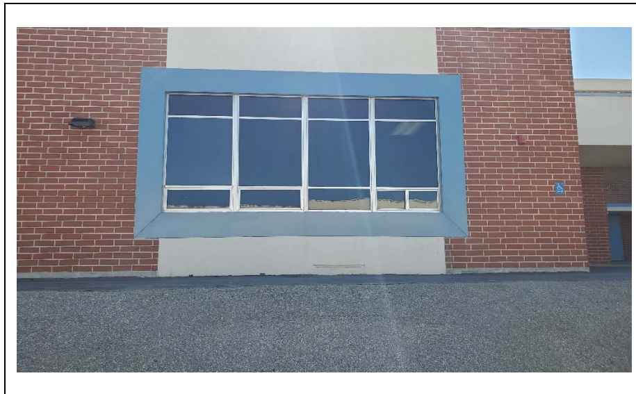
Photograph 2 – View of metal cladding around windows of Rooms 704/705.
