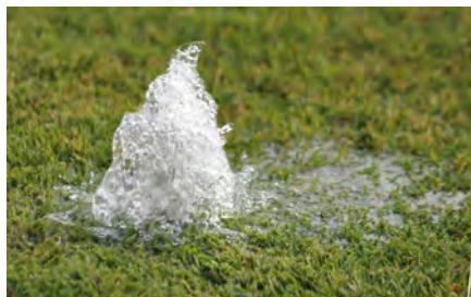
Example of Broken Sprinkler
