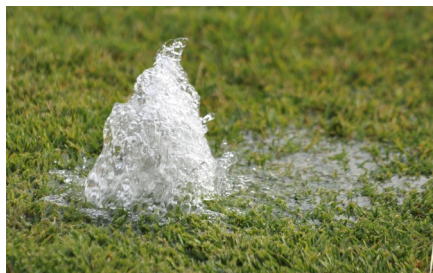
Example of Broken Sprinkler
