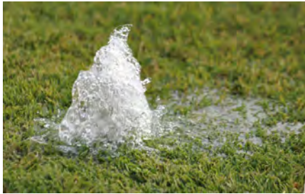
Example of Broken Sprinkler
