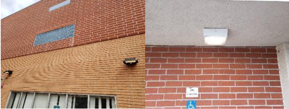
Figure 23. Exterior LED lights on seen from when traveling from auditorium to the teacher lounge. Also, light on during the day near the gymnasium.
