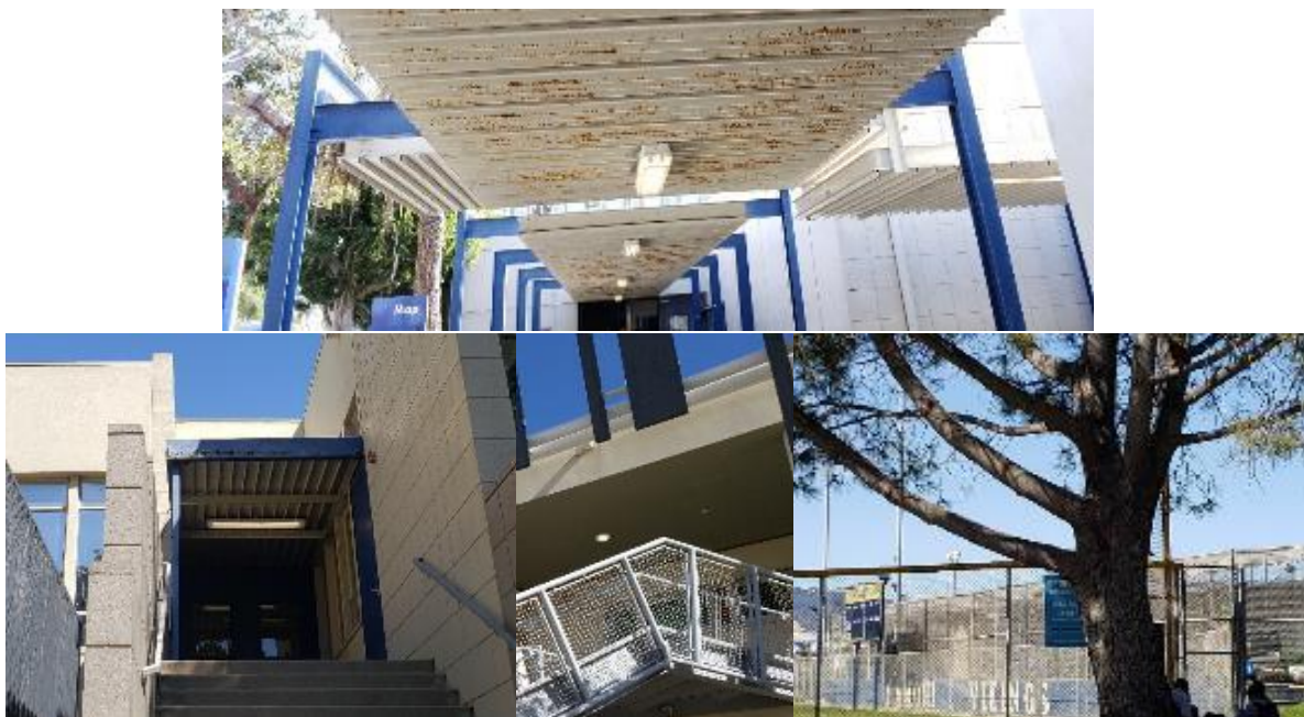
Figure 9. Exterior lights found turned on near the Admin building, multiple lights on around the innovation building, and near the construction of the parking lot.
