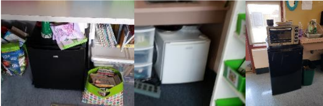
Figure 13. Mini-fridges found on-campus classrooms and break rooms. It is recommended to replace three mini-fridges with a single full-sized fridge. A mini-fridge uses roughly half of the power for a quarter of the storage capacity of a full-size refrigerator.
