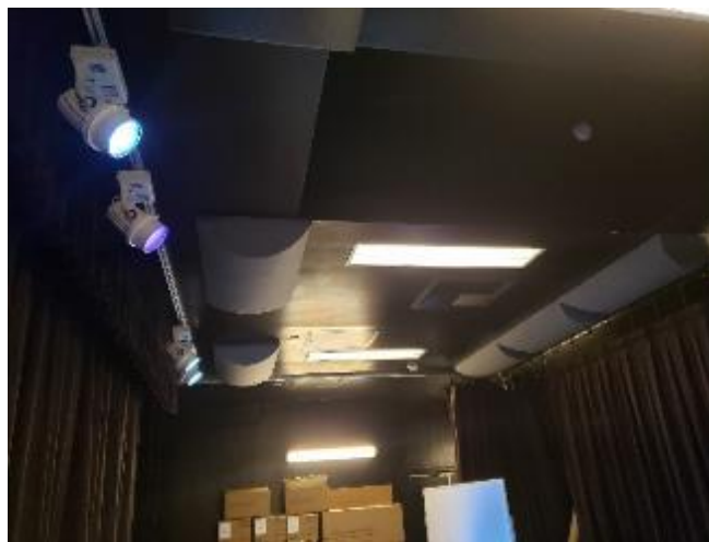
Figure 7. The stage lights left on while the stage was not used. The multipurpose room was set up to be a voting area, but curtains for the stage were pulled to close off the light.
