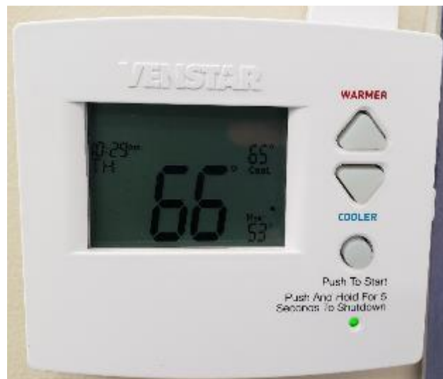
Figure 17. The setpoints are low, at 53°-65°F, in room 110.
