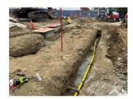
**STEM building**Site utilities and gas line relocation in progress.
