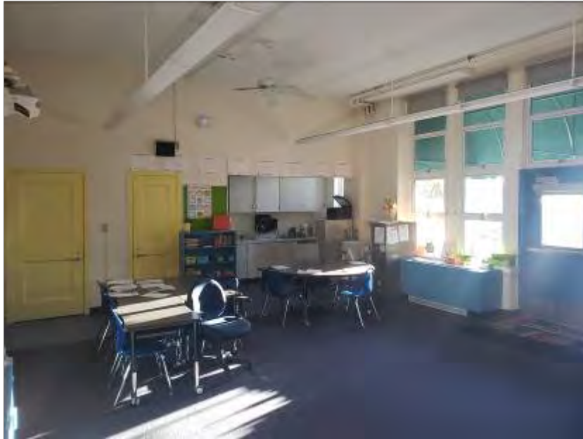
Photo 11: Typical Classroom Interior
