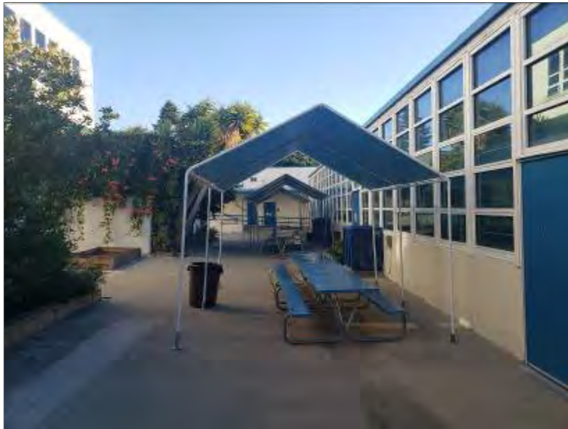
Photo 20: Classroom Building Exterior
