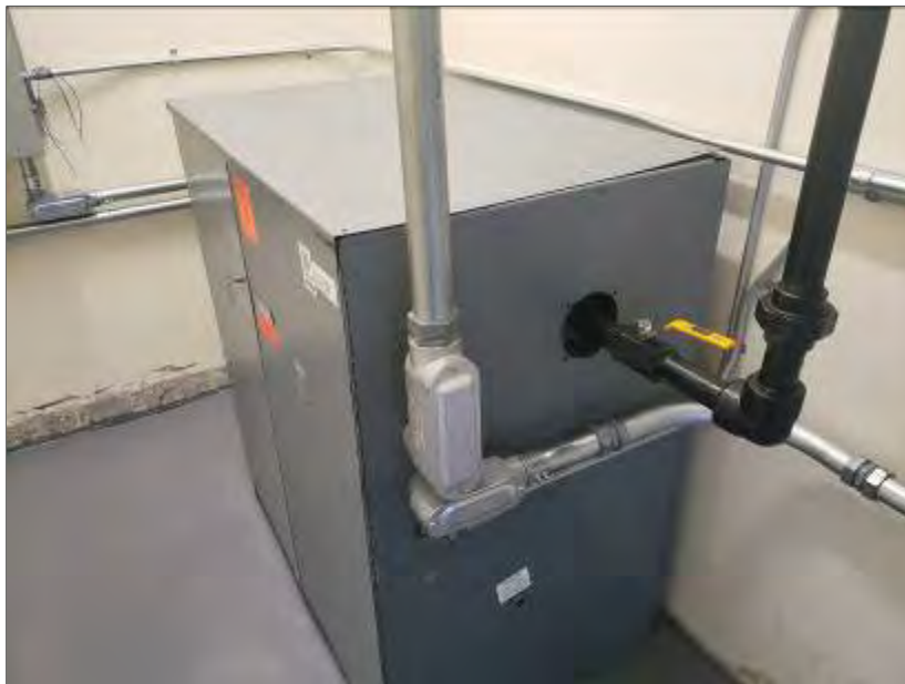
Photo 16: Passenger Elevator Equipment
