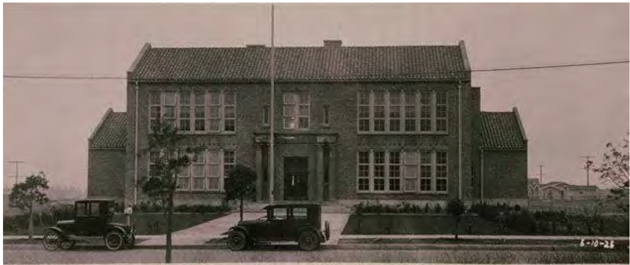
Original Franklin School, 1928 (Santa Monica Public Library)
