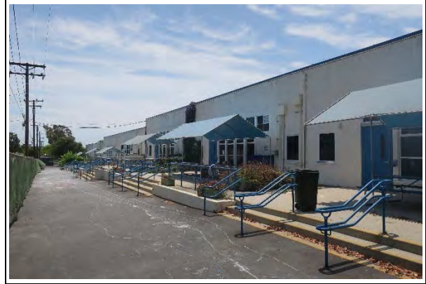
Building F, east façade, view south (ARG, 2021)
