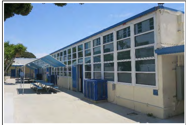
Building E, north façade, view east (ARG, 2021)
