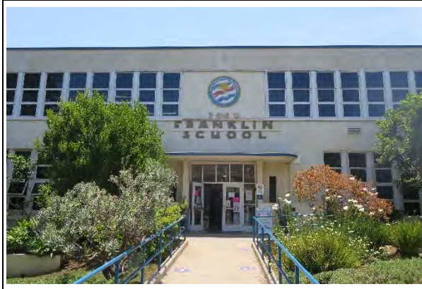
Building B, primary (north) façade, view southeast (ARG, 2021)
