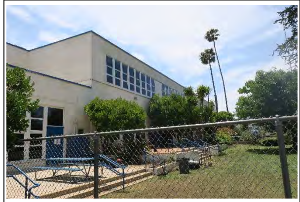
Building B, primary (north) façade, view west (ARG, 2021)
