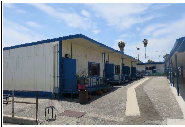
Portable buildings (ARG, 2021)
