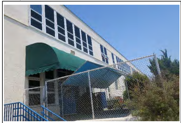
Building B, rear (south) façade, view north (ARG, 2021)
