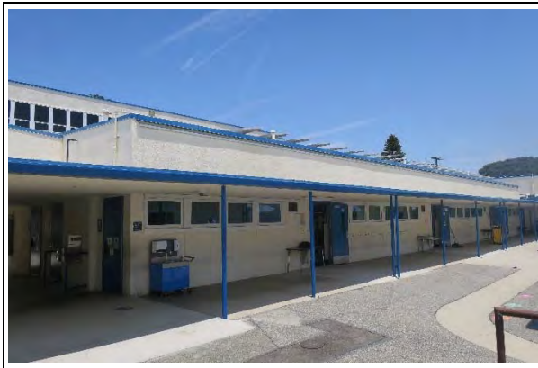
Building E, south façade, view northeast (ARG, 2021)
