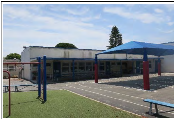
Building G, north façade, view southwest (ARG, 2021)
