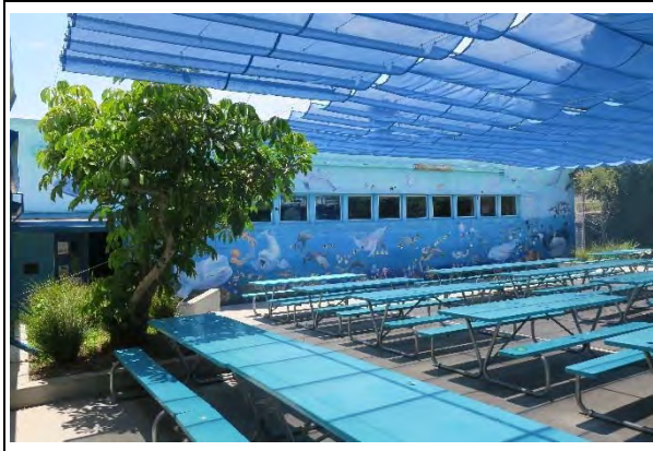
Building C, north façade, view southwest (ARG, 2021)
