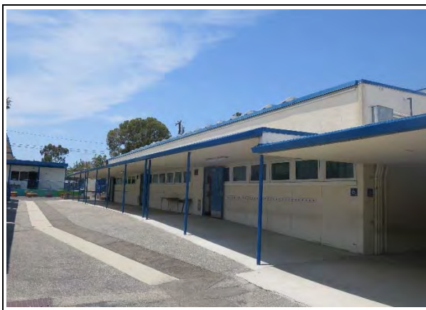
Building D, south façade, view northwest (ARG, 2021)
