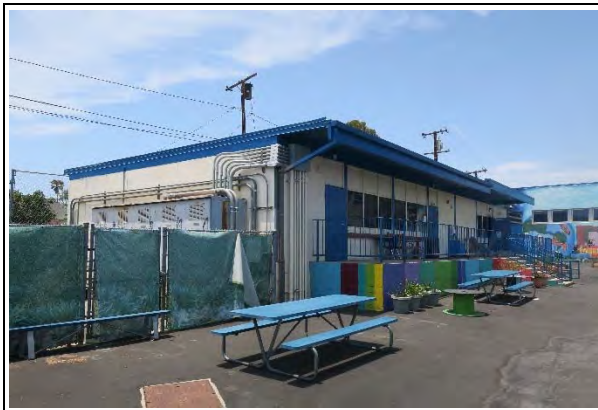
Portable buildings (ARG, 2021)
