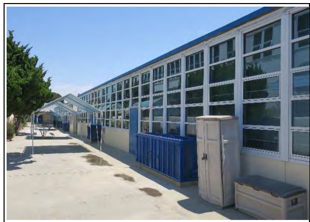
Building D, north façade, view east (ARG, 2021)
