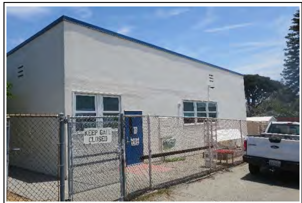
Building G, west façade as seen from 24 th Place, view east (ARG, 2021)
