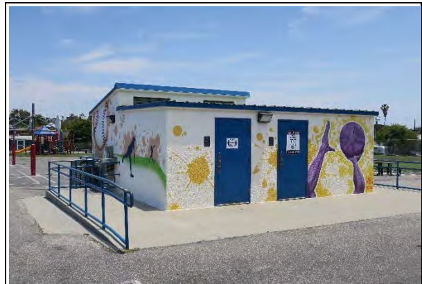
Ancillary restroom building at south end of campus, view southeast (ARG, 2021)
