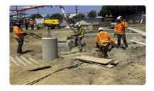
In the staff parking lot, base material was imported and graded, and crews drilled and formed light pole bases and tree well curbs. Structural work included bolting and welding for the bridge connection, fish scale panels, elevator hoist beam, and guide rails. NV5, an environmental consulting company, conducted air quality monitoring throughout all earthwork activities for compliance with Rule 1466.
