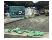
Administration Building Compacting road base in preparation for upcoming asphalt paving.
