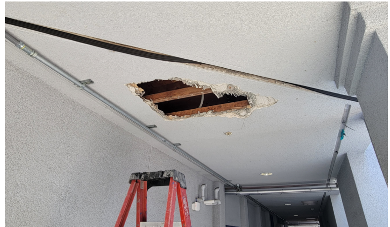
Photo 01: Opening in Existing Soffit
