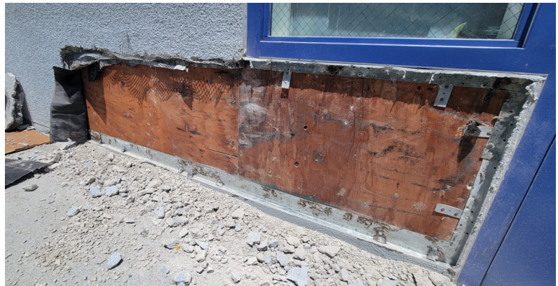
Photo 07: Room 415 Exposed Flashing
