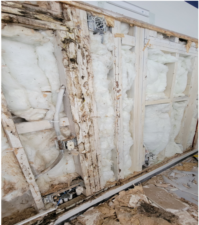
Photo 06: Room 415 Rotted Framing
