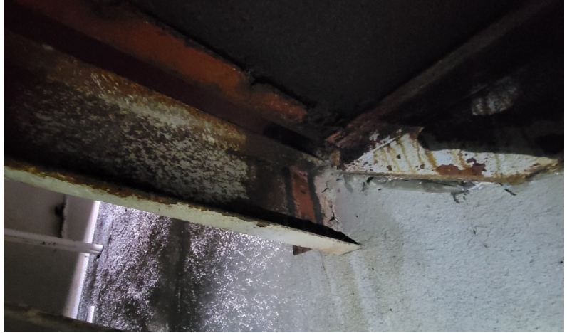
Photo 16: Exterior Stair Corrosion
