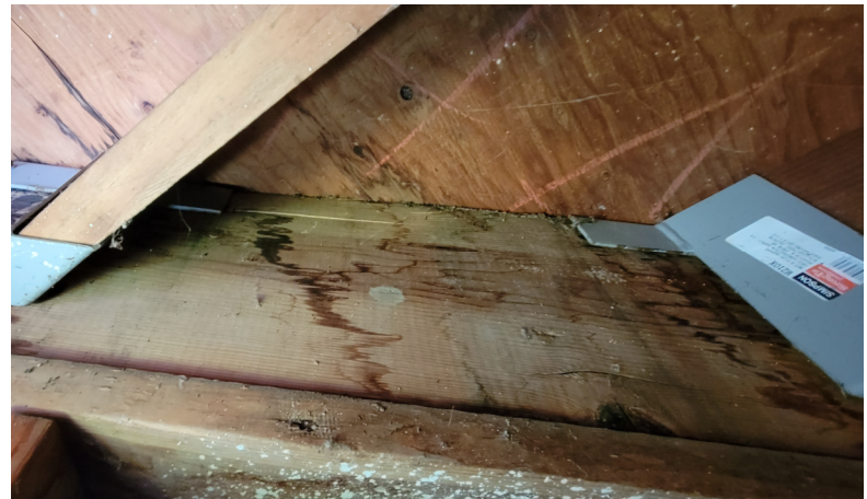
Photo 02: Damaged Beam at Existing Soffit
