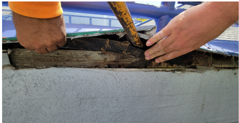
Photo 13: Parapet Plate Rotted
