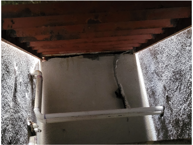
Photo 18: Exterior Stair Corrosion
