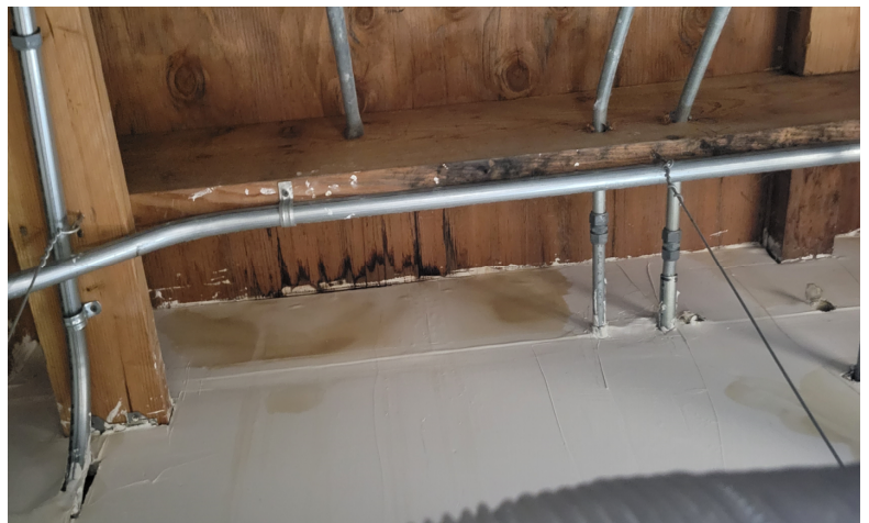
Photo 04: Room 210B Staining of Lumber
