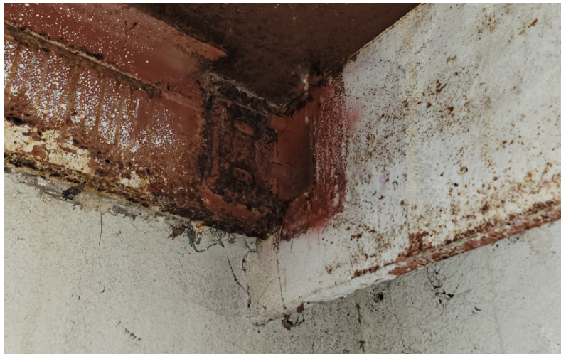
Photo 17: Exterior Stair Corrosion
