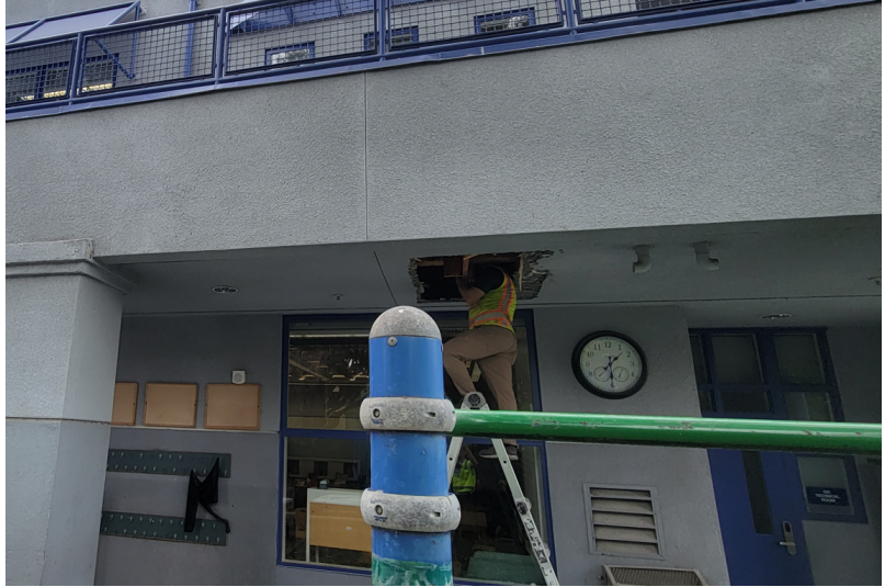
Photo 09: Soffit Removed at Room 405
