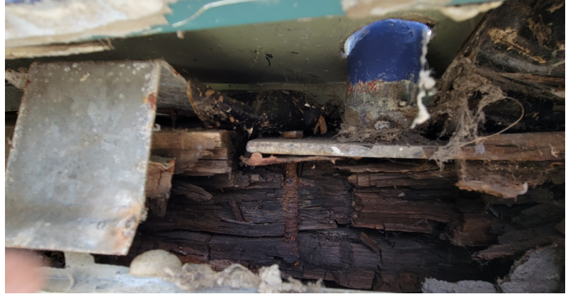
Photo 11: Parapet Plate Rotted
