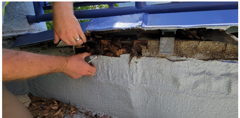
Photo 12: Parapet Plate Rotted
