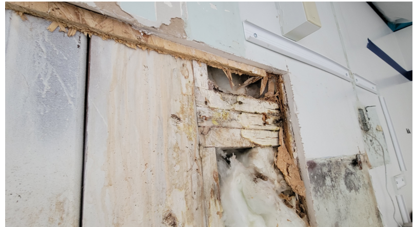
Photo 05: Room 415 Rotted Framing
