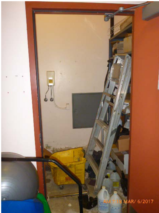
Photo #9: Overview of Custodial closet in hallway adj. Classroom 615
