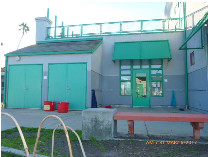
Photo #15: Overview of Classroom 600 exterior (west)
