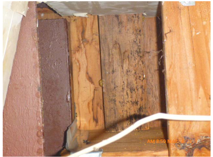
Photo 38: Close-up of staining on wooden beams
