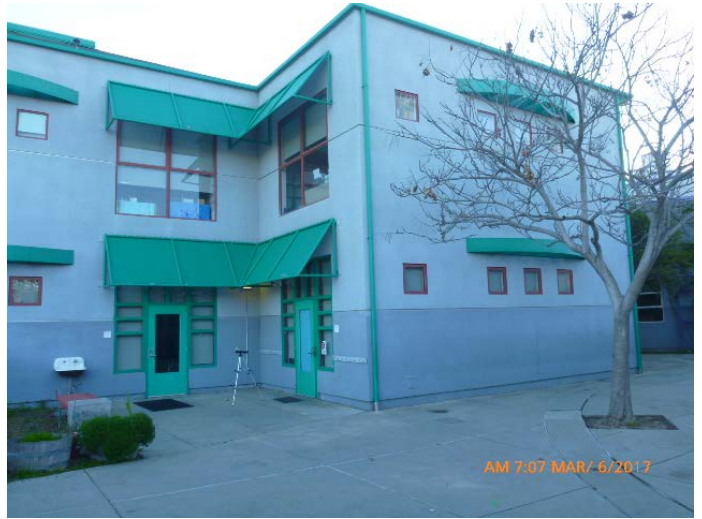
Photo #2: Overview of exterior of Classroom 615 (1 st floor)
