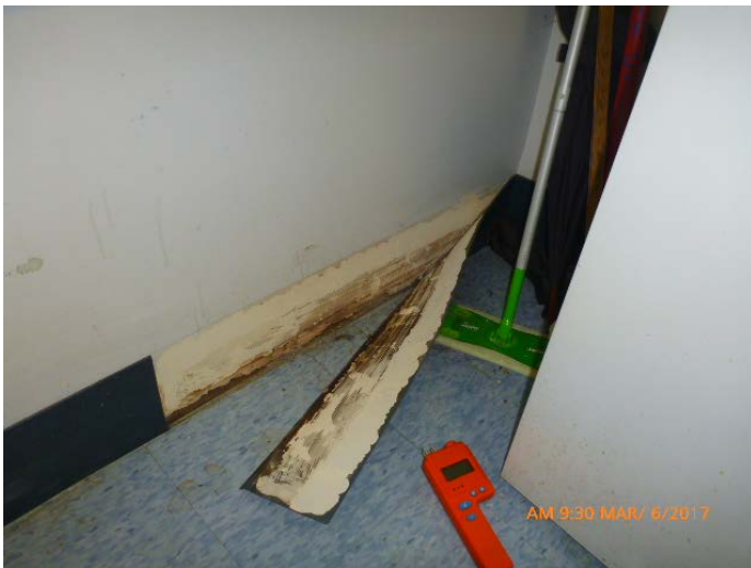
Photo 59: Overview of south wall adj. bathroom
