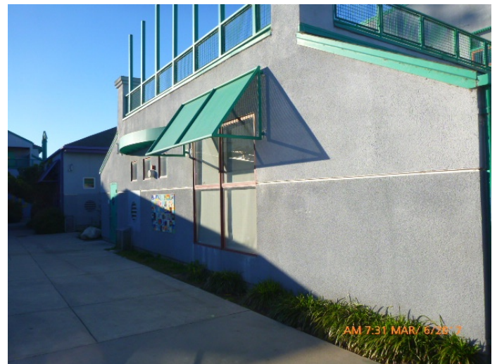
Photo #16: Overview of Classroom 600 exterior (north)
