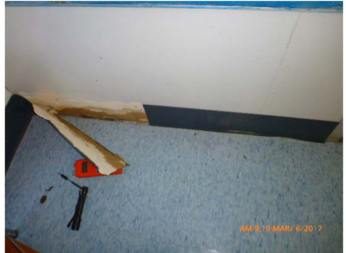
Photo 54: Overview of base of west wall
