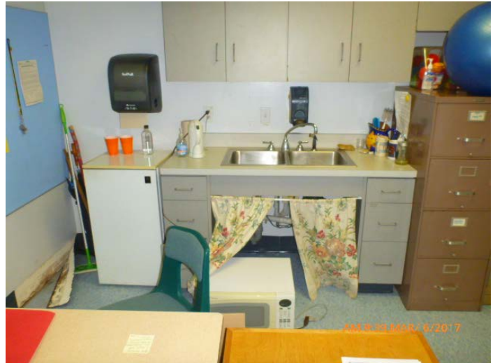
Photo 58: Overview of SW corner including sink cabinetry
