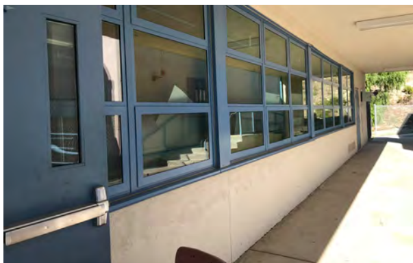
Typical door and storefront window system.
