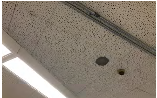
Typical gluedown ceiling tile.
