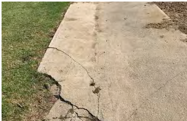
Broken Drainage - Concrete Ditch
