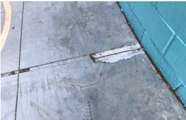
Concrete Cracking
