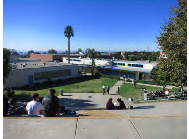
View of major grade change at Malibu High School Photo by LPA
