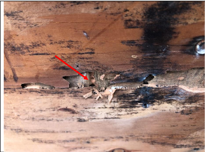
Photo 266: Insect damage was observed on the exterior side of the exterior plywood sheathing after the building paper had been removed.
