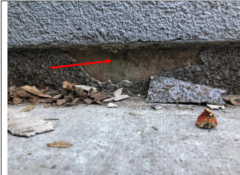
Photo 230: Cracked and broken cement plaster texture coat was observed at numerous curb locations.
