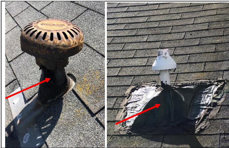
Photo 162: Corroded vent stacks with deficient flashing were observed in several locations.
