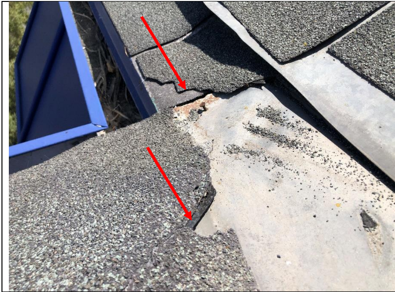
Photo 159: Shingle tabs were observed on the roof deck, damages on the roof, or were missing altogether.
