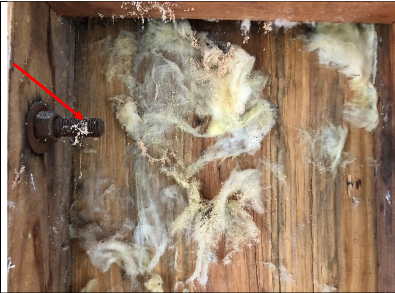
Photo 283: Some water staining and corrosion were observed inside the west wall of room 400.
