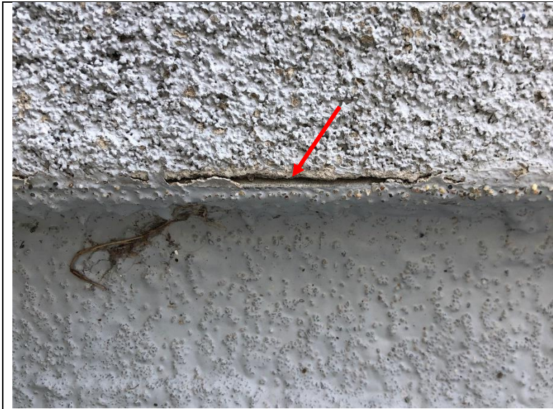
Photo 26: Deficiencies in the cement plaster were observed at the base of the walls
