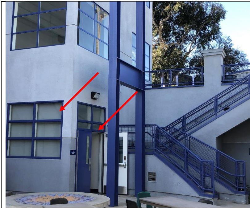
Photo 98: Hollow metal frame assemblies.
