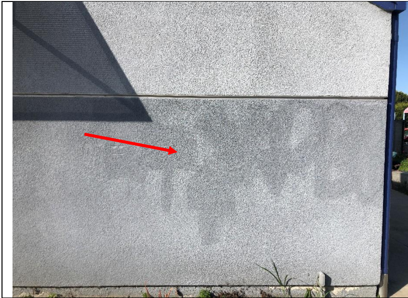
Photo 36: New paint had been applied on the cement plaster.
