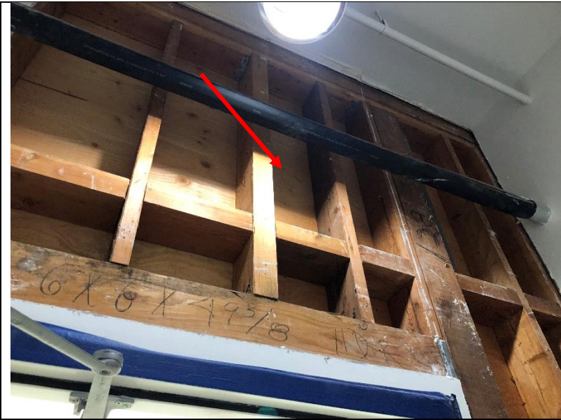
Photo 292: Interior finishes and insulation were removed above the door to room 513.
