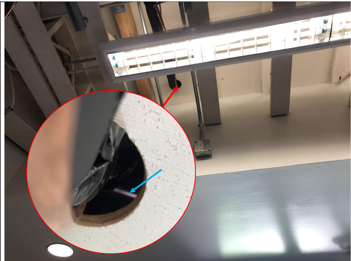
Photo 182: Exterior light was visible through the wall system over the east entrance to the library. The location is a reported leak site.
