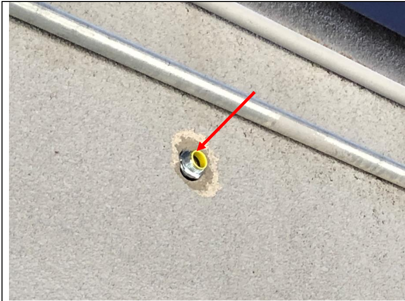
Photo 10: An open penetration in the cement plaster assembly with no visible sealant.
