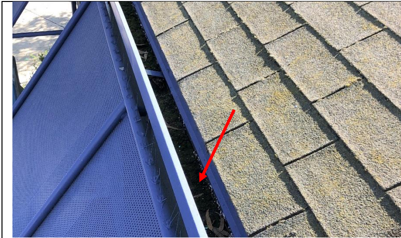
Photo 156: A gutter on building B was filled with granules and debris.
