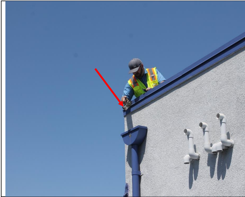
Photo 152: DTR clearing a blocked downspout.
