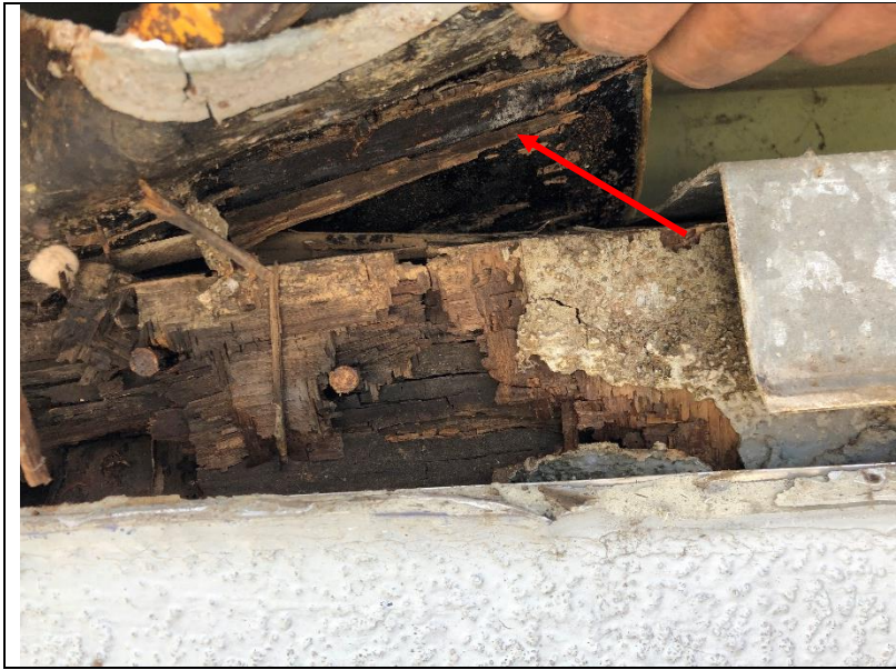
Photo 341: The self-adhered sheet membrane was not adhered to the substrate and numerous open seams were observed in the installation of the product.
