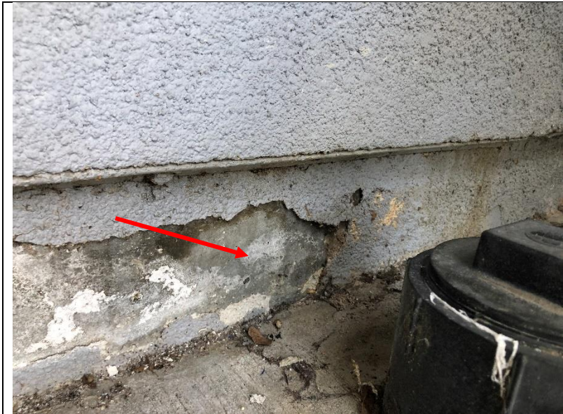
Photo 231: Cracked and broken cement plaster texture coat was observed at numerous curb locations
