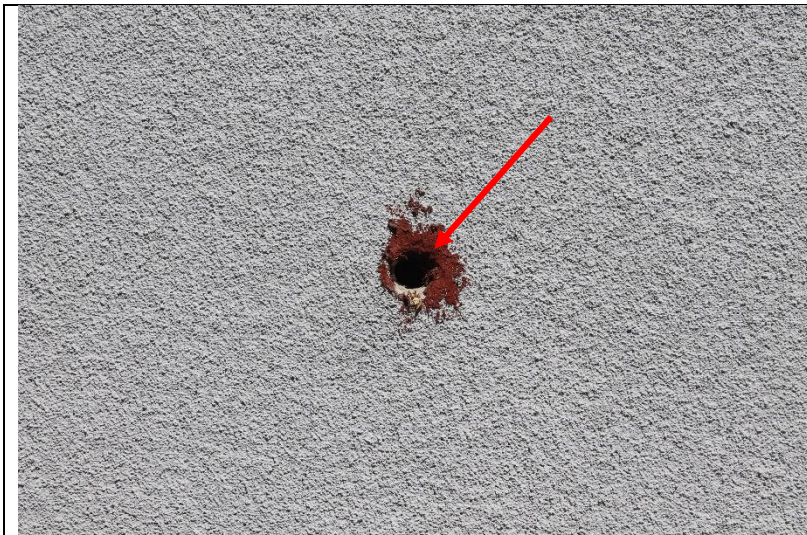
Photo 16: An abandoned penetration in the cement plaster assembly with what appears to be fire caulk (rather than a weather sealant) applied.
