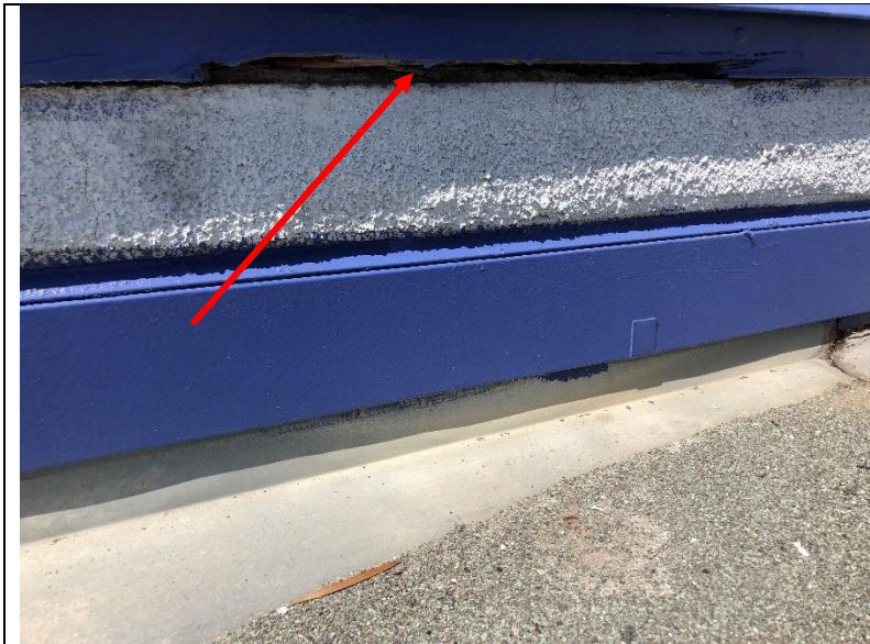
Photo 176: Dry rot and suspected insect damage at the wooden roof trim.
