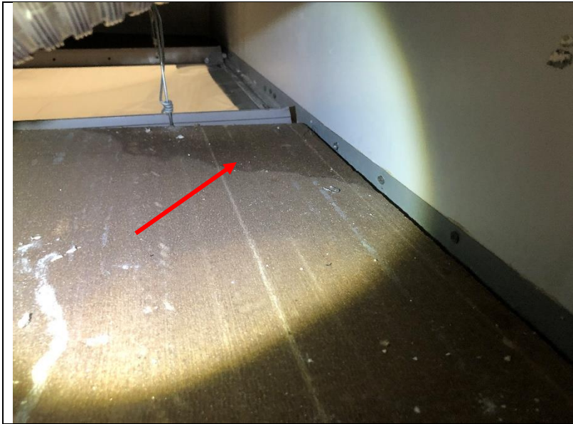
Photo 307: Staining was observed on the top of the ceiling panels.
