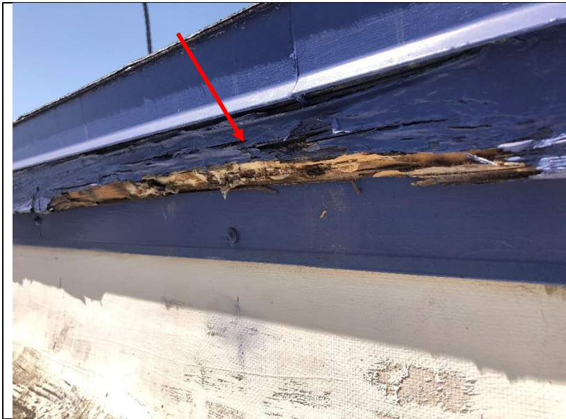
Photo 173: Dry rot and suspected insect damage at the wooden roof trim.
