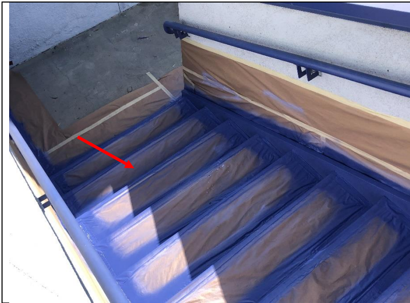
Photo 67: The stairs were masked off during painting.
