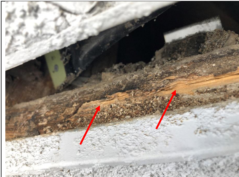
Photo 322: Insect damage on wood surfaces at the bottom of the building A expansion joint after the compressed foam had been removed.
