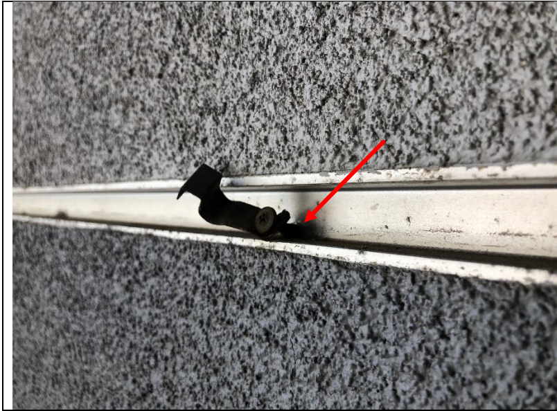
Photo 09: An un-sealed penetration in a cement plaster control joint.
