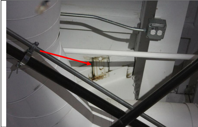
Photo 192: Water stains above the recessed ceiling in the multipurpose room.
