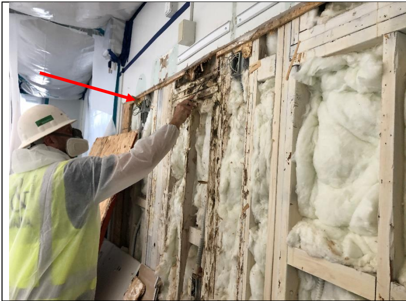
Photo 253: Martin & Associates making observations of wood rot and deterioration to the south wall of room 415.
