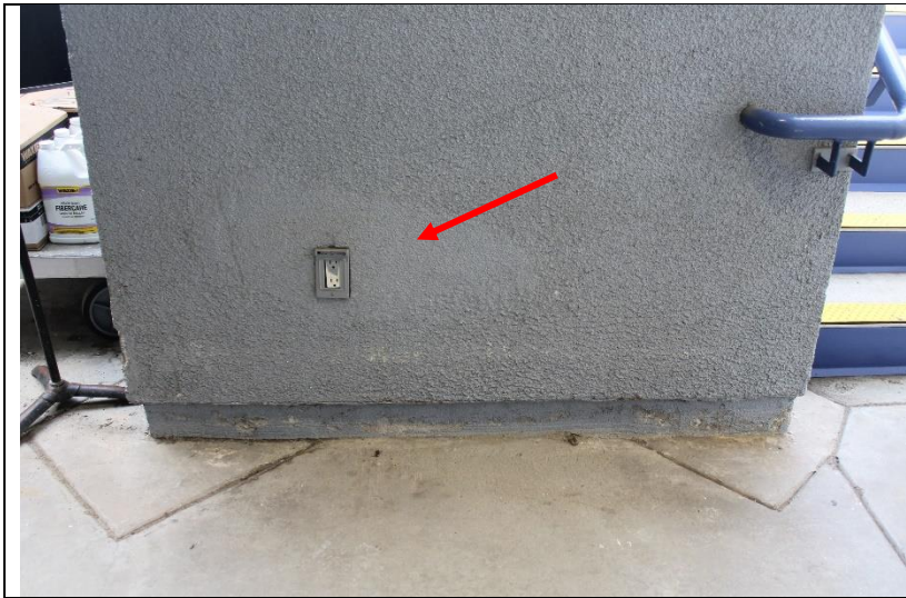
Photo 33: New paint had been applied over repairs to the cement plaster
