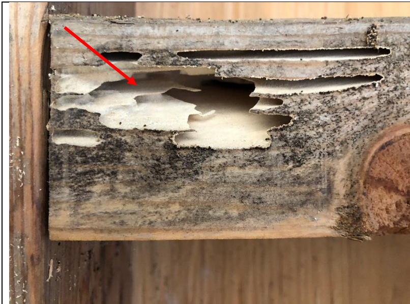
Photo 281: Insect damage at blocking inside the west wall of room 400.
