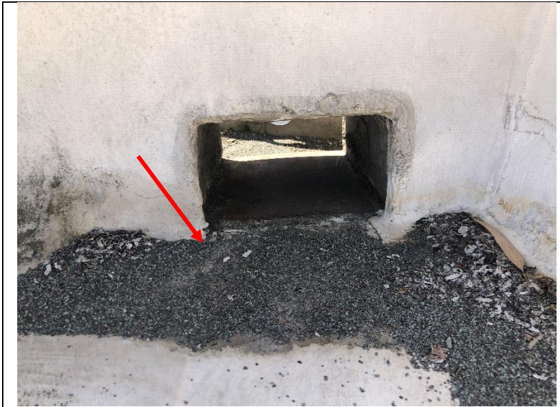
Photo 154: Granule loss was significant at all of the asphalt shingle roofs.
