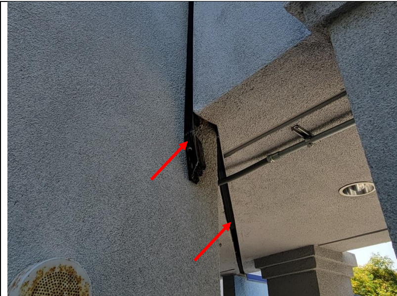
Photo 319: The compressed foam at the bottom of the expansion joint was loose and had fallen away at some locations. Photo courtesy of JAMA
