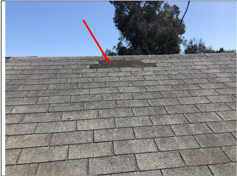
Photo 160: Shingle tabs were observed on the roof deck, damages on the roof, or were missing altogether.
