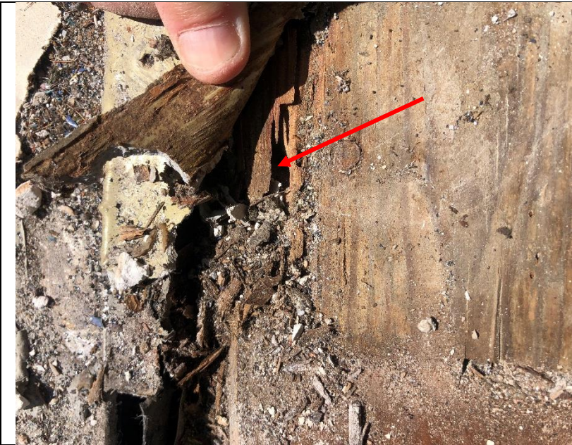
Photo 79: Dry rot, water damage, and suspected insect damage at the threshold of classroom 480
