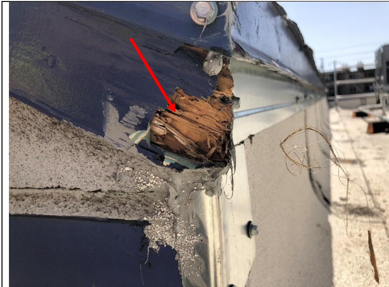
Photo 175: Dry rot and suspected insect damage at the wooden roof trim.
