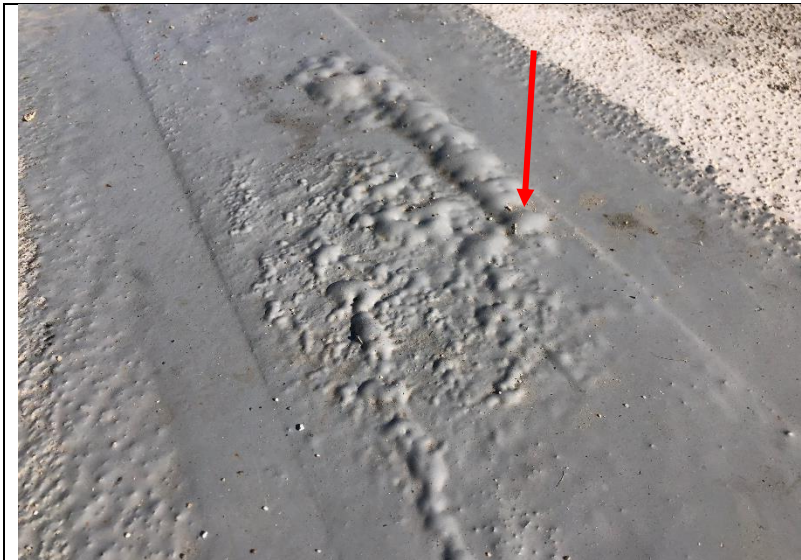
Photo 52: Blistering at a traffic coating patch indicating trapped water and/or coating failure.
