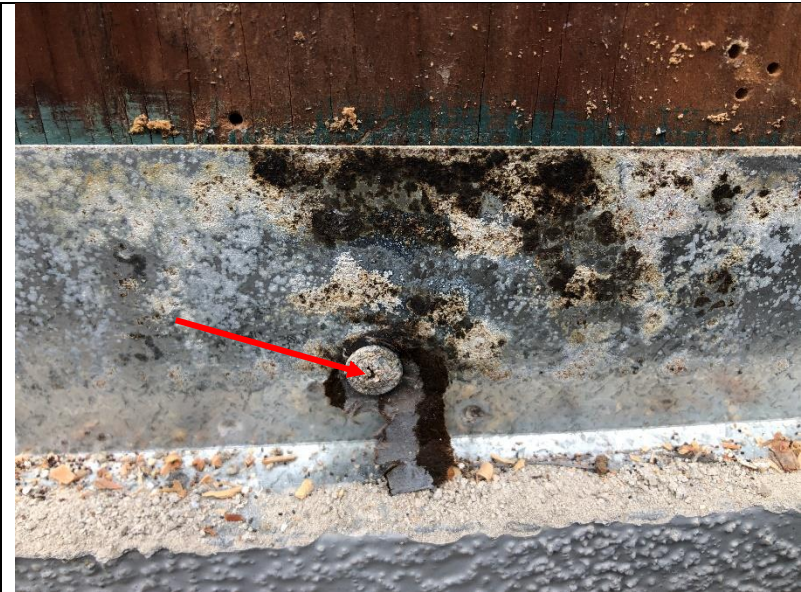
Photo 267: Fasteners at the top flange of the z-flashing outside of room 480 penetrated the building paper.
