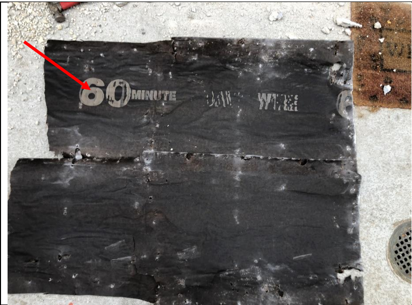
Photo 265: Two layers of 60-minute building paper were removed from behind the cement plaster assembly at the exterior of building B room 480.
