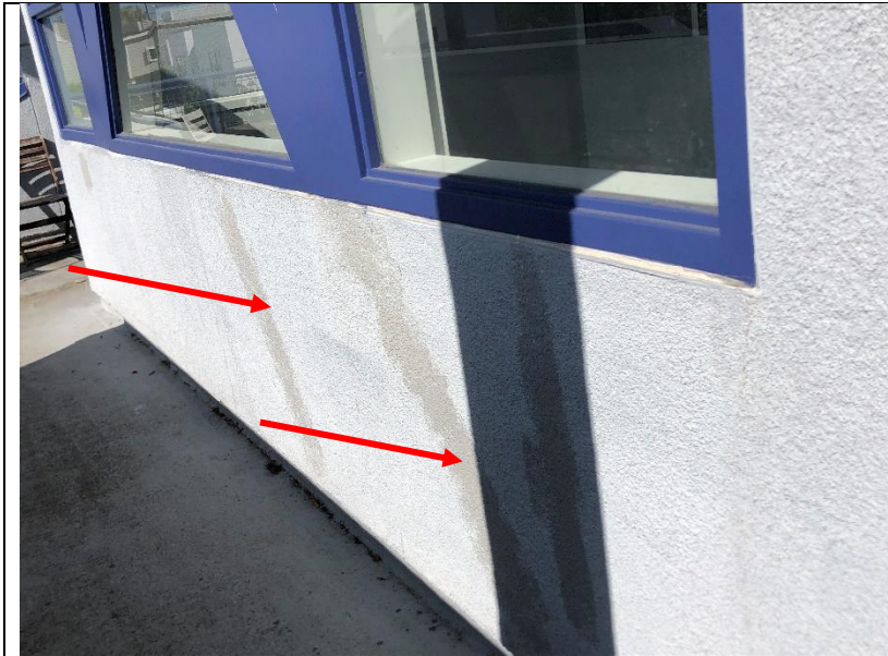
Photo 35: New paint had been applied on the cement plaster.
