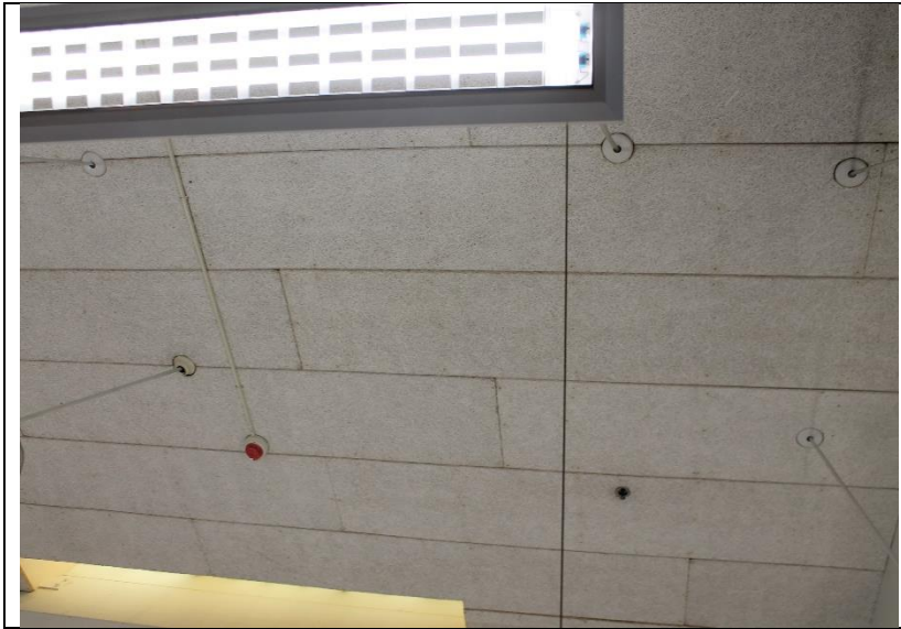
Photo 218: Acoustical panels on the ceiling of the classrooms in building D.
