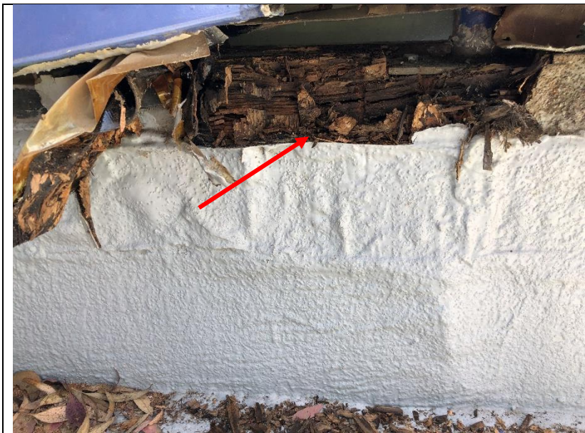
Photo 346: Wood rot and deteriorated wood materials at the handrail curb under the coping cap outside room 400.
