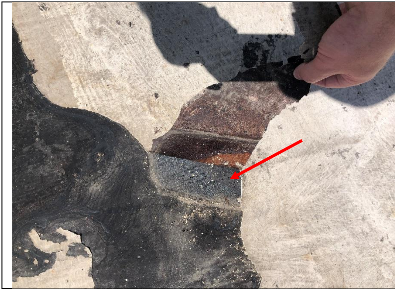
Photo 128: A coating failure at the BUR roof over the multipurpose room.
