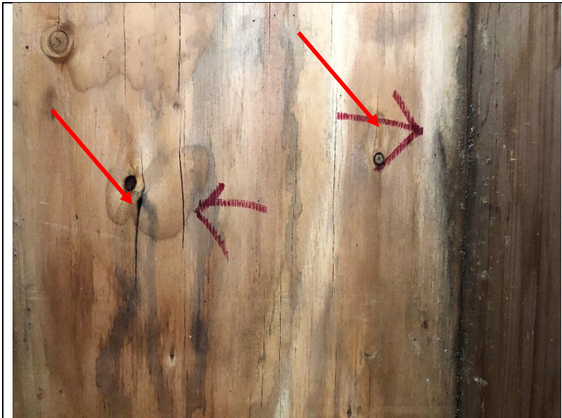
Photo 278: Delamination and water staining were observed on the exterior sheathing plywood on the south wall of room 400.
