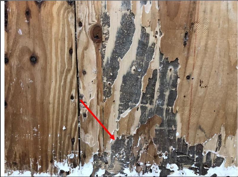
Photo 276: Insect damage at the interior shear wall plywood on the south wall of room 400.
