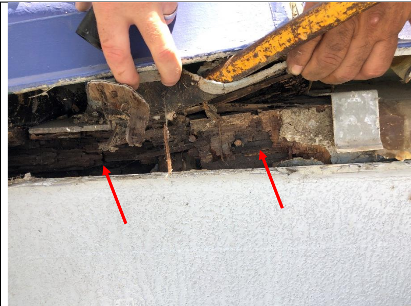
Photo 339: Wood rot and deteriorated wood materials were observed under the coping cap at the handrail curbs.
