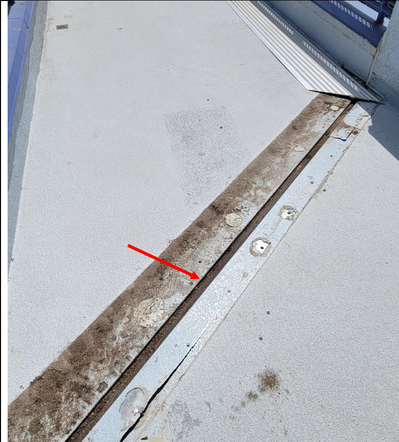
Photo 318: The expansion joint above the DT location at the walkway between the administration and library spaces at building A. The metal cover was removed to allow for observations. Photo courtesy of JAMA
