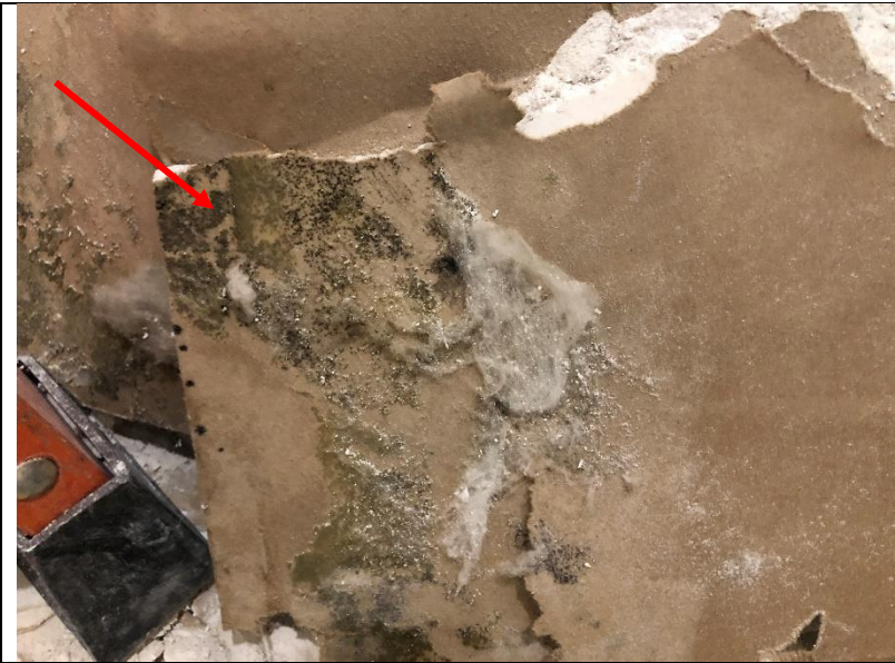
Photo 295: Biological growth was observed on the back of the interior gypsum board when it was removed from the wing wall outside the entry of room 513.
