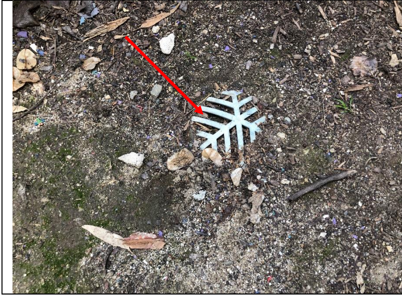
Photo 224: A surface drain at a landscaped area blocked by landscaping materials.
