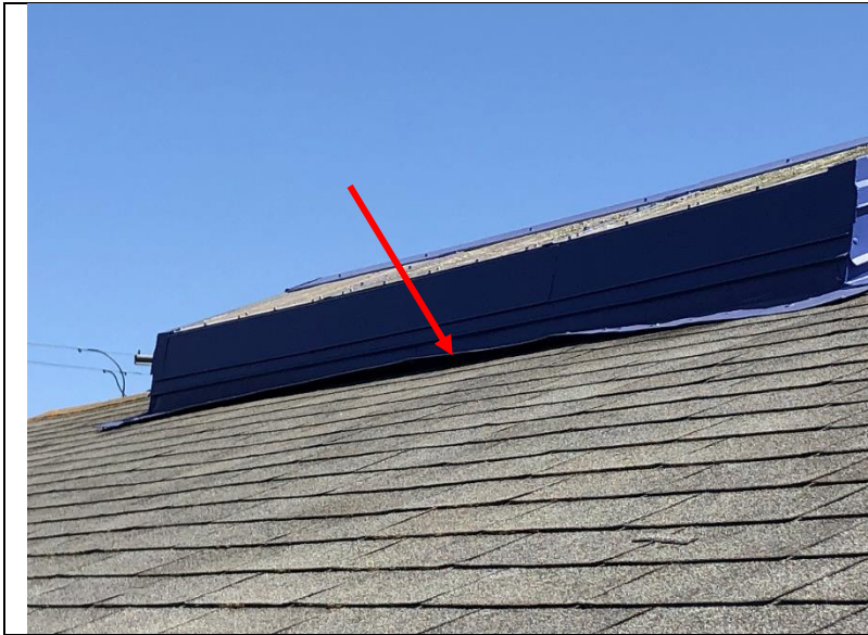
Photo 172: Sheet metal skirt flashing at the skylights was not flat and flush to the roof.
