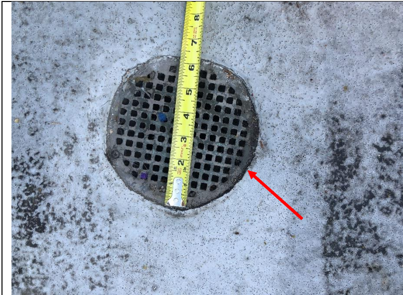
Photo 59: A 6-inch round drain cover over a 2-inch pipe.
