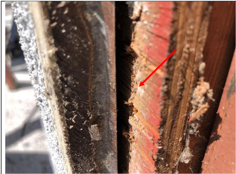
Photo 90: Delamination of the exterior plywood sheathing was observed after the hollow metal frames were removed. No flashing, waterproofing, or weather resistive barrier were observed at this location.
