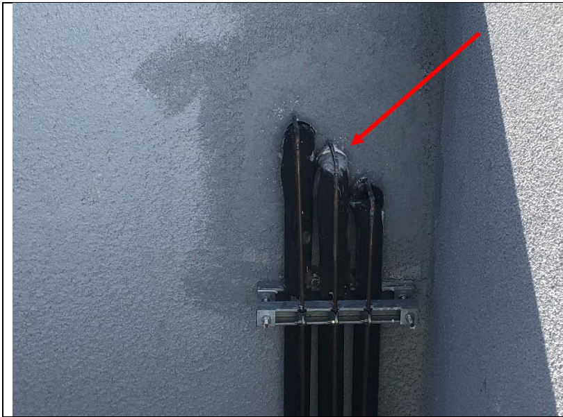
Photo 11: Penetrations in the cement plaster assembly.
