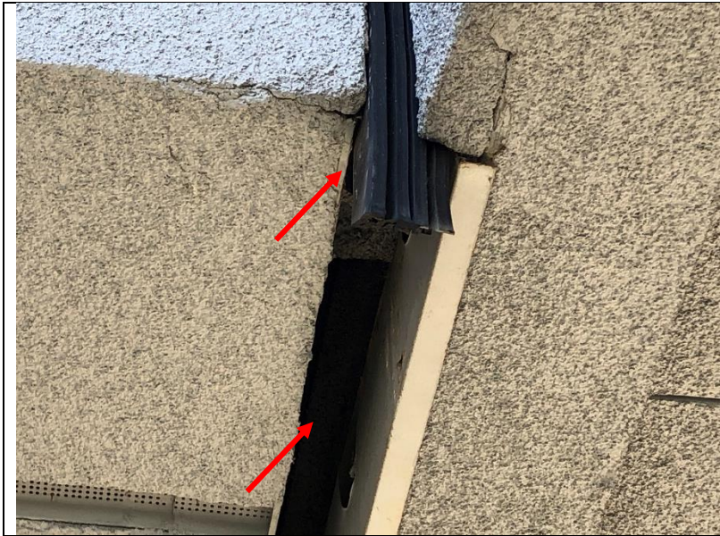
Photo 320: The compressed foam at the bottom of the building A expansion joint was loose and had fallen away at some locations.
