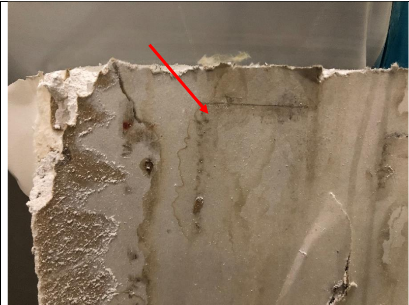
Photo 296: Biological growth was observed on the back of the gypsum board when it was removed from the wing wall outside the entry of room 513.
