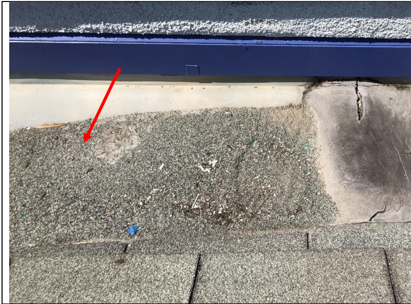
Photo 155: Granule loss was significant at all of the asphalt shingle roofs.
