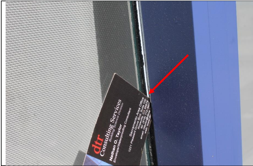
Photo 111: A glazing gasket failure at the perimeter of the glazing at an aluminum-framed window.
