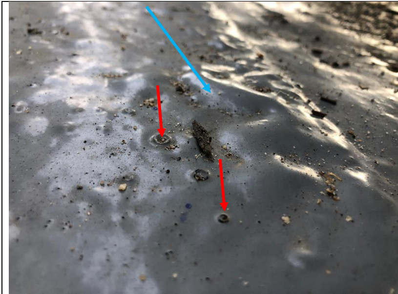
Photo 51: Blisters (blue arrow) and pinholes (red arrows) in a traffic coating patch indicating trapped water and/or coating failure.
