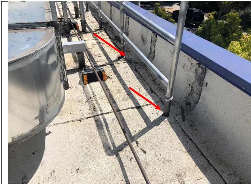
Photo 141: Lead flashings were installed at the fall protection rail at the newly installed granulated cap sheet on the roof of the multipurpose room.
