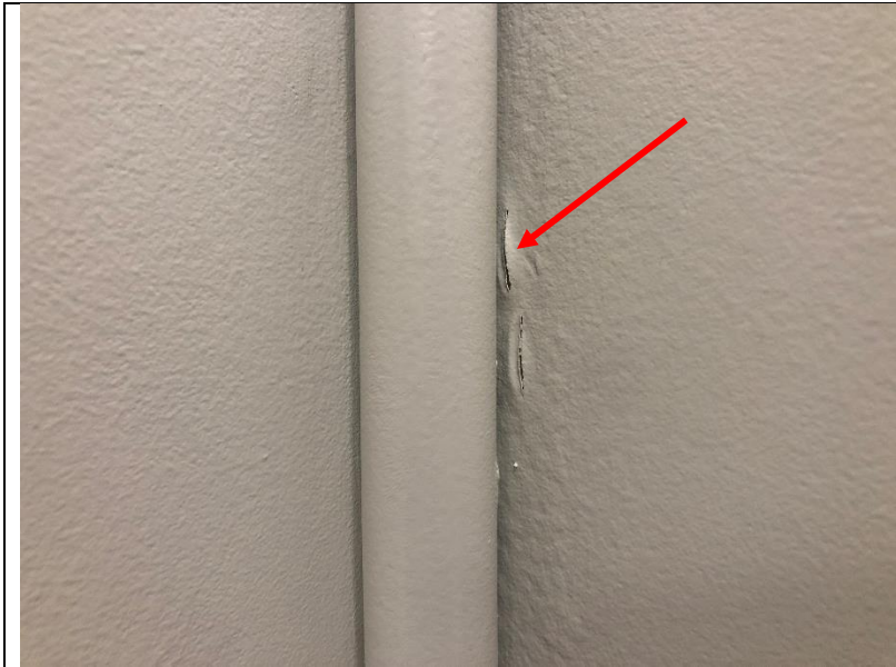
Photo 325: Close view of water damage at the interior corner of the library.
