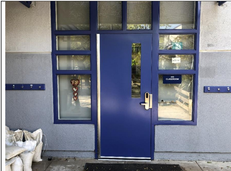
Photo 97: A hollow metal frame door/window assembly.
