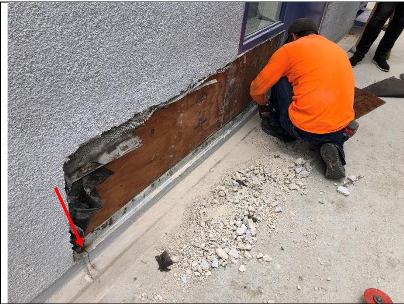
Photo 268: The contractor cut vertically through the z-flashing to allow for it to be pulled down and removed from the building.
