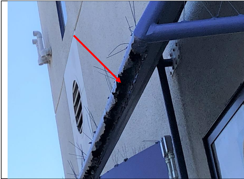
Photo 228: Corrosion at metal awnings was observed at several locations.
