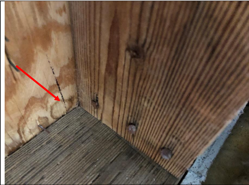
Photo 287: Evidence of abrasion and previous mold remediation were visible inside the west wall of room 400.
