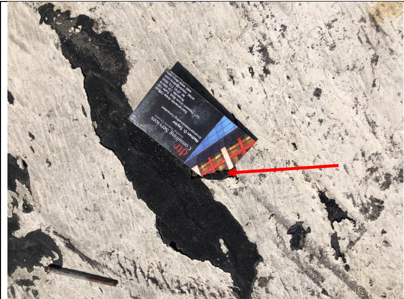
Photo 131: A hole in the BUR roof over the multipurpose room.
