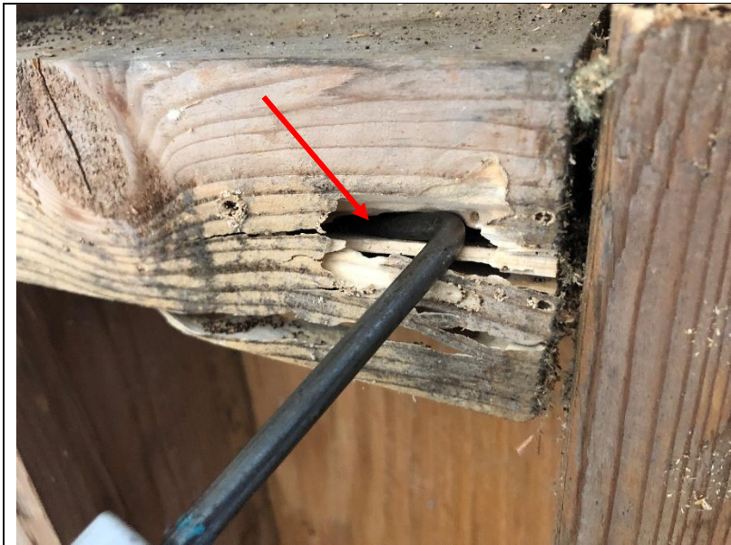
Photo 282: Insect damage at blocking inside the west wall of room 400.
