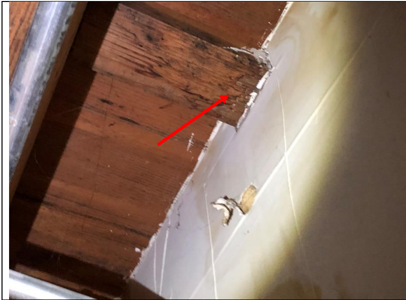
Photo 303: Staining is visible at several locations adjacent to the exterior wall overhead in room 210B.
