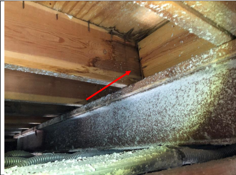
Photo 336: Staining was observed at the joists under the walkway outside room 415.
