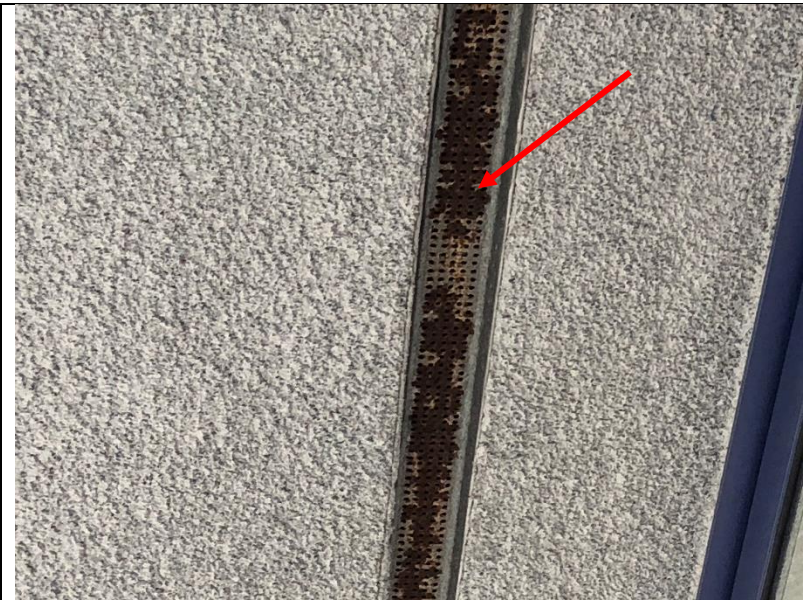
Photo 333: Much of the soffit venting track that ran parallel to building B was corroded. The location is below the water stains observed at the joist hangers and the ledger against the building.
