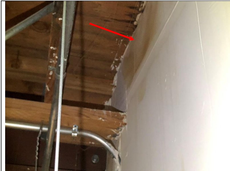
Photo 304: Staining visible at several locations adjacent to the exterior wall.
