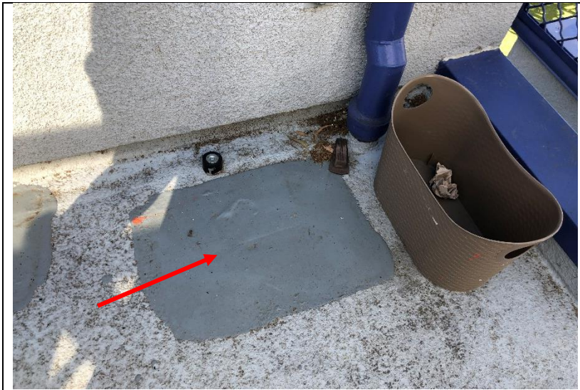
Photo 50: A patch in the traffic coating.
