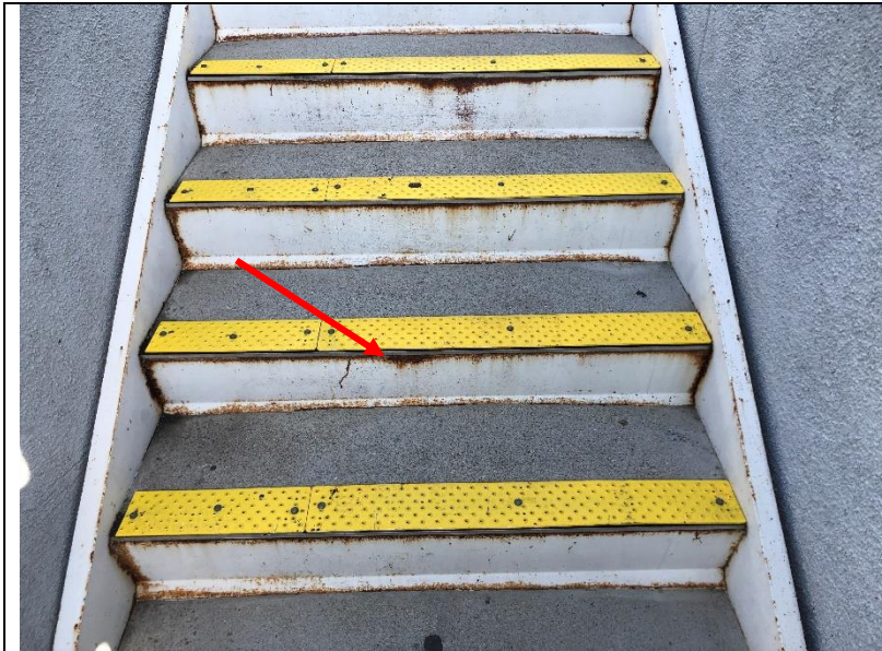
Photo 65: Corrosion was observed at the stairs prior to repainting.
