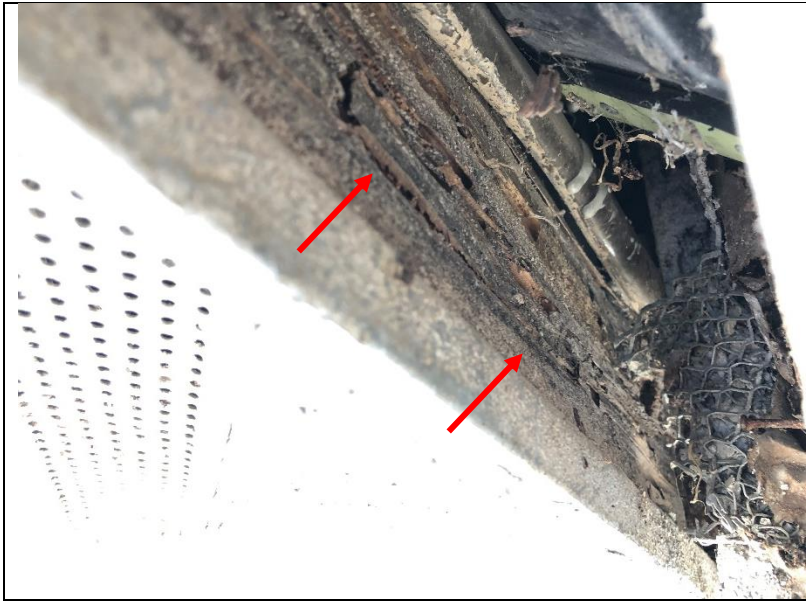
Photo 321: Insect damage on wood surfaces at the bottom of the expansion joint after the compressed foam had been removed.
