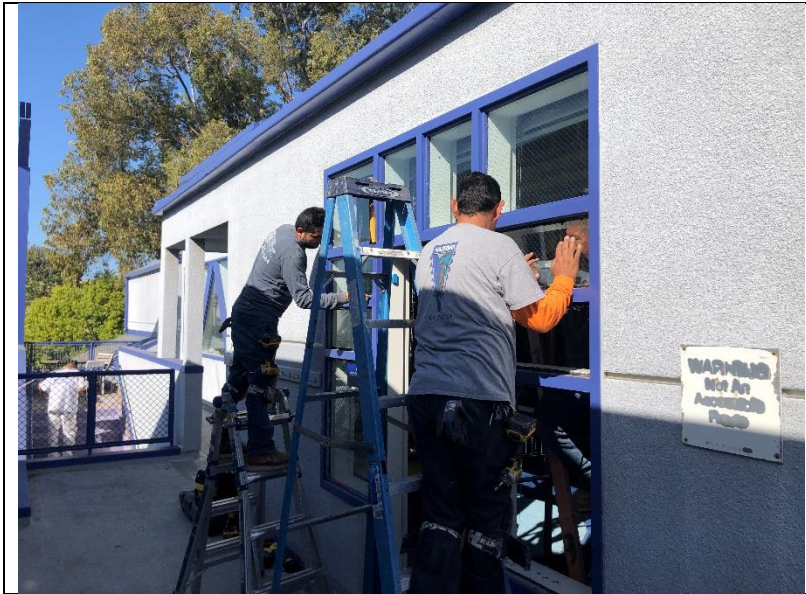
Photo 69: The hollow metal frame was being removed at Classroom 480.
