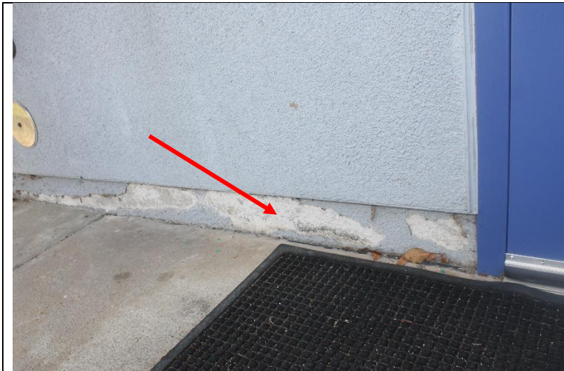
Photo 232: Cracked and broken cement plaster texture coat was observed at numerous curb locations
