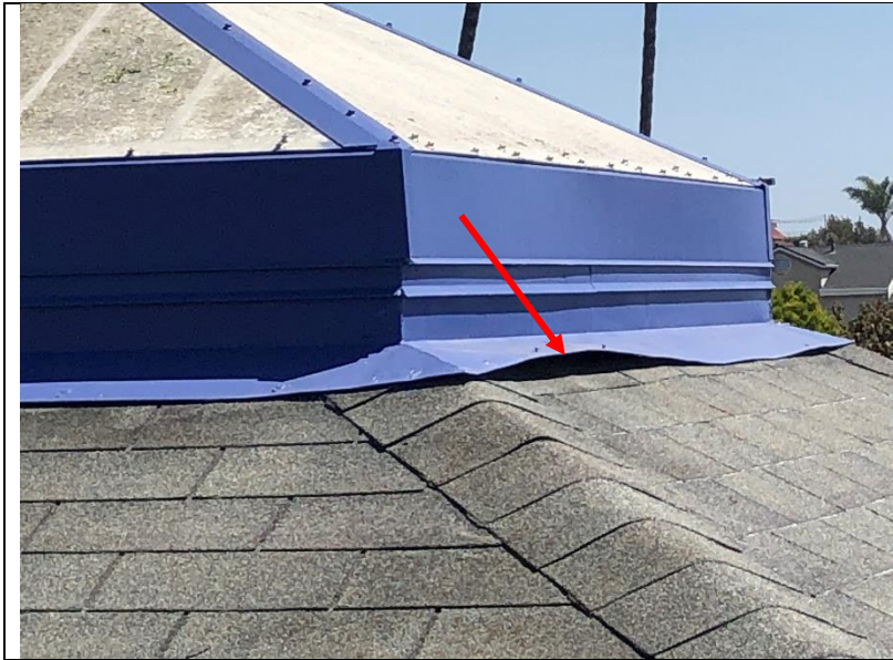
Photo 171: Sheet metal skirt flashing at the skylights was not flat and flush to the roof.
