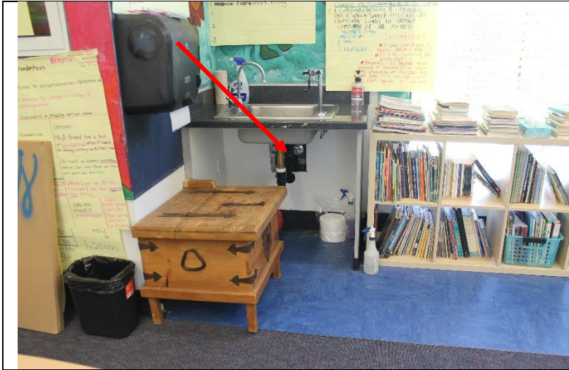
Photo 210: Interior finishes had been removed at two classrooms in building D prior to the DTR site assessment, in an effort to address a leak at this location.
