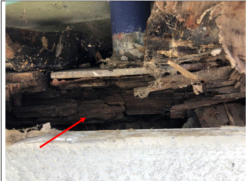
Photo 340: A void was observed under the coping cap outside room 400 at one of the handrail anchor plates where the wood structure had deteriorated.
