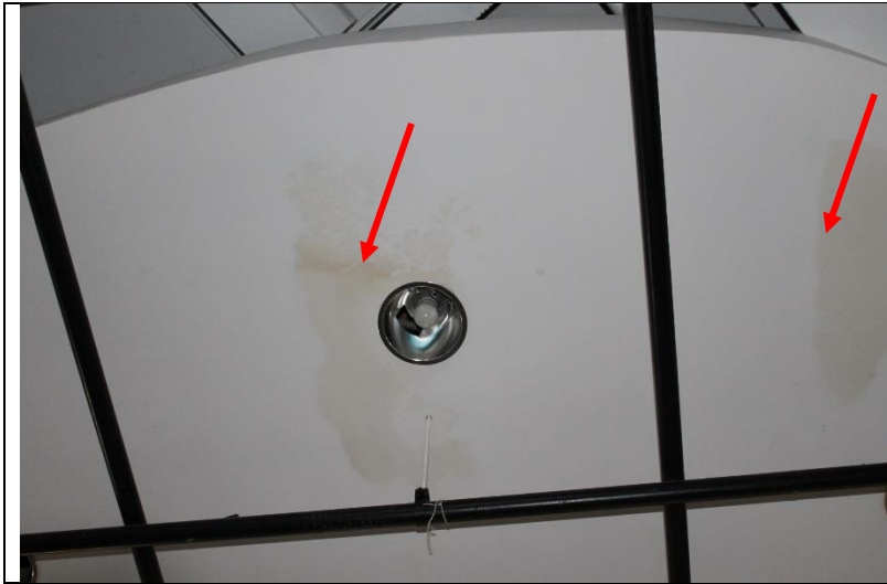
Photo 191: Water stains on the recessed ceiling in the multipurpose room.
