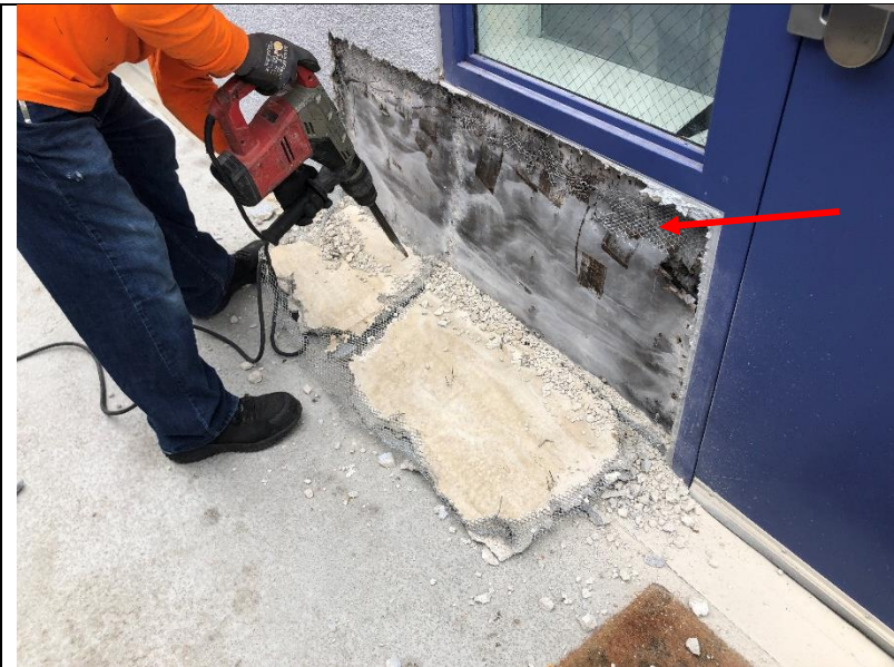
Photo 264: The contractor removed exterior cladding from the wall outside of classroom 480.
