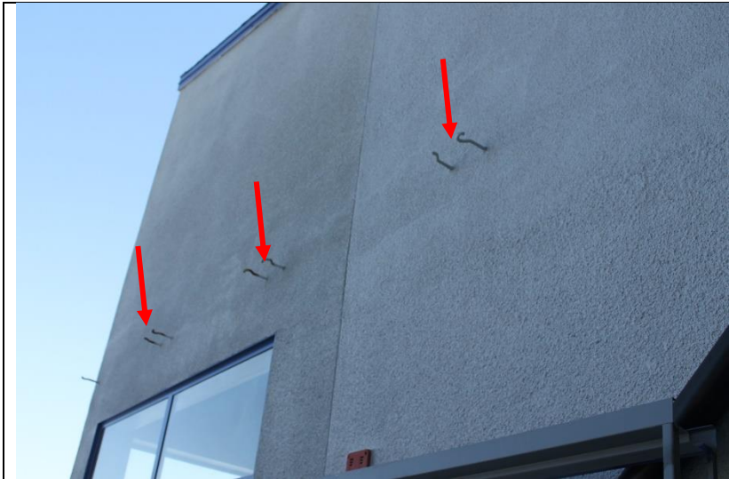
Photo 21: Hook anchor penetration in the cement plaster assembly
