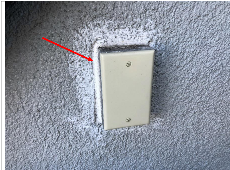
Photo 14: A penetration in the cement plaster assembly with a new sealant application.
