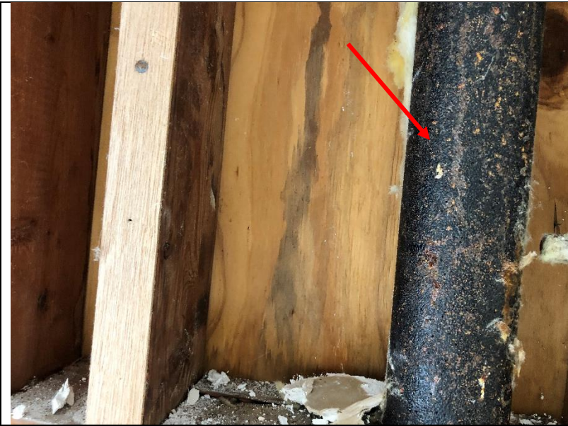
Photo 284: Some corrosion was observed on the drain pipes inside the west wall of room 400. The pipes were not wrapped in insulation.
