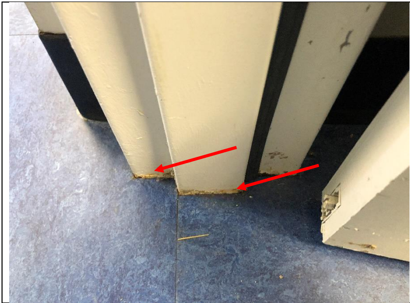
Photo 209: Corrosion at the bottom of the door jamb at Room 403 Teachers' Prep.
