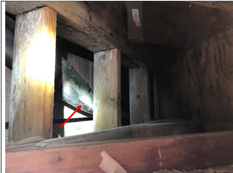
Photo 323: The drainage assembly under the expansion joint was hanging loose and no longer attached to the bottom of the expansion joint assembly.
