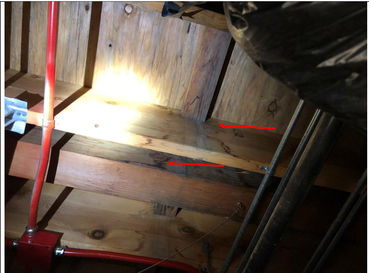
Photo 205: Water damage and staining above the ceiling tiles in room 205 Teacher's Prep.
