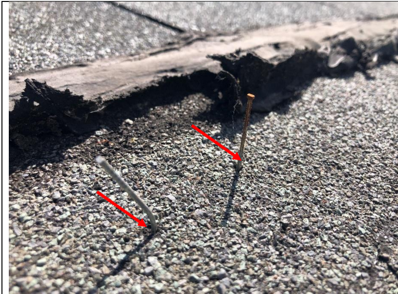
Photo 151: Staples and nails were observed at the mastic swath.
