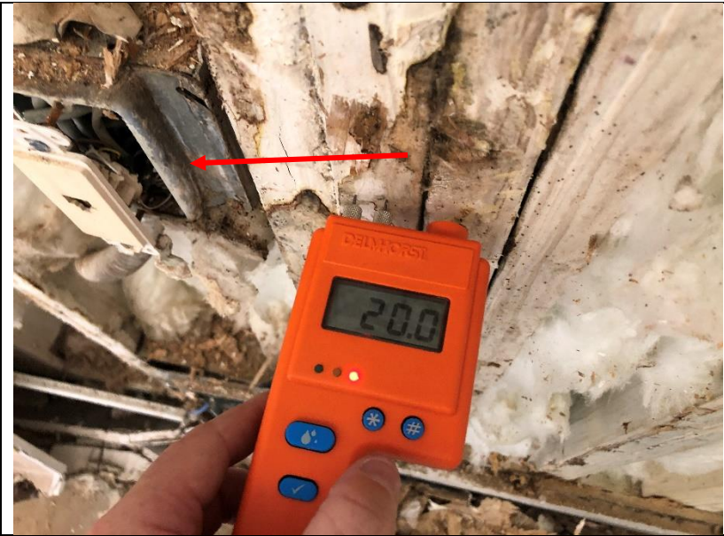
Photo 252: Corrosion and water damage were observed at several electrical junction boxes and along electrical conduits. Moisture reading at an adjacent wood stud was high (20.0 percent).
