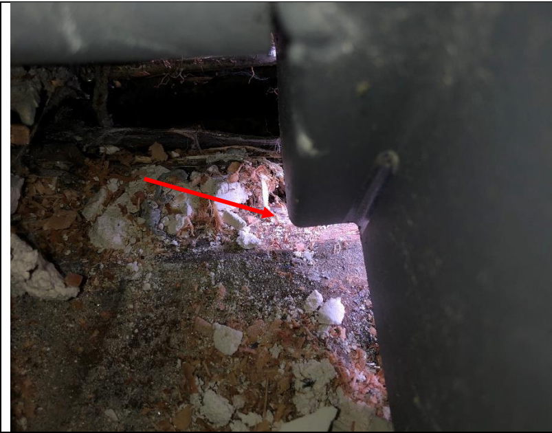
Photo 263: Exterior light is visible in this closer view of the base of the room 480 hollow metal door frame (viewed from the interior).
