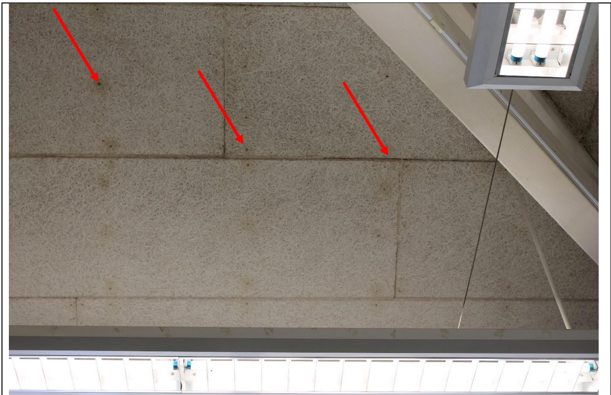
Photo 219: Water staining at the acoustical panels on the ceiling of the classrooms in building D.
