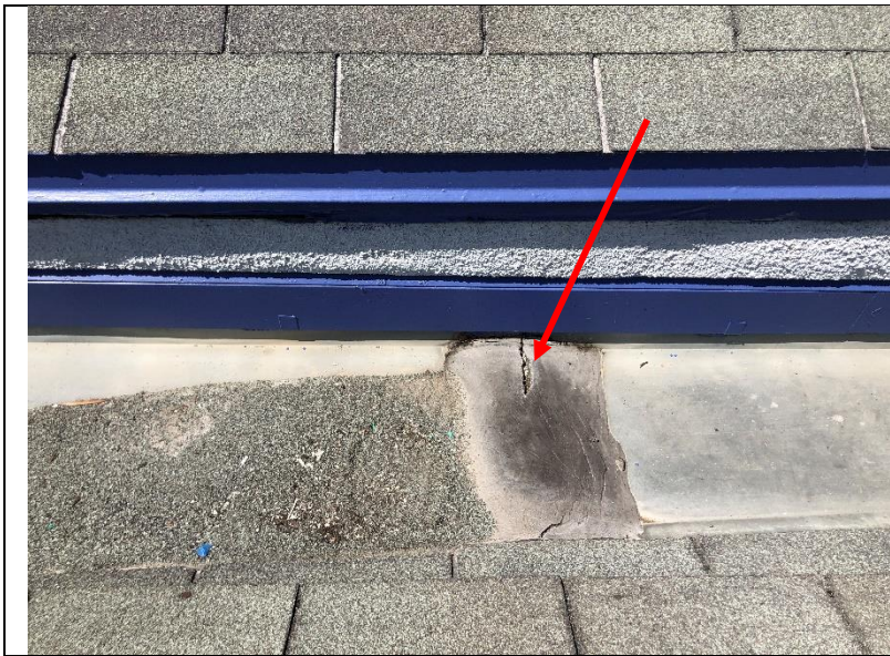
Photo 166: A black mastic had been applied to the sheet metal along a roof-to-wall valley. The mastic was cracked and had failed.
