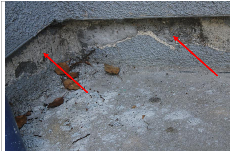
Photo 229: Cracked and broken cement plaster texture coat was observed at numerous curb locations
