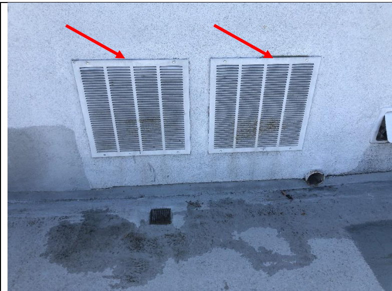
Photo 182: Exterior light was visible through the wall system over the east entrance to the library. The location is a reported leak site.
