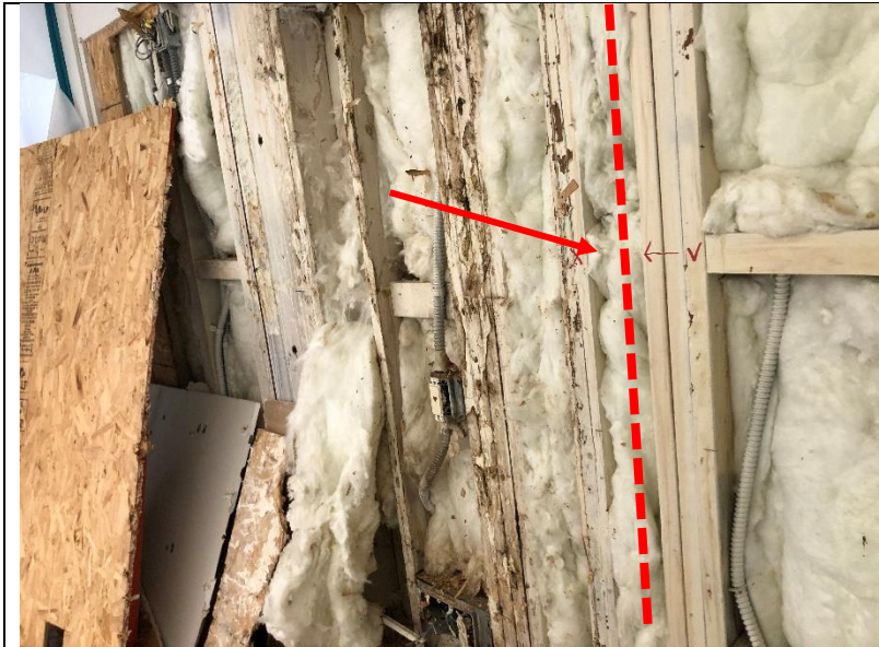
Photo 255: Another view showing the change between damaged and undamaged areas on the south wall of room 415.
