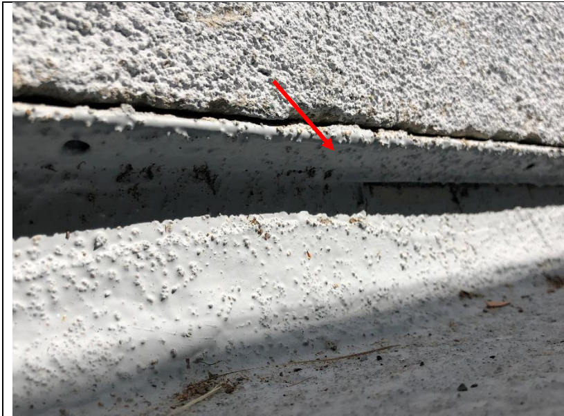
Photo 47: The traffic coating lapped up onto the weep screed with some of the weep holes blocked.
