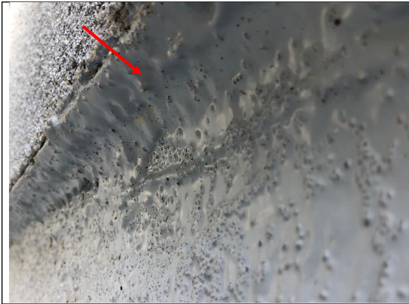
Photo 49: The traffic coating lapped up onto the weep screed. No weep holes were visible at this location.
