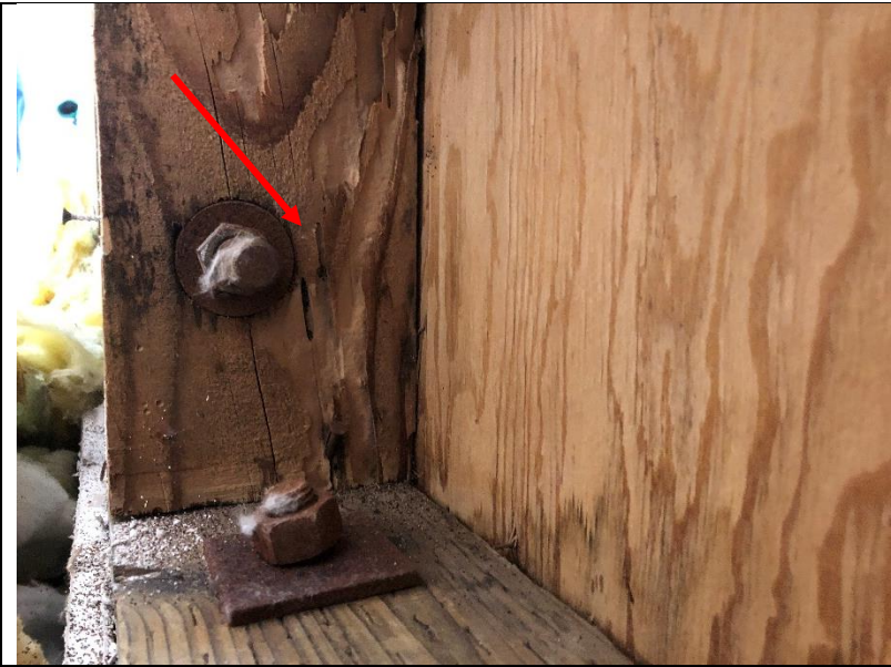
Photo 288: Evidence of abrasion and previous mold remediation were visible inside the west wall of room 400.
