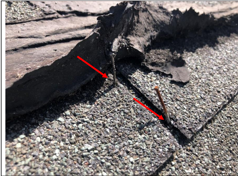
Photo 150: Staples and nails were observed at the mastic swath.
