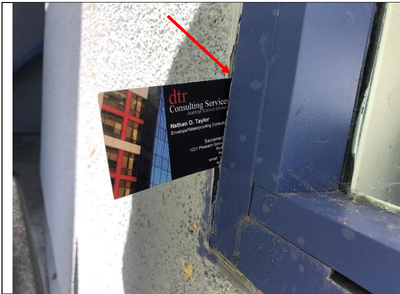
Photo 112: A sealant failure at the perimeter of an aluminum-framed window.
