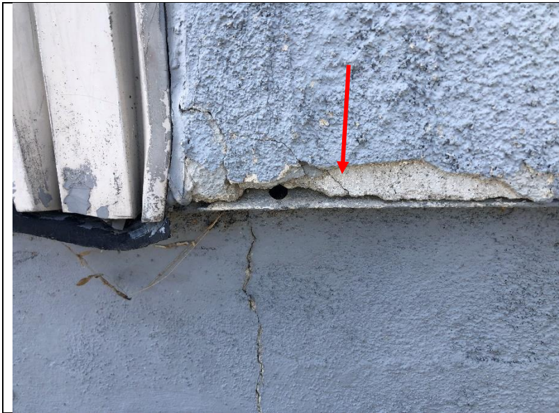
Photo 25: Deficiencies in the cement plaster were observed at the base of the walls
