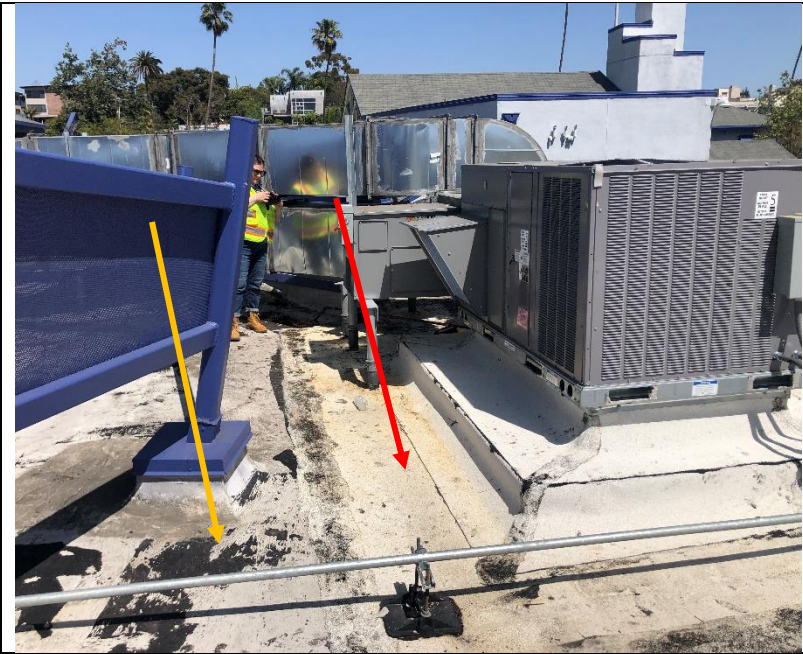
Photo 132: The existing BUR with a coating (yellow arrow) and the new granulated cap sheet (red arrow) were installed at the new mechanical curbs.
