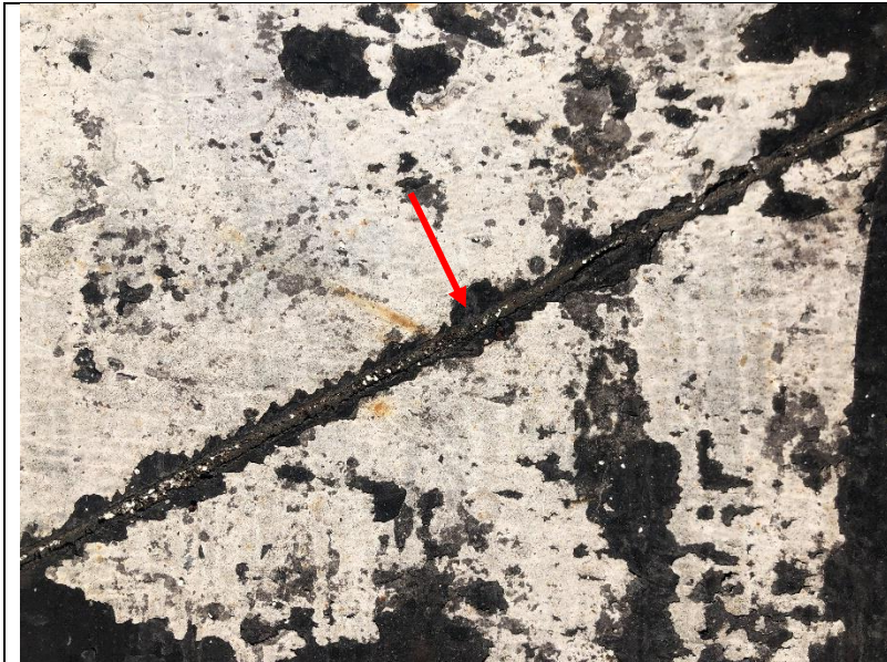
Photo 130: A cut mark in the BUR roof over the multipurpose room.
