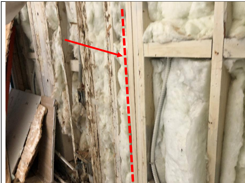
Photo 254: Delineation of damaged (left of dashed line) and undamaged areas on the south wall of room 415.
