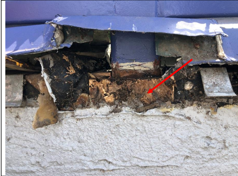
Photo 343: Wood rot and deteriorated wood materials were observed under the coping cap at the handrail curbs.
