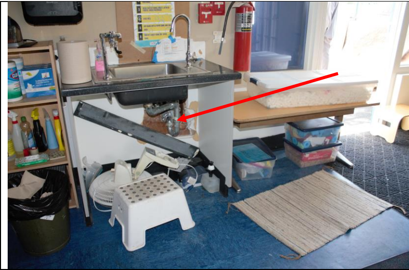
Photo 211: Interior finishes had been removed at two classrooms in building D prior to the DTR site assessment, in an effort to address a leak at this location.
