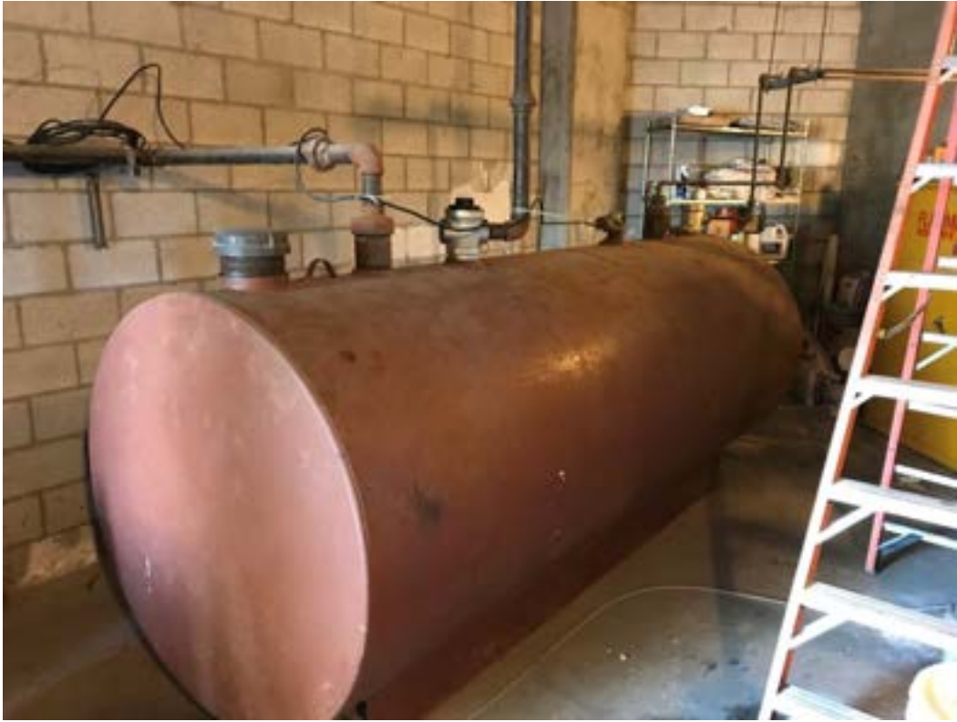
PHOTO 13: Diesel AST for hotel emergency generator
