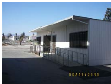
Construction progress photos of completed construction work on Relocatables Project
