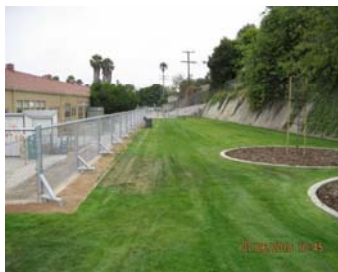
Photos of completed work on Landscape Improvements Project
