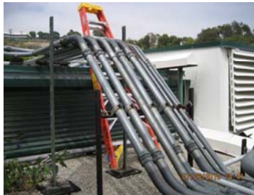
Construction progress photos at Webster ES Fire Alarm Replacement Project
