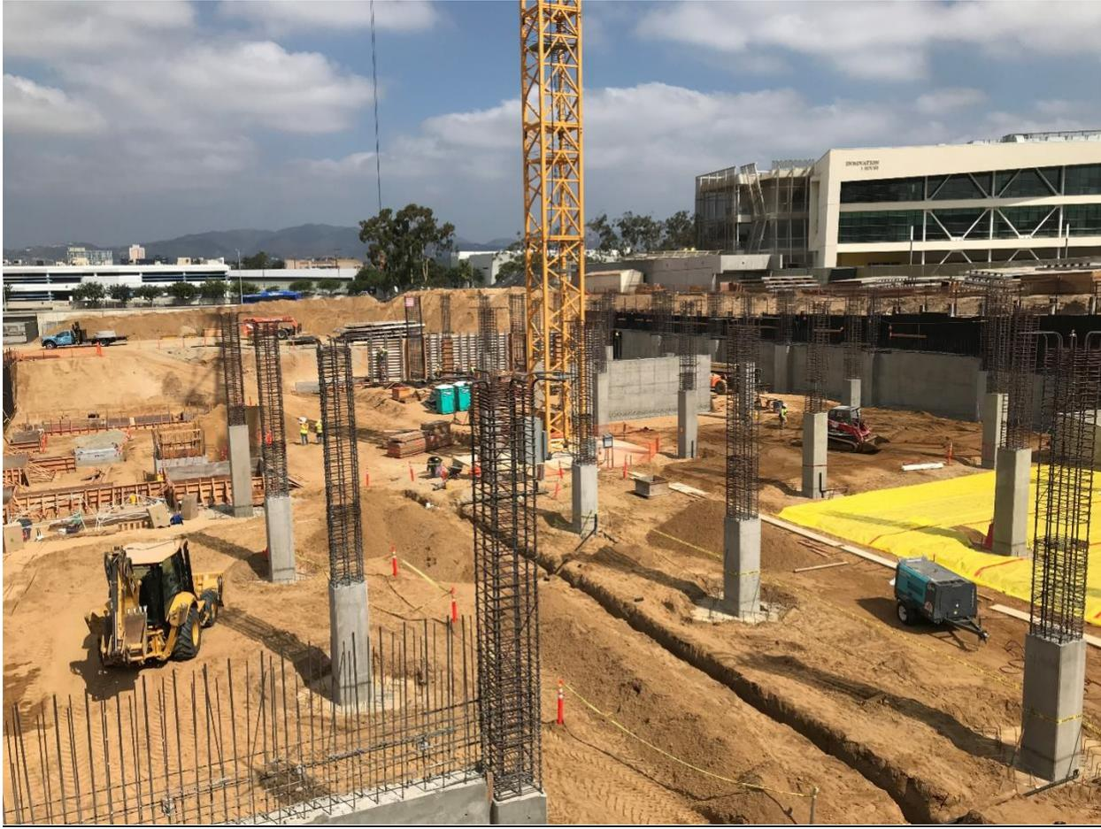
**Bases are complete for three of four quadrants. The wall and columns for the second level of parking are now 50% complete and waterproofing for the floor slab is installed.**
